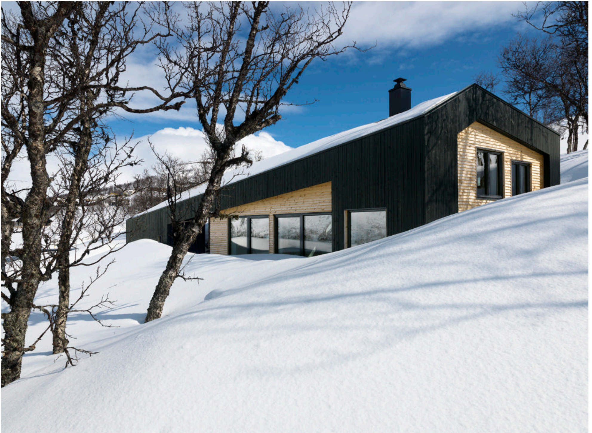
The Tyin Cabin is nestled into a slope, allowing drifting snow to partially cover the structure for added insulation. High environmental performance was a fundamental part of the client's brief.
