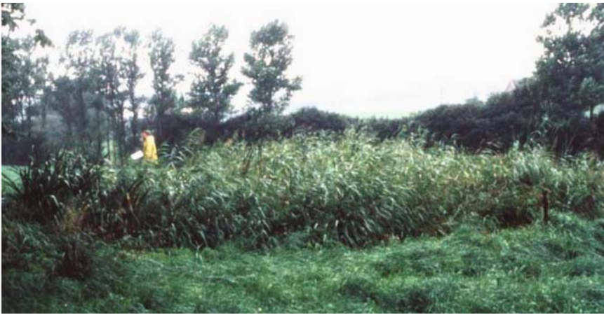
Figure 7-10. HF constructed wetland Ingstrup, Denmark (100 m 2 ) built in 1984 to treat sewage and dairy farm wastewaters. Photo by Hans Brix, with permission.
