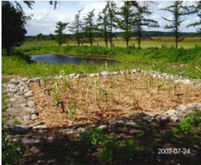
Figure 4-43. A single bed VF constructed wetland ( 15 \text{ m}^2 ) at Mørke, Denmark, planted with Phragmites australis . Left: shortly after planting in 2002 (from Arias and Brix, 2005a, with permission from Backhuys Publishers), Right: in June 2005, photo by Jan Vymazal.
