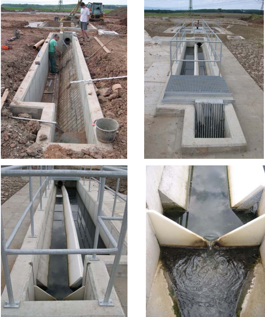
Figure. 5-12. Horizontal flow grit removal chamber in CW Libnič, Czech Republic. Top left: during the construction, note the depth of a sludge compartment, top right: grit chamber with screen bars after completion, bottom left: the view from the outflow side with the triangle trough in the left, bottom right: detail of the weir. Photos by Lenka Kröpfelová.
