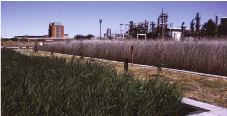
Figure 6-2. HF constructed wetland at Estarreja, Portugal treating wastewaters from nitric acid production. Photo by Jan Vymazal.
