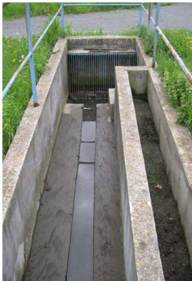
Figure 5-10. Left: grit chamber after the bar screens (CW Slavošovice, Czech Republic, photo by Lenka Kröpfelová), right: grit chamber preceding the screens (CW Kámen, Czech Republic, photo by Jan Vymazal).
