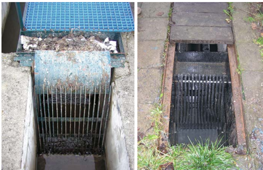
Figure 5-8. Manually-cleaned bar screens with dewatering plate on top of the screen, left: CW Slavošovice, right: CW Malhotice, Czech Republic. Photos by Lenka Kröpfelová.
