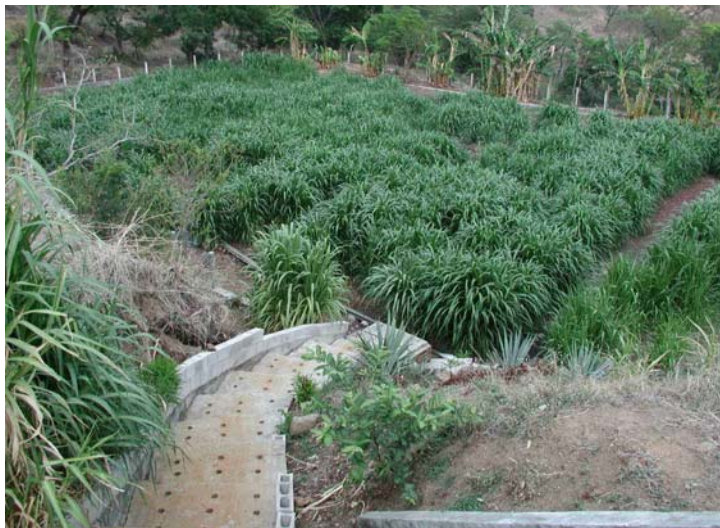
Figure 7-41. HF constructed wetlands “San José las Flores” at Chalatenango, El Salvador. Photo by Michael Platzer, with permission.
