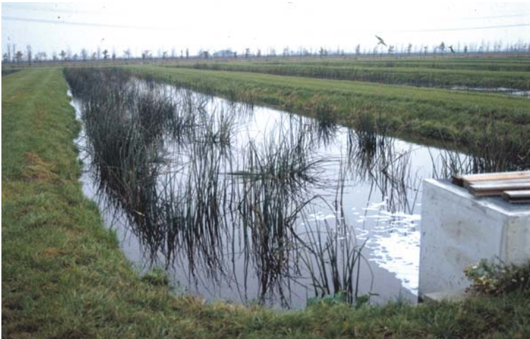
Figure 4-22. FWS constructed wetland at Lelystad, the Netherlands, planted with Scirpus lacustris . Photo by Hans Brix, with permission.
