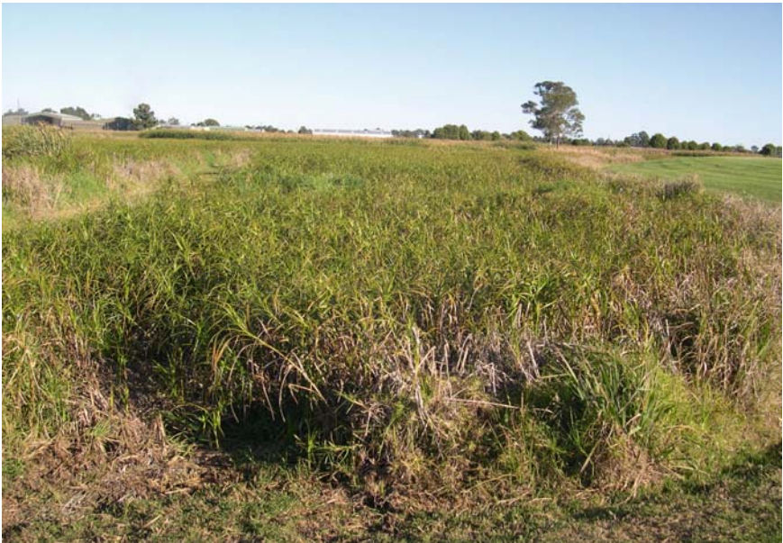
Figure 4-24. A 3-ha FWS constructed wetland for tertiary treatment of municipal sewage in Casino, NSW, Australia, planted with Bolboschoenus fluviatilis (picture) and Typha spp. Photo by Jan Vymazal.
