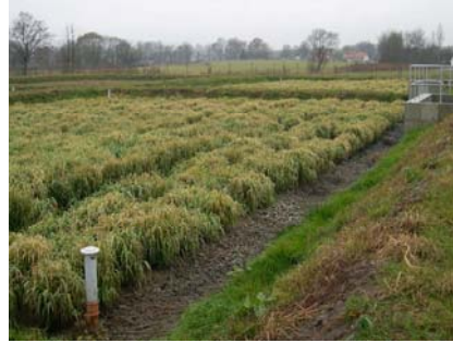
Figure 5-26. Distribution pipe buried on the bottom of the distribution zone. HF CW Čejkovice, Czech Republic. Left: construction of the inflow zone, right: Inflow zone after completion and in operation. Photos by Jan Vymazal.
