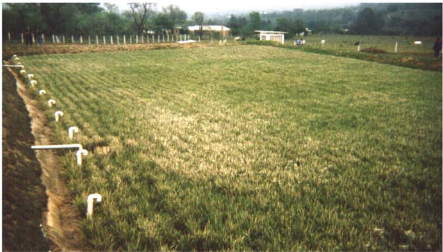
Figure 4-48. VF upflow constructed wetlands planted with rice ( Oryza sativa ) near Piracicaba, Brazil. Photos by Jan Vymazal.
