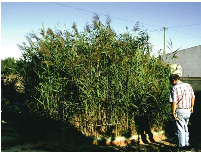
Figure 7-20. On-site HF constructed wetland at Malhão da Corcha near Odemira, Portugal planted with Phragmites australis (4 PE, 15 m 2 ). Photo by Jan Vymazal.
