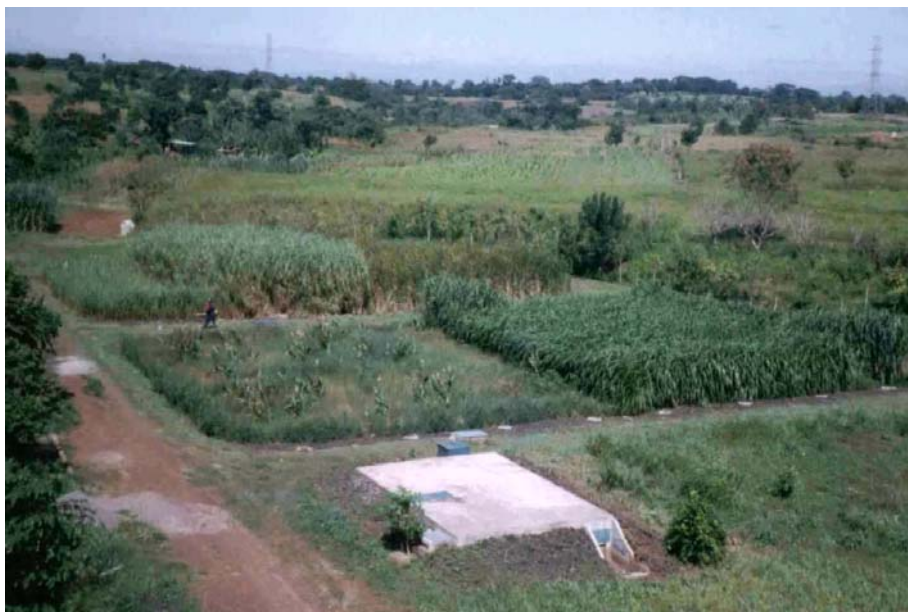
Figure 7-44. HF constructed wetland “Villa Bosco Monge” in Masaya, Nicaragua. Total area of the beds is 1,280 m 2 . Volcanic gravel (0.5-15 mm) is used as filtration substrate and beds are planted with Phragmites australis , Typha domingensis , Cyperus articulatus and Pennisetum purpureum . Photo by Michael Platzer, with permission.
