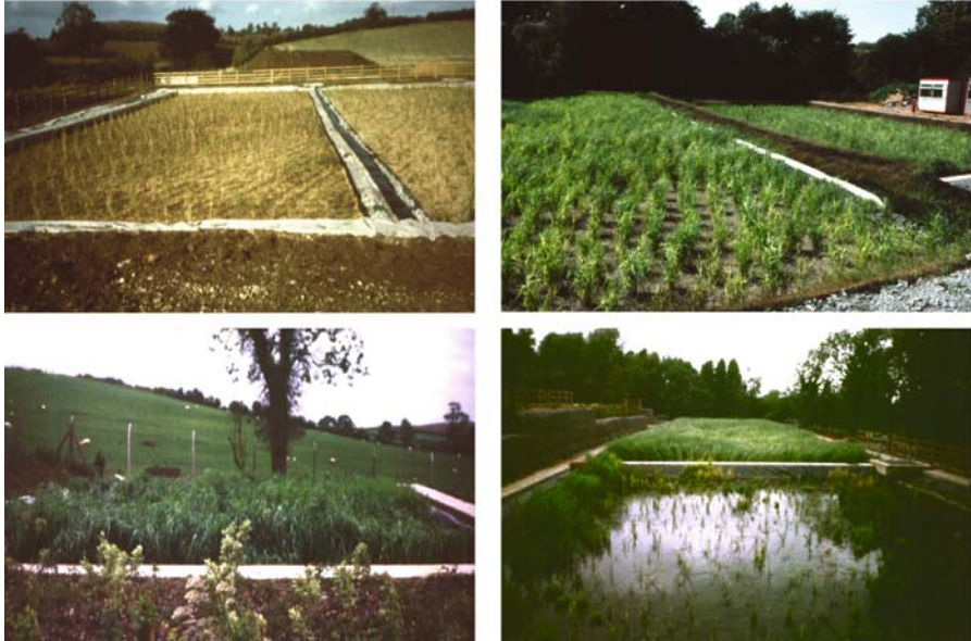
Figure 7-29. Examples of tertiary (a-c) and storm sewage overflow (d) HF constructed wetlands in the United Kingdom. Top left (a): Ashby Folville; Top right (b): Himley (Photos by Paul Cooper, with permission); Bottom left (c): Wormleighton; Bottom right (d): Leighthorne Heath – the front bed is flooded in order to protect newly planted Phragmites from rabbits; (Photos by Jan Vymazal).
