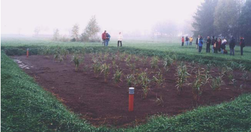
Figure 7-13. HF bed as a part of a hybrid system in Paistu, Estonia. Photo by Jan Vymazal.
