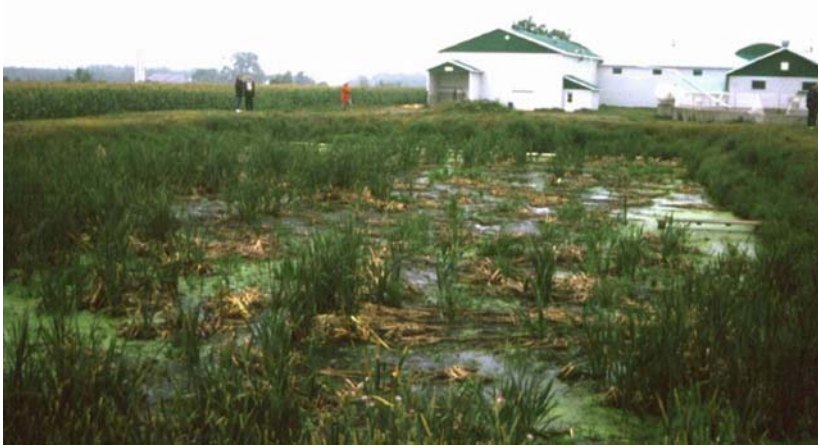
Figure 4-35. FWS constructed wetlands for abattoir wastewater treatment at Pouliot, Québec, Canada. Photo by Jan Vymazal.
