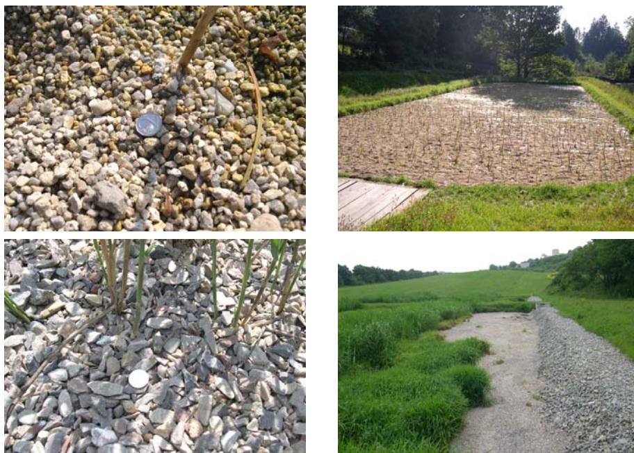
Figure 5-19. Washed gravel 4-8 mm in CW Sedlce, Czech Republic (top) and crushed rock 16-32 mm in CW Mořina, Czech Republic (bottom). As a scale, coin with a 20 mm diameter is used. Photos by Lenka Kröpfelová and Jan Vymazal.
