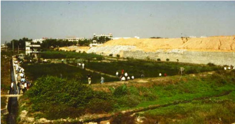
Figure 7-52. Constructed wetland at Bainikeng, Longgang, Shenzhen Special Economic Zone, China. The system consists of three HF compartments with a total area of 6,100 m 2 treating 1450 m 3 d -1 . Photo by Jan Vymazal.
