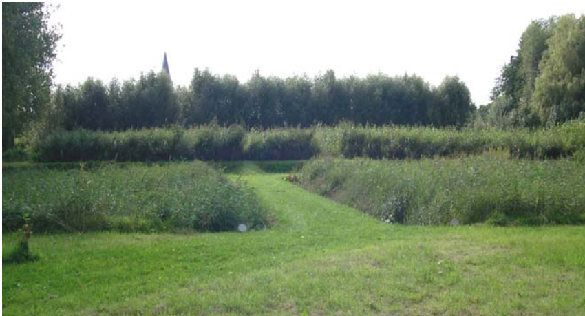
Figure 4-49. VF-HF constructed wetland (2,250 m 2 ) at De Pinte-Zevergem, Belgium planted with Phragmites australis . Photo by Lenka Kröpfelová.
