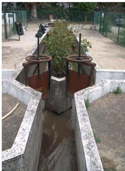
Figure 5-11. Two-chamber grit removal unit. Left: CW Ostrolovský Újezd, Czech Republic, no flow regulation; right: CW Beja, Portugal with adjustable baffles enabling the flow direction to one or both channels. Photos by Lenka Kröpfelová.
