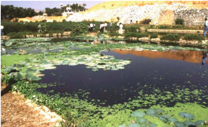
Figure 4-13. Constructed wetland in Bainikeng in south China. The pond planted with Nelumbo nucifera Gearth is the third stage of a hybrid constructed wetland. Photo by Jan Vymazal.
