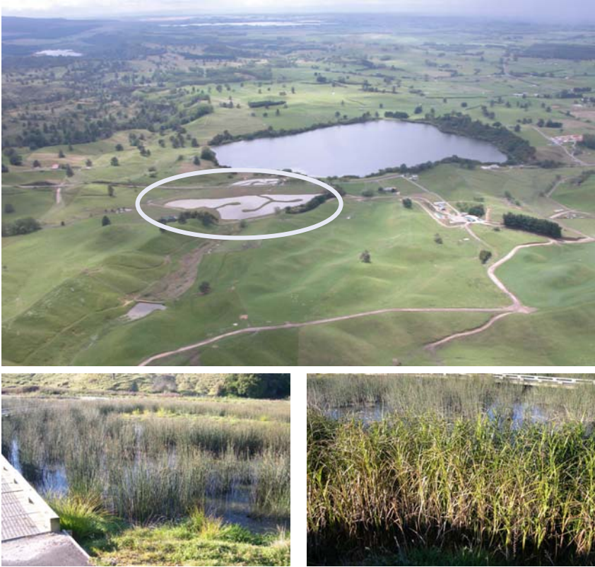
Figure 4-28. FWS constructed wetland (2.3 ha, in a white circle) treating runoff waters from 40 ha pasture catchment before discharging into Lake Okaro, New Zealand. Top - general view after construction, photo provided by Environment Bay of Plenty, New Zealand, bottom: details of vegetation: Scirpus tabernaemontani (left) and Bolboschoenus fluviatilis (right). Photo Jan Vymazal.
