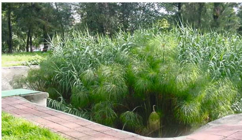
Figure 7-34. HF constructed wetland in the Mexico City park “Viveros de Coyoacán” for the treatment of highly polluted Magdalena River. Photo by Carmen Durán-de-Bazúa, with permission.
