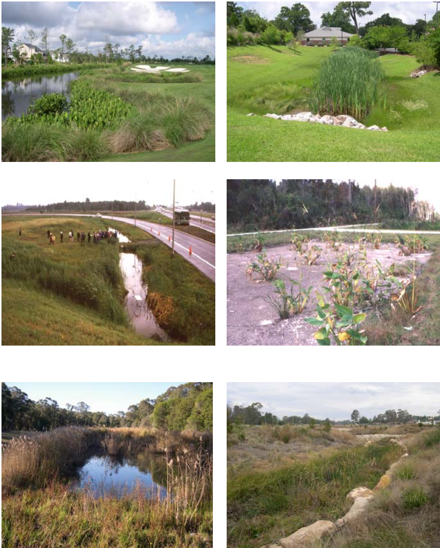
Figure 4-27. FWC constructed wetlands for golfcourse runoff in Rivertowne, South Carolina, USA (top left, dominant plant Sagittaria latifolia ), parking lot runoff in Charleston, South Carolina (top right, Typha latifolia ), highway intersection runoff in Boucherville near Montréal, Québec, Canada (middle left, Phragmites australis ), highway runoff in West Palm Beach, Florida, USA (middle right, Thalia geniculata ), stormwater runoff from residential area in Plumpton Park, NSW, Australia (bottom left, Phragmites australis ) and in Bonnyrigg Park, Fairfield, NWS, Australia (bottom right, Typha spp. Baumea articulata ). Photos by Jan Vymazal.
