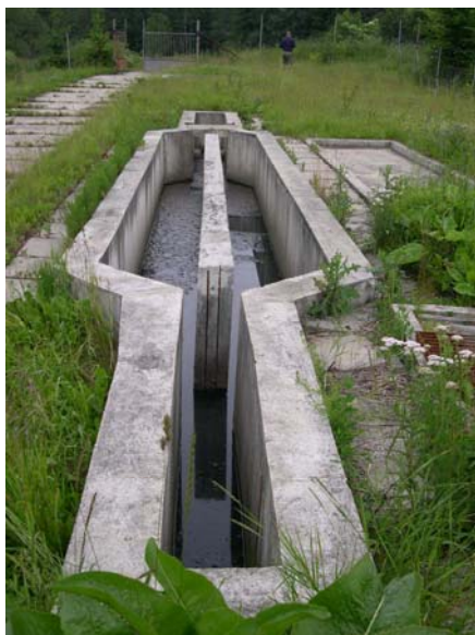
Figure 5-11. Two-chamber grit removal unit. Left: CW Ostrolovský Újezd, Czech Republic, no flow regulation; right: CW Beja, Portugal with adjustable baffles enabling the flow direction to one or both channels. Photos by Lenka Kröpfelová.
