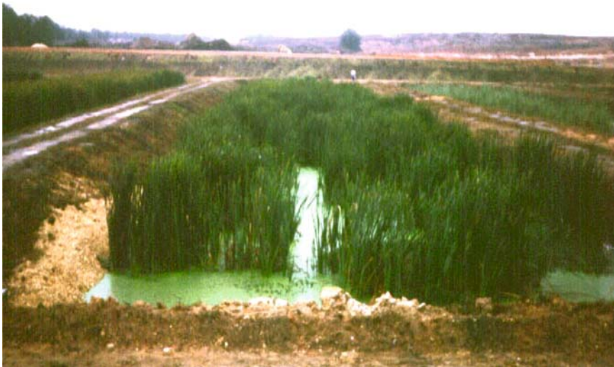
Figure 4-34. FWS constructed wetland for municipal landfill leachate at the Perdido Landfill near Pensacola, Florida. Detail of one out of 10 cells (91 x 11 m each) connected in series. For details on performance see DeBusk (1999) or Martin and Moshiri (1992). Photo by Jan Vymazal.
