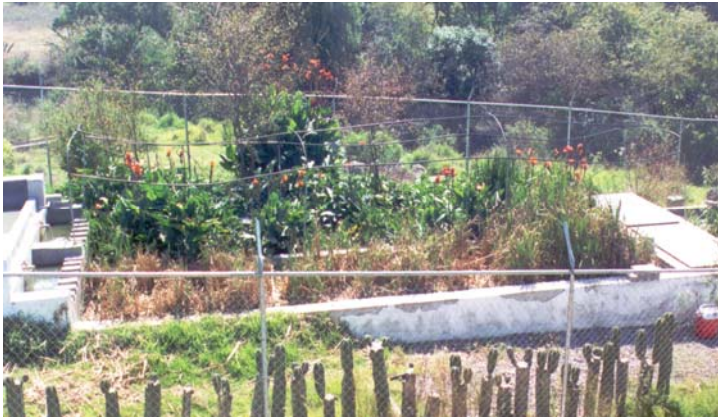
Figure 7-33. HF constructed wetland as part of the hybrid system at Santa Maria Nativitas in central Mexico. Photo by Marco Belmont, with permission.
