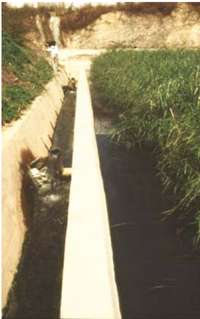
Figure 5-36. Wide outflow zones may be equipped with a series of outflow structures in order to provide an even discharge along the outflow zone. Left: Yaintian, China, right: Piracicaba, Brazil. Photos by Jan Vymazal.
