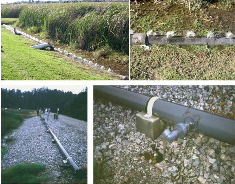
Figure 4-19. Examples of water distribution at the inflow of FWS constructed wetlands. Top: Casino, NSW, Australia; bottom: Pensacola, Florida, USA. Photos by Jan Vymazal.
