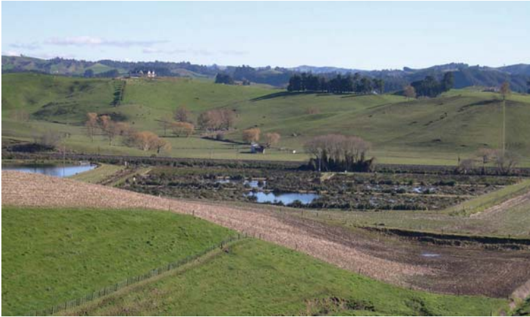
Figure 4-54. A 3 ha tertiary FWS-HF constructed wetland at Otorohanga, New Zealand. FWS part in front is planted with Eleocharis sphacelata and Scirpus tubernaemontani , HF part in the back is planted with Baumea articulata and Carex secta . Photo by Jan Vymazal.
