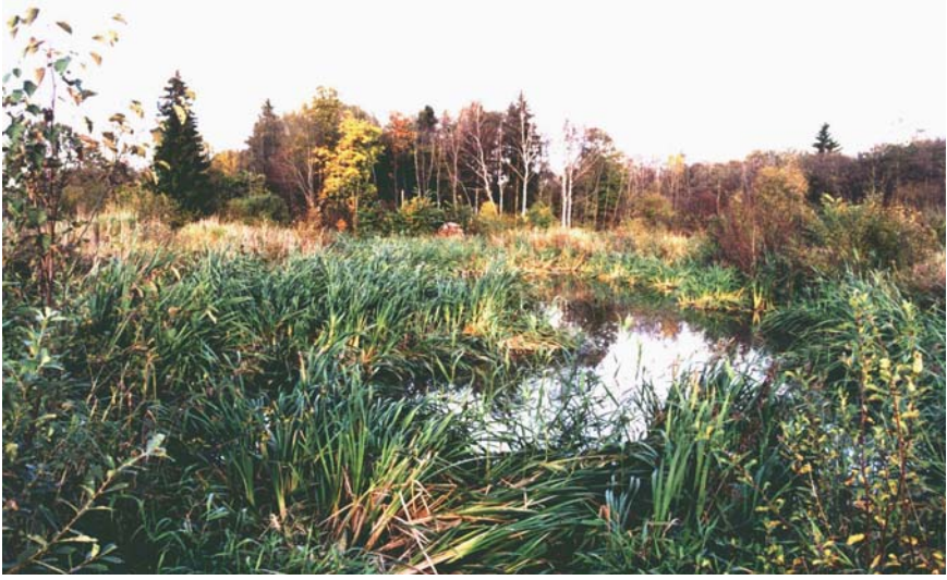
Figure 4-23. FWS constructed wetland for tertiary treatment of municipal sewage in Põltsamaa, Estonia planted with Typha latifolia . Photo by Jan Vymazal.
