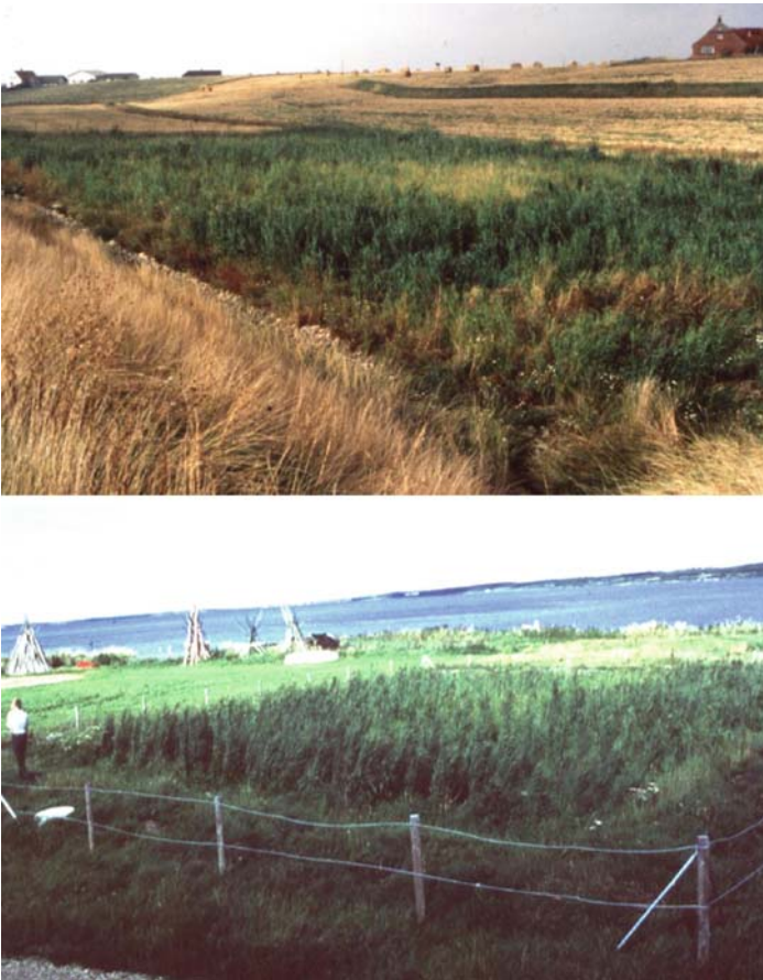
Figure 5-2. Two of the first HF constructed wetlands built in Denmark in 1984: top: Ferring ( 2,000\text{ m}^2 , 500 PE), bottom: Knudby ( 418\text{ m}^2 , 65 PE). Photos by Hans Brix, with permission.
