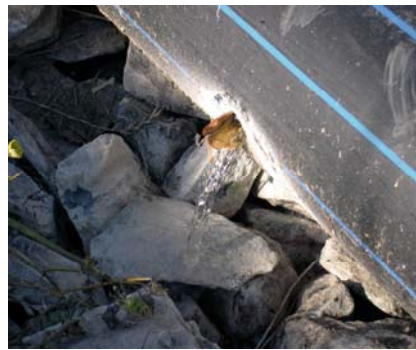
Figure 5-27. Distribution pipes on the surface of distribution zone. HF CW Čehovice, Czech Republic. Left: general view, right: detail of the wastewater inflow. Photos by Lenka Kröpfelová.
