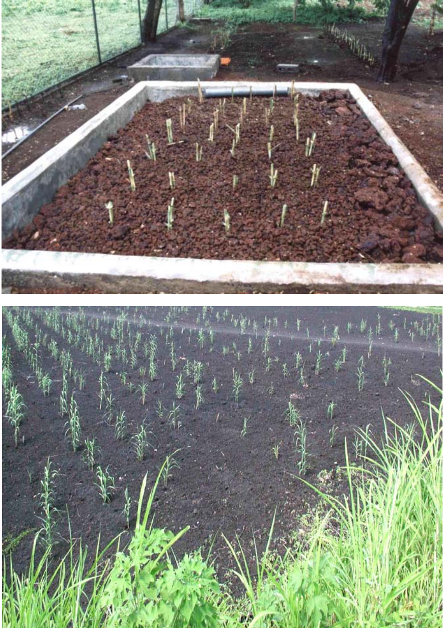
Figure 7-45. HF constructed wetlands “Carretera Sur” at Managua, Nicaragua (5 PE, 7 m 2 ) planted with Phalaris arundinacea (top) and “Chicigalpa” at Chinandega, Nicaragua (8,750 PE, 10,000 m 2 ) planted with Phragmites australis (bottom). Photos by Michael Platzer, with permission.
