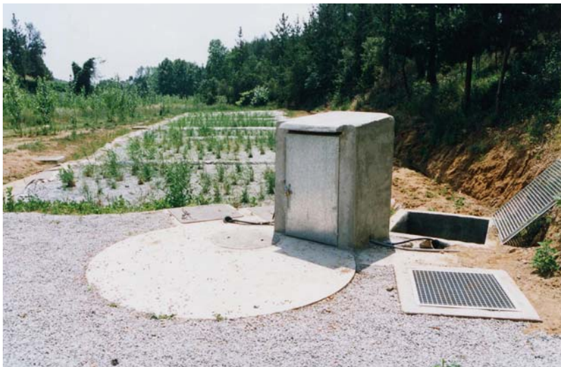
Figure 7-25. HF constructed wetland at Les Franqueses, Spain, treating wastewaters from 100 PE in 8 parallel beds ( 54 \text{ m}^2 each). Photo by Joan García, with permission.
