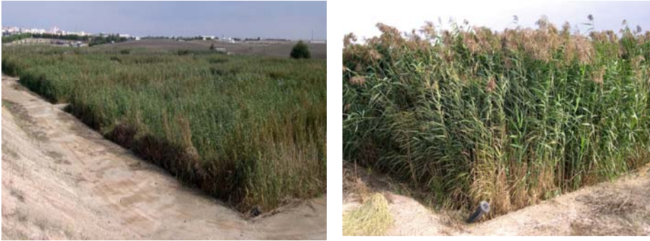
Figure 5-41. HF constructed wetland Beja, Portugal planted with Phragmites australis . Top: general view, bottom: detail on Phragmites stand. Photos by Jan Vymazal and Lenka Kröpfelová.
