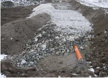
Figure 5-26. Distribution pipe buried on the bottom of the distribution zone. HF CW Čejkovice, Czech Republic. Left: construction of the inflow zone, right: Inflow zone after completion and in operation. Photos by Jan Vymazal.
