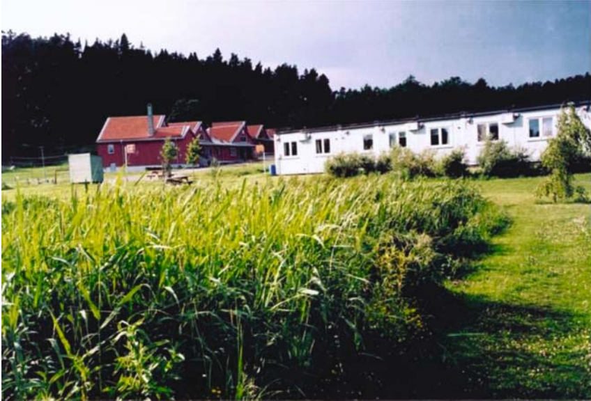
Figure 7-26. HF constructed wetland at Björkö-Ljungsbo for treatment of wastewater from a school with 250 children. Photo by Zdeňka Žáková, with permission.
