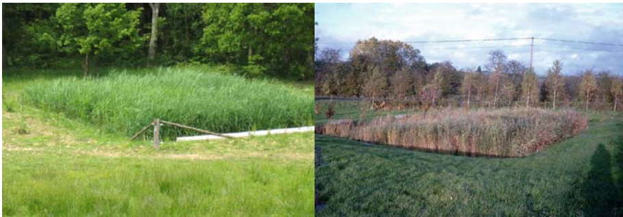
Figure 7-3. HF constructed wetlands Nassogne for 20 PE (left) and Sainte Ode for 40 PE (right) in the Walloon region of Belgium. Photo by Nathalie Fonder, with permission.
