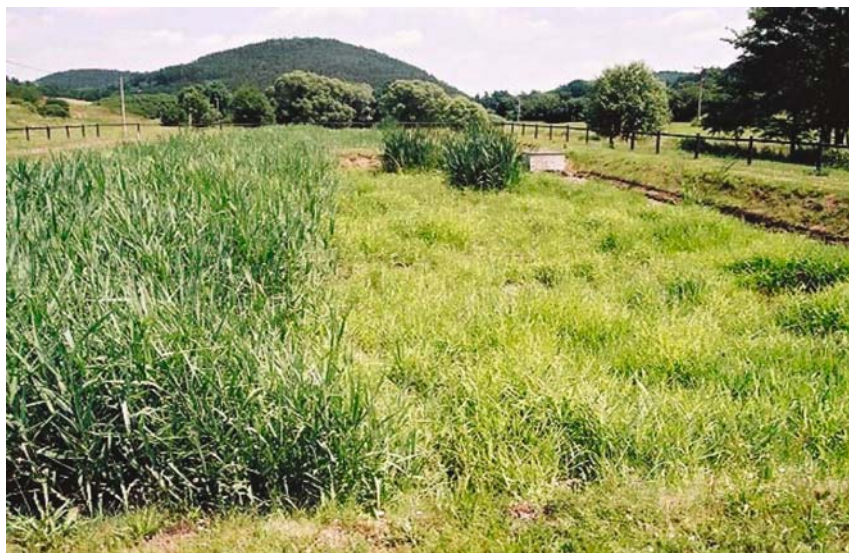
Figure 7-7. HF constructed wetland Čim planted with bands of Phragmites australis (left) and Phalaris arundinacea (right). Photo by Jan Vymazal.
