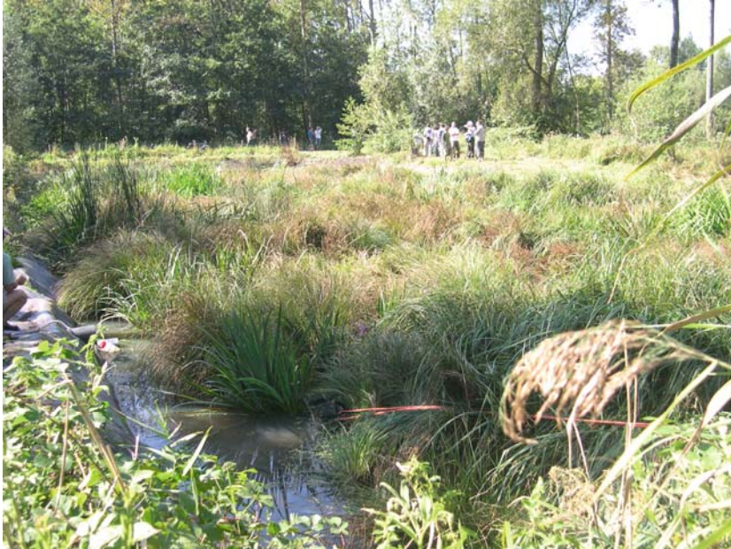
Figure 4-39. FWS constructed wetland with floating mats of emergent macrophytes (e.g., Sparganium , Juncus , Epilobium , Scirpus ) for treatment of combined sewer overflow in Bornerm, Belgium. Plants are kept upright using coconut string grid. Photo by Lenka Kröpfelová.
