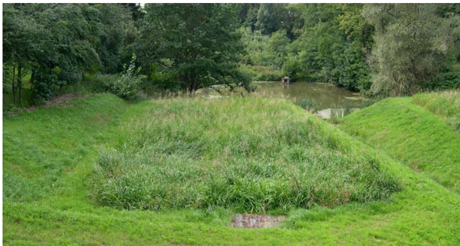
Figure 5-53. HF constructed wetland Sedlce, Czech Republic planted with Glyceria maxima . For detail see Fig. 5-51. Photo by Lenka Kröpfelová.
