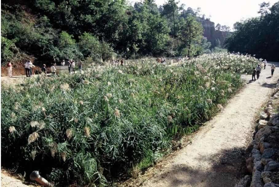
Figure 4-44. VF constructed wetlands treating raw sewage from 1,200 PE in Roussilon, France. Photo by Jan Vymazal.
