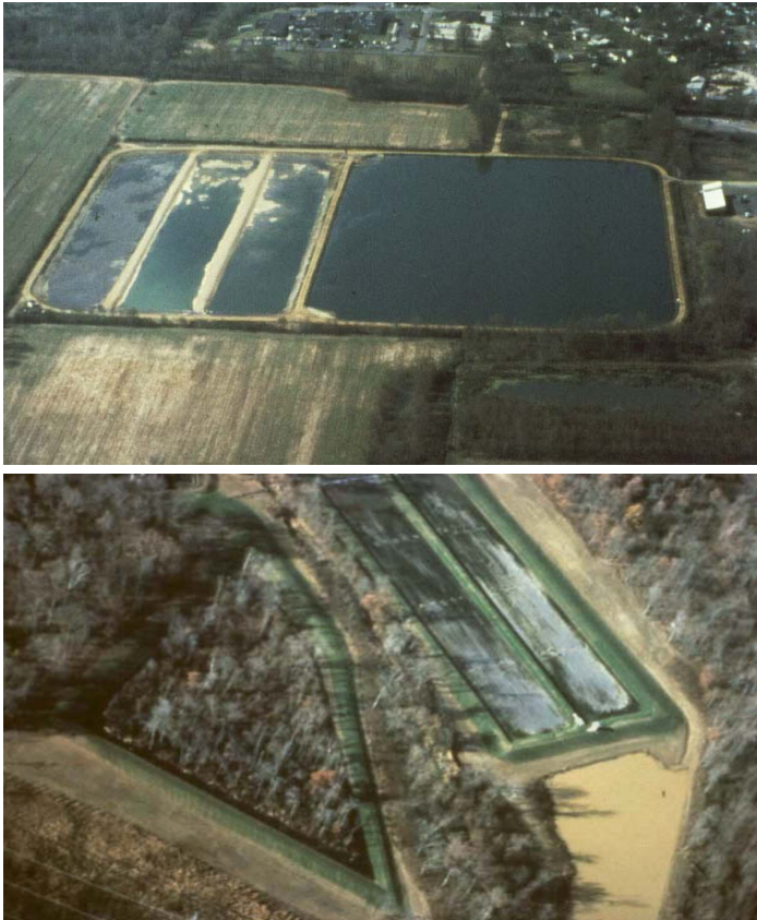
Figure 7-35. Tennessee Valley Authority demonstration HF constructed wetlands at Benton (top) and Hardin (bottom), Kentucky shortly after construction. Photo courtesy Jim Watson.
