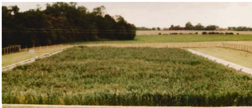
Figure 5-69. HF constructed wetland at Freethorpe, United Kingdom with one bed of 3,500 \text{m}^2 . Photo by Jan Vymazal.
