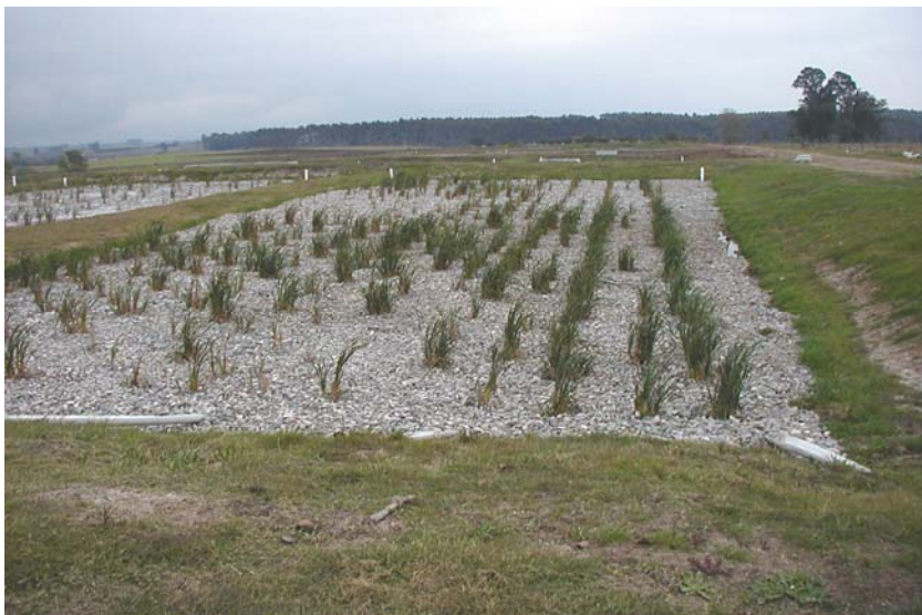
Figure 5-6. Newly-planted HF constructed wetland San Jacinto, Uruguay, treating wastewater from a meat processing facility shortly after plantation of Typha domingensis in 2006. Total area of four beds is 1.5 ha, average flow 3000 \text{ m}^3 \text{ d}^{-1} . Photo by Silvana Perdomo, with permission.
