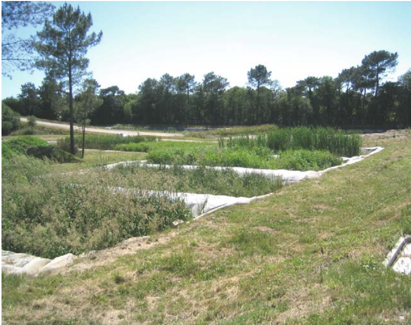
Figure 4-50. VF-HF hybrid constructed wetlands for composting plant leachate treatment in Bretagne, France. The 1 st VF stage (4 x 120 m 2 ) is planted with Phragmites australis , 2 nd VF stage (4 x 72 m 2 ) is planted with Typha latifolia , P. australis , Scirpus lacustris and Phalaris arundinacea in each bed and 3 rd HF stage (2 x 290 m 2 ) is planted with Carex acuta , Iris pseudacorus , Acorus calamus , S. lacustris , Juncus effusus , Mentha aquatica and Sparganium erectum . From Reeb and Werckmann (2005) with permission from Backhuys Publishers.
