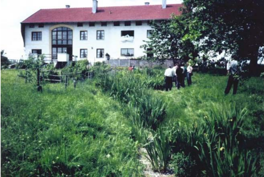
Figure 7-14. HF constructed wetland at Gasteig, Germany built in 1986. Photo by Zdeňka Žáková, with permission.
