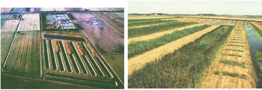
Figure 4-17. Constructed wetland Eversteekoog on the island of Texel, The Netherlands. From the right, ditches 1, 3, 5 and 7 are planted with Phragmites , ditches 2, 4, 6 and 8 are planted with Typha (at the time after a harvest). The second half of the ditches contains submerged macrophytes. Photos by Ruud Kampf, with permission.
