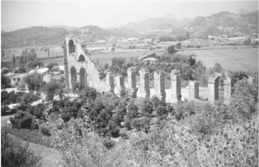
FIGURE 1.39 Remnants of triple siphon at Aspendos, Turkey. The wide valley is illustrated with the south tower in the foreground and the north tower in the distance. Open tanks were located at the top of each of the two towers, commonly referred to as pressure towers in the literature. (Photo by Koksal B. Celik)
