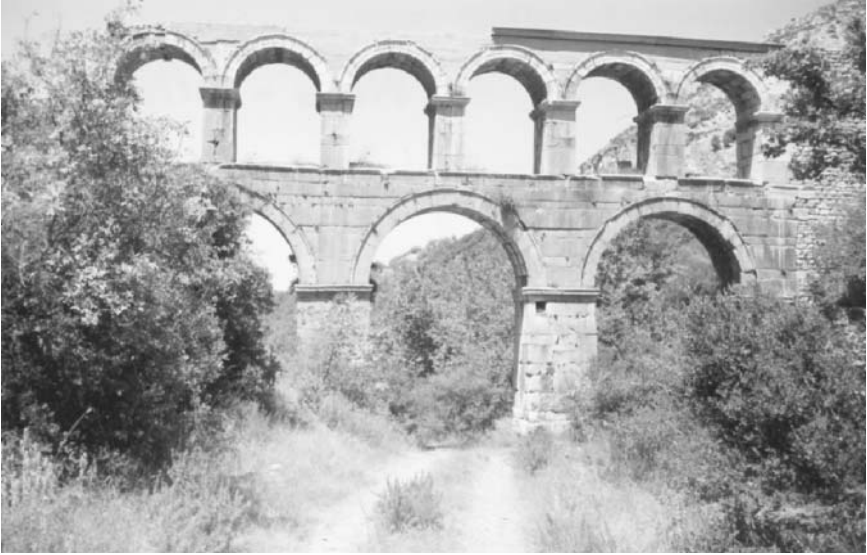
FIGURE 1.35 Bridge (16 m high) of the aqueduct Sextilius-Pollio of the Derbentdere system to Ephesus. This is part of the Marnas conveyance system to Ephesus built around A.D. 4–14. (Photo by Koksal B. Celik)
