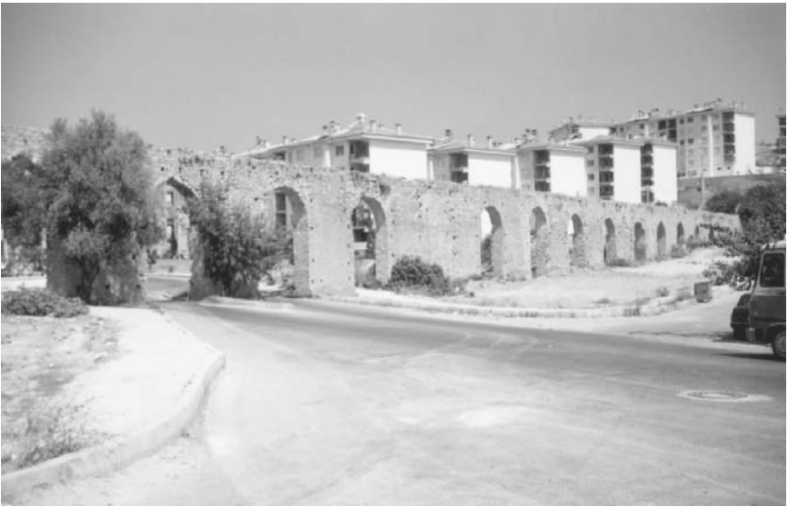
FIGURE 1.36 Aqueduct of the Degirmendere system to Ephesus located in Kusadasi, Turkey. (Photo by Koksal B. Celik)
