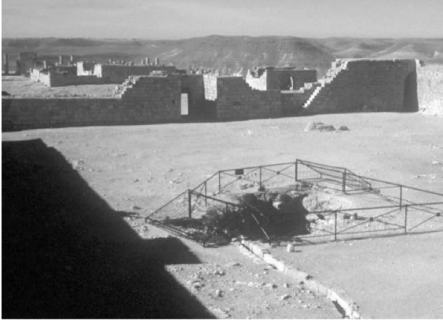
FIGURE 17.5 The acropolis of the ancient Nabatean-Byzantine city of Avdat is situated on a flat hilltop in the central Negev Desert. A conduit enters the acropolis from outside the city walls. It used to channel runoff water from a natural catchment into the main cistern on the acropolis. (Photograph H. J. Bruins)
