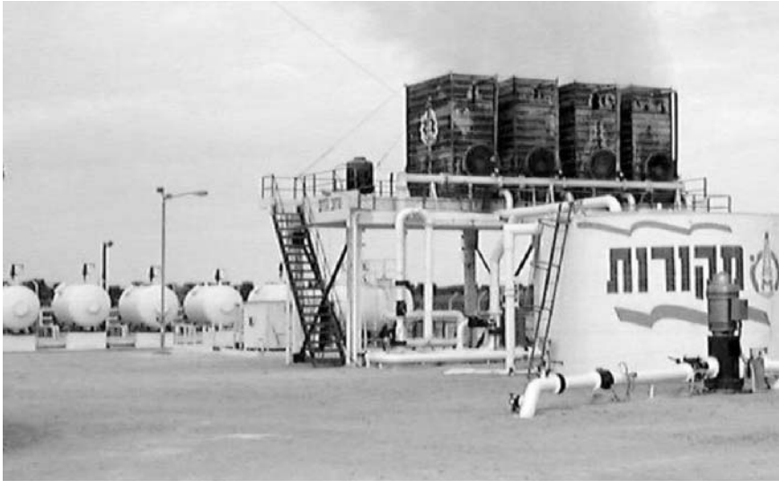
FIGURE 17.9 Pumping of (warm) groundwater in the Arava Rift Valley from a depth of 1500 m. (Photograph H. J. Bruins)
