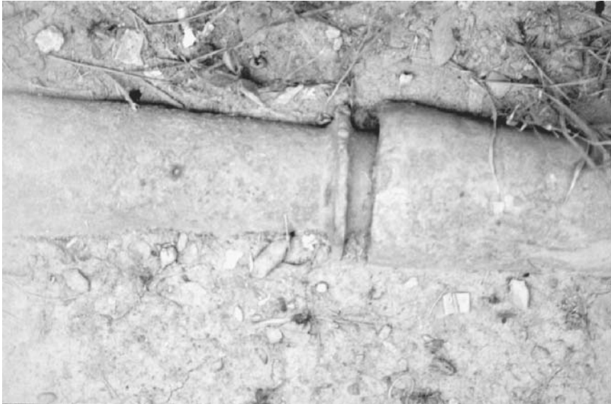
FIGURE 1.8 Water distribution pipe in Knossos, Crete, built around 2000 B.C. by the Minoans. (Photo by Larry W. Mays and copyright by Larry W. Mays)
