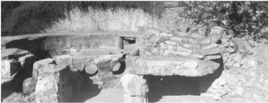
FIGURE 1.47 Views of the castellum divisorium at Nîmes. Water enters the circular basin through the rectangular aqueduct opening. Refer to Fig. 1.48 for the plan view with dimensions. (a) Shows 6 of the 10 openings for lead pipes used to distribute the water, and (b) shows a different view illustrating two of the openings. (Photos by Larry W. Mays and copyright by Larry W. Mays)
