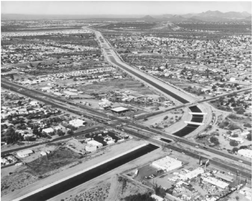
FIGURE 1.6 Central Arizona Project (CAP) aqueduct through a residential area in Scottsdale, Arizona. (Courtesy of Central Arizona Project)
