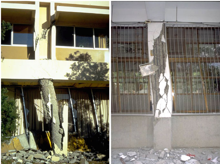
Fig. 17.1 Examples of buildings with residual displacements that lead to their demolition (Photos courtesy of NISEE, UC Berkeley)
