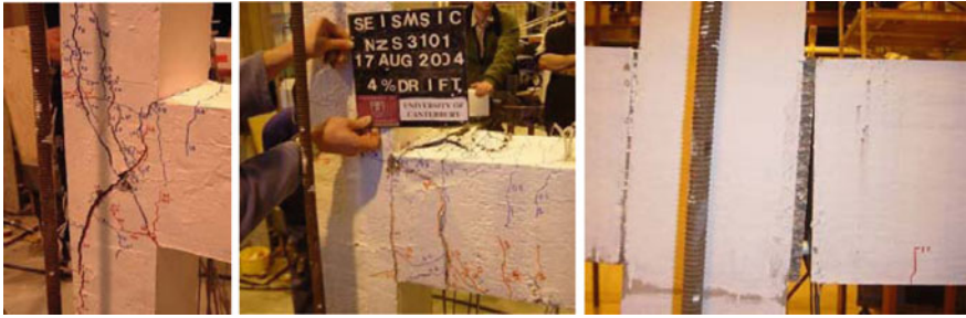
Fig. 28.2 Evolution of seismic resisting connections: experimental performance of beam-column joints designed according to Left : pre-1970 codes (shear damage in the joint); Centre : capacity design principles as per the NZS3101:1995 (beam plastic hinge) and Right : hybrid jointed ductile connections as per NZS3101:2006, Appendix B (controlled rocking) [14]
