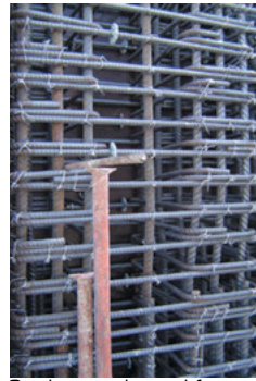
Setting up plywood formwork
