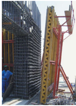
Setting up formwork
