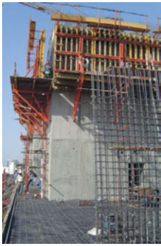
Moving formwork up to higher floors
