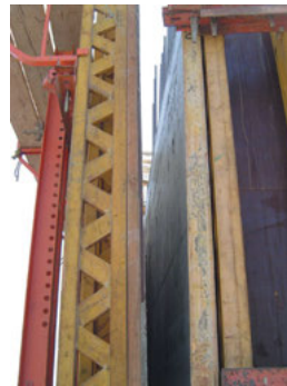
Setting up formwork
