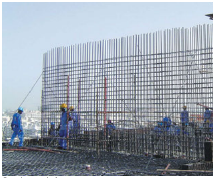
Setting reinforcement
