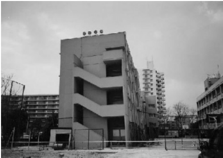
Photo 6.1. Settled school houses in Kobe
