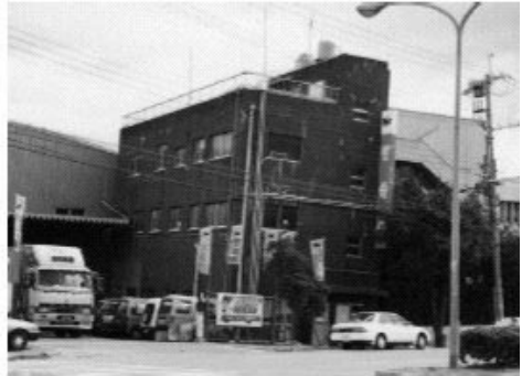
Photo 11.2. Tilted building in liquefied level ground
