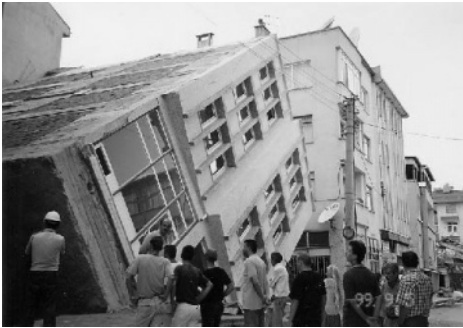
Photo 6.3. A settled building at Site 16 and S4 in Adapazari
