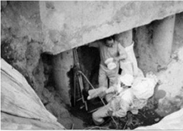
Photo 11.5. Borehole camera survey followed by excavation
