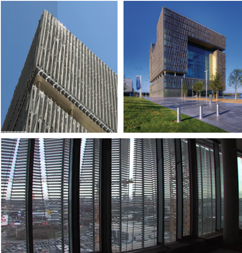
FIGURE 4.7 Changing daylight levels in Q1 (top), Facades of Q1 (bottom).
