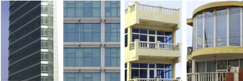
FIGURE 16.64 Large glazing areas should be avoided in the façades' typologies, as they are largely responsible for the overheating of the building, and subsequent use of energivorous air conditioning systems. The sealed façades with large areas of glazing are an imported typology, inadequate in the hot climates (Luanda, Angola; Praia, Cape Verde).
