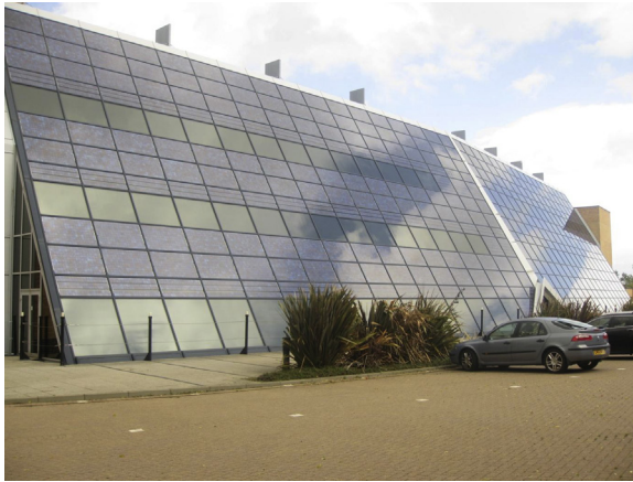
FIGURE 4.3 The Integrated PV array on the South Façade of the Doxford Solar Building. Photo courtesy: the author.
