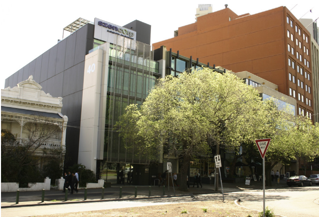
FIGURE 13.14 40 Albert Road South Melbourne, Victoria, Australia.
