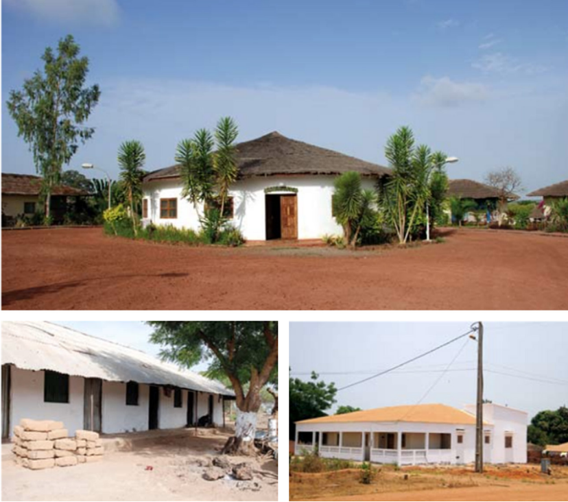
FIGURE 16.54 Buildings painted white, in Guinea-Bissau, to reduce the discomfort from overheating.
