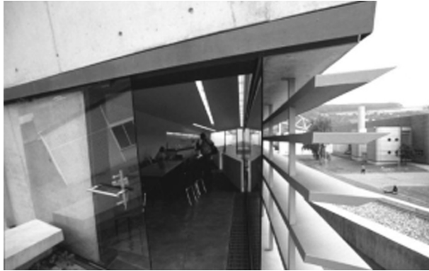
FIGURE 9.11 Fixed shading devices darken the room and artificial light is switched on: Vitra, fire station, Weil a.R., Germany, architect: Zaha M. Hadid.
