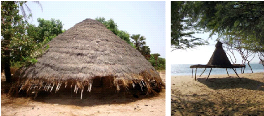
FIGURE 16.25 Shading is a centuries-old heat protection technique. Vernacular buildings in Guiné-Bissau (left) and Angola (right).
