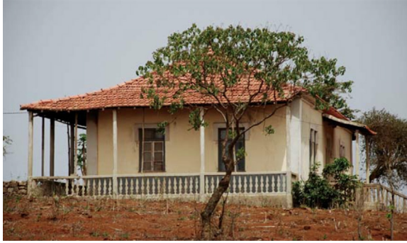
FIGURE 16.35 Examples of fixed shading in Cape Verde: 1. Projection of the roof to shade the façades, in the Amilcar Cabral house-museum; 2. Projection of the roof in institutional building; 3. Shading of esplanade in St. Antao, 4. Grid system for shading and ventilation in a building in Mindelo, 5. Vertical shading in a services' building in Praia.
