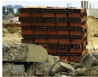
FIGURE 16.62 Left: Schematic representation of a radiant barrier on a roof, with ventilated air box. Right: the use of perforated brick may improve the building's insulation, though it should be further reinforced with external or cavity wall insulation materials.
