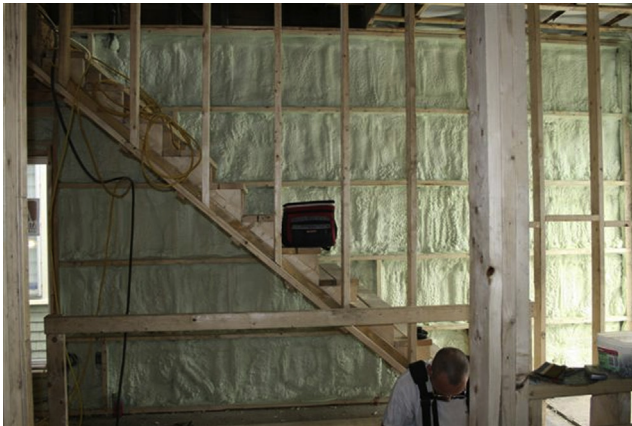
Cross bracing and interior insulation.
