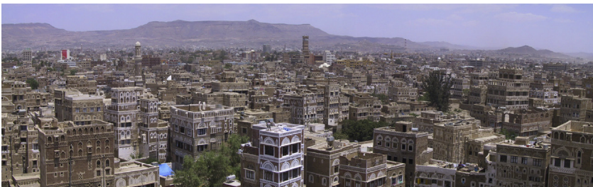
FIGURE 10.1 Panorama view of Sana'a. (Photograph by Daniel Pini, Courtesy of General Organization for the Preservation of Historic Cities of Yemen, GOPHCY)
