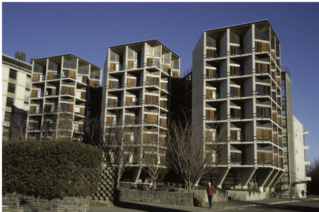
FIGURE 13.10 Erskine Building – north-east Façade.
