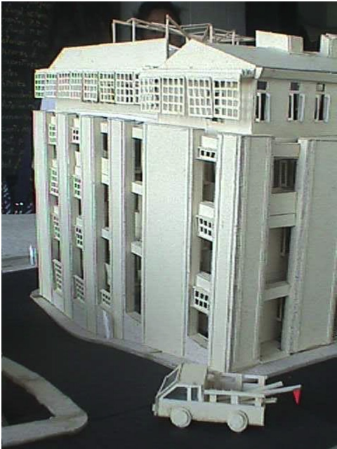
FIGURE 8.29 Model of the building, incorporating the preexisting wall as a double skin.
