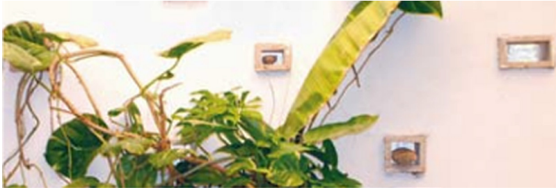
FIGURE 16.79 Vents with mosquito nets in a house in Mindelo.
