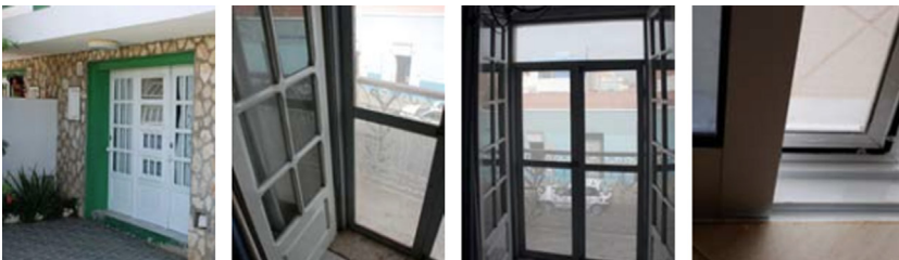
FIGURE 16.78 Windows protected by a mosquito net, in Praia.
