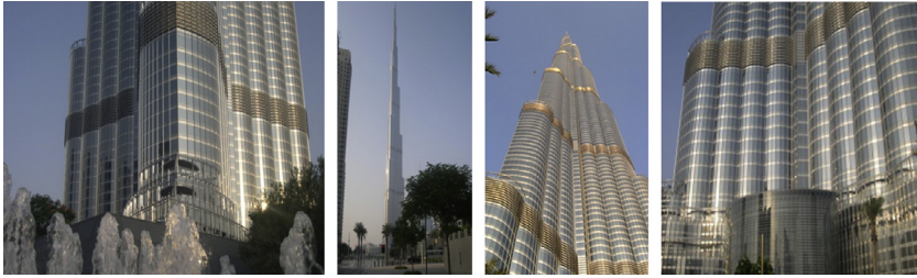
A view showing the massive area of facades glazing
