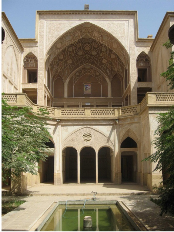
FIGURE 14.1 The courtyard and its elements provided a comfortable microclimate inside the house in a desert climate; Abbasian House, Kashan, Iran.
