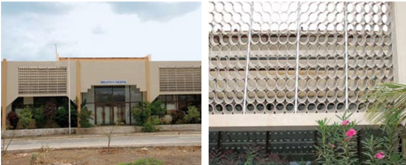
FIGURE 16.36 Fixed shading in Cape Verde: double façade shading system, in an institutional building in the city of Praia. The exterior façade shades the glass and opaque areas through the use of an ingenious grid system using overlapping tubes, allowing for natural light and ventilation.
