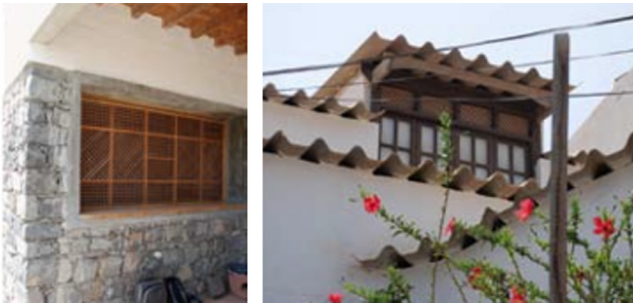
FIGURE 16.75 The use of fixed grids, although not allowing adjustments to control shading and the ventilation flow, can also be an effective solution in some cases.
