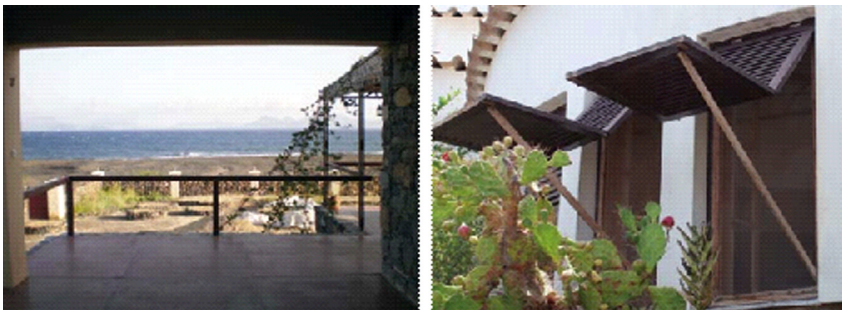
FIGURE 16.26 Left: a house with covered courtyard in Porto Novo. Right: Adjustable external shading in a house in Mindelo, Cape Verde.
