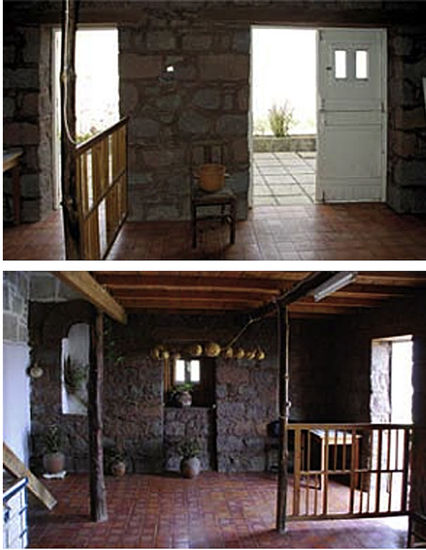
FIGURE 16.66 Rehabilitated vernacular house in Santo Antão. The window area is sufficient and adequate to meet the needs of natural lighting and ventilation.
