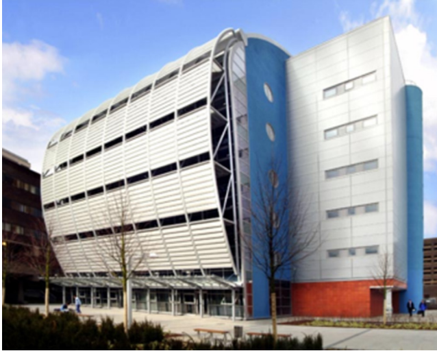
FIGURE 4.6 The Devonshire Building completely closed in response to a sunny day.
