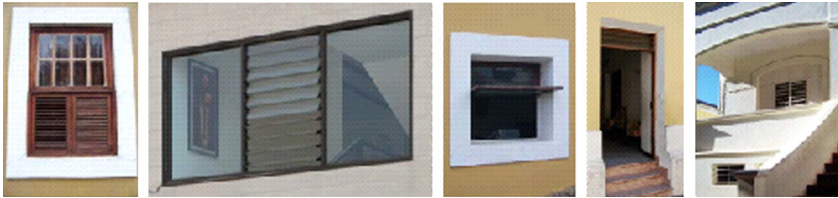
FIGURE 16.73 Maputo, Mozambique: adjustable devices for natural ventilation.
