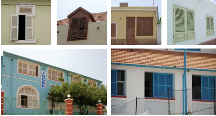
FIGURE 16.74 External shutters are a typology traditionally used in Cape Verde and Bissau. They provide window shading, and allow the control of the natural ventilation flow to the interior of the building.
