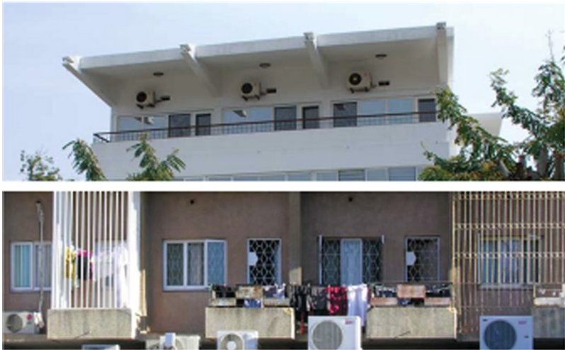
FIGURE 16.124 Use of air conditioning devices, city of Praia, Cape Verde.
