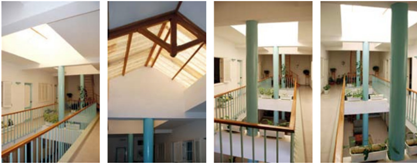
FIGURE 16.90 (1.4) Atrium inside a building in Praia promotes natural lighting and stack effect ventilation. In hot climates, the top of the atrium must be at least 5m above the occupied space, and it must have outlet air vents in order to prevent the accumulation of hot air.
