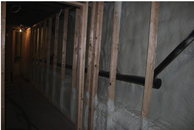
Interior insulation with stand-off wall in basement.
