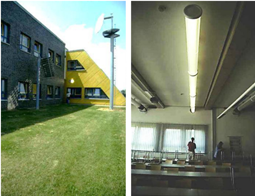
FIGURE 9.21 Heliostat and light tube at Solar Campus Juelich, Fachhochschule Aachen, Germany.
