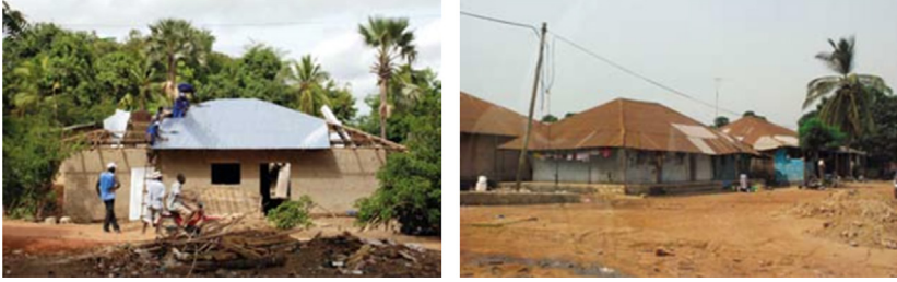
FIGURE 16.59 Guiné-Bissau: The use without protection (insulation) of metal roofing should be avoided, as it leads to situations of internal overheating. Furthermore, with the oxidation, the metal cover darkens, transmitting more heat to the internal spaces.
