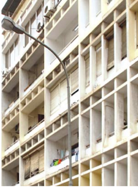
FIGURE 16.33 Fixed shading in the façades of modernist buildings in Luanda.
