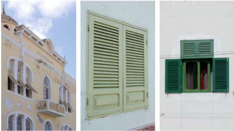
FIGURE 16.37 Adjustable external shading: wood shutters (venetian blinds) provide shade and simultaneously allow for natural lighting and ventilation. Right: Adjustable shading: leisure area in the fort museum, at the Cidade Velha. The shading strategy allows natural lighting and ventilation.
