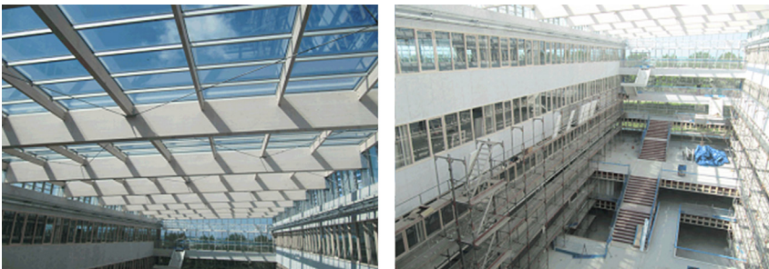
FIGURE 1.11 Roof and area of the atrium.
