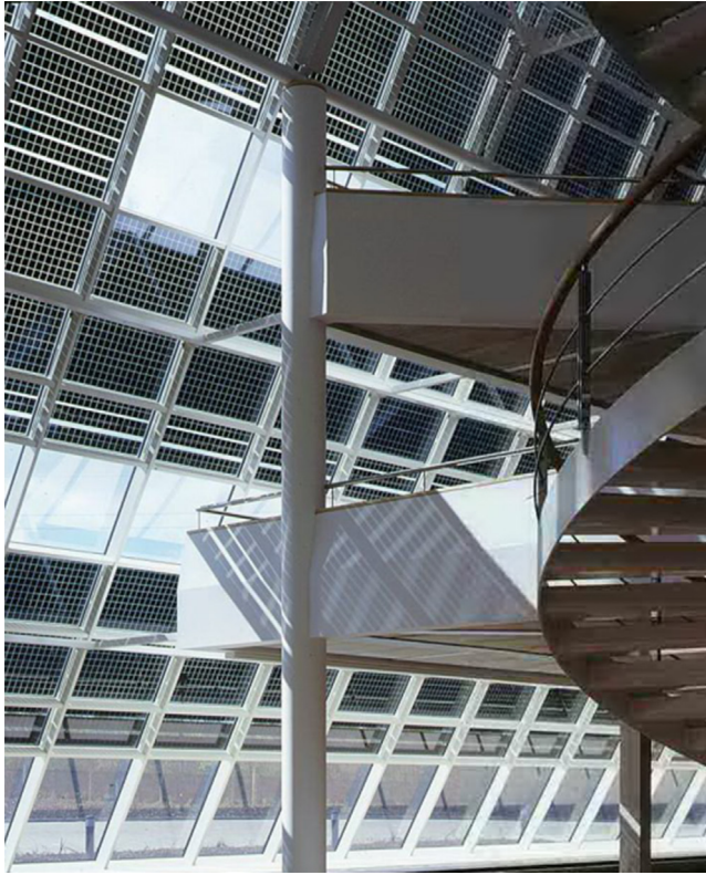
FIGURE 4.5 The interior of the building, with its varied shadows and light from PV arrays and transparent areas.
