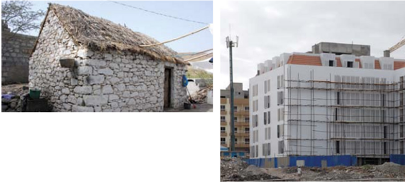
FIGURE 16.51 Heat protection: (1) Whitewashed vernacular house, on Santo Antão, (2) contemporary building painted white, in Mindelo, Cape Verde.
