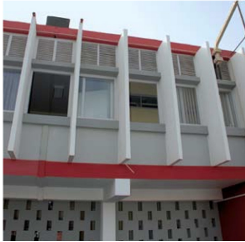
FIGURE 16.76 Modernist building in Praia, with façade ventilation openings at various levels: high, for air exchange and cooling of the building mass, and lower (windows) for the comfort of occupants. The need for natural ventilation and shading were factors that were considered in the design of the building, which is visible in the façade typology.
