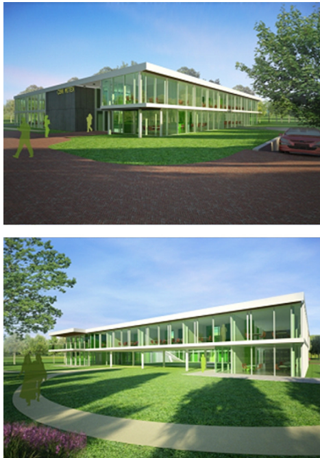
FIGURE 1.12 View of the main entrance and the back of the building [Rau].
