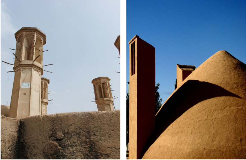
FIGURE 14.4 Wind towers could have various numbers of faces, mainly depending upon the availability of wind and the function of the space beneath. (Left photo: Hajar Maghbouli; Right photo: MasihMostajeran)
