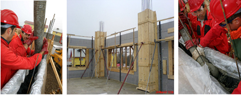
FIGURE 15.8 Amvic Marc Insulated Concrete Forms building system.
