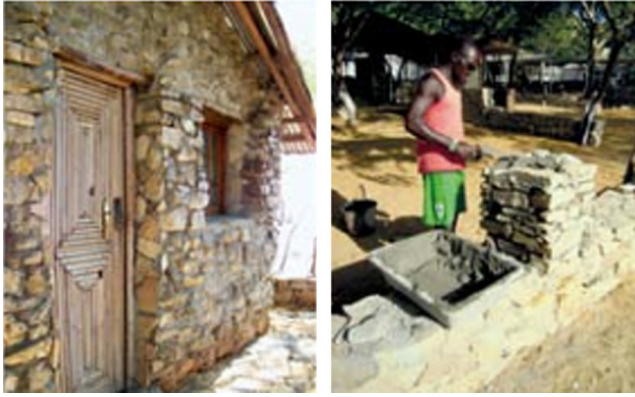
FIGURE 16.108 New construction near Luanda, using massive materials – brick, stone and concrete, which provide thermal inertia to the building. This type of construction is adequate in hot climates with significant amplitudes between daytime and night time temperatures.
