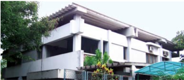
FIGURE 16.81 Ventilated roof in Maputo, Mozambique.
