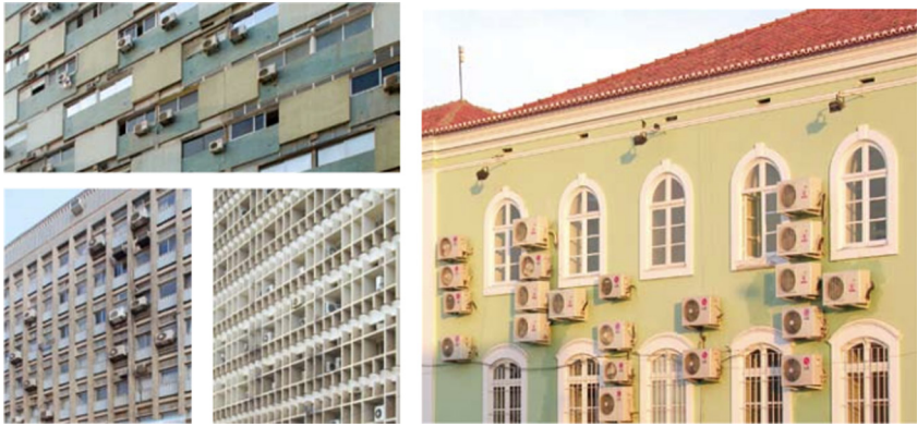
FIGURE 16.123 Luanda, Angola: the use of air conditioning can be avoided through a correct use of passive design, reducing damage to the environment and operation costs.
