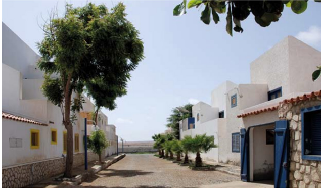
FIGURE 16.23 Use of porches and vegetation canopies for protection against solar radiation in residential buildings (Cape Verde).
