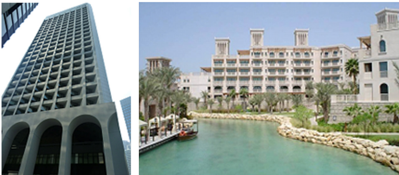
FIGURE 17.6 Good practice in high rise buildings with proper shading, and a recent hotel in Dubai with wind towers.
