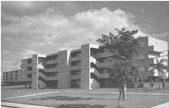
FIGURE 8.17 Open urbanization based on typical housing blocks for workers, Arch. Martínez Inclán, Romañach, Quintana and Mantilla, Guanabacoa, 1948. (From Rodríguez, E. L., The Havana Guide. Modern Architecture 1925 – 1965 , Princenton Architectural Press, New York, 1999)
