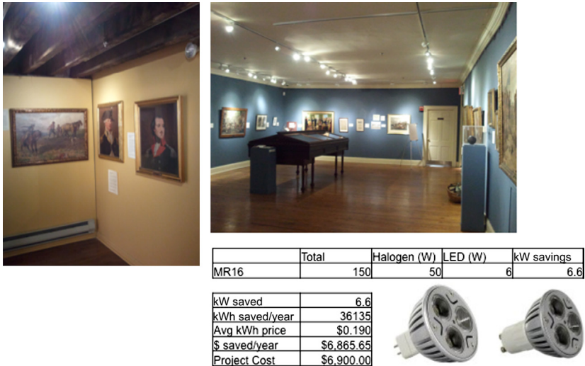
FIGURE 7.9 Pictures of the LED MR16 retrofit at the Sons of the Revolution museum in NYC; a summary table and a picture of the specific product used.
