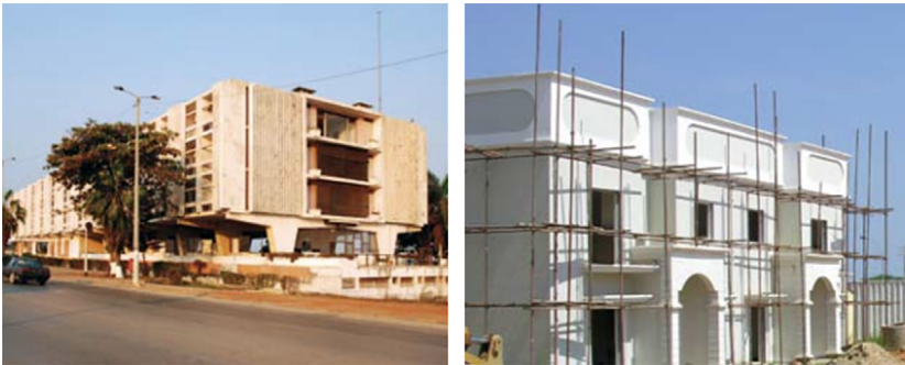
FIGURE 16.53 Buildings painted white, in Luanda, Angola: the painting of buildings with light colors (e.g. using whitewash), would be an economical way to significantly reduce the discomfort from overheating.
