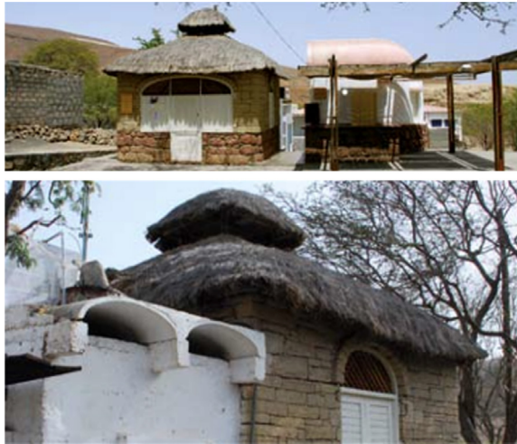
FIGURE 16.107 Tourist information building in Santo Antao, built using hollow concrete slabs, and incorporating openings on the roof for ventilation.
