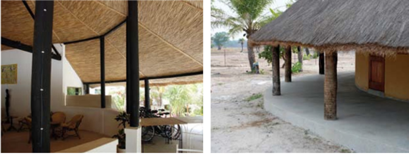
FIGURE 16.41 Fixed Shading: left – shading projection of roof in a contemporary residential building in Guiné-Bissau. Right: shaded streets in Bissau.
