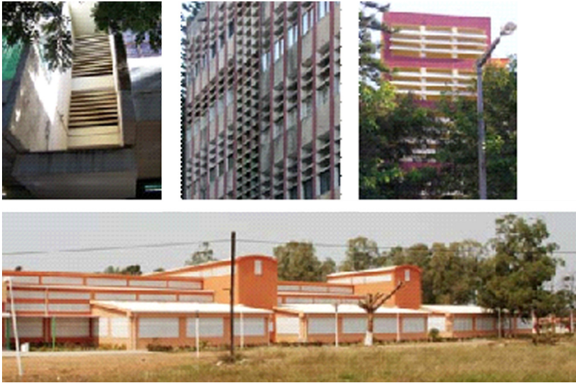
FIGURE 16.72 'Brise-Soleil' grills in Mozambique, for shading and natural ventilation.
