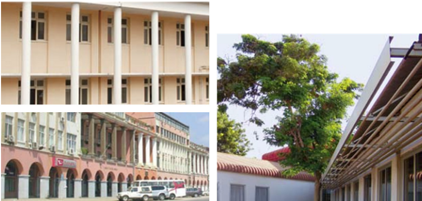
FIGURE 16.34 Fixed shading in Luanda: Above: porch (left); shaded roof (center): 'Brise-soleil' (right). Below: arcades (left) and a fixed shading device at the Faculty of Architecture's building.
