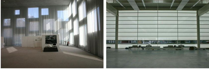
FIGURE 9.20 Examples for light scattering windows. Left: Light diffusing curtains, Folkwang Art School, Essen, Germany, Sanaa Architects. Right: Fritted glass for illumination as well as solar thermal and glare control, Sedac production hall, Gersthofen, Germany. Architect: Thomas Herzog and partners.
