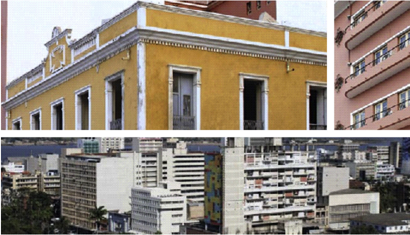
FIGURE 16.65 Most residential buildings we find in more established urban areas in Cape Verde (above), Angola (center), Guiné (below) and Mozambique (bottom) have very reasonable glazing areas. They are a good reference for the design of new buildings. The area of glass should not exceed 30% of the total area of the main façade, and should be fully shaded.
