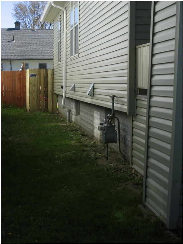
Exterior above grade insulation.
