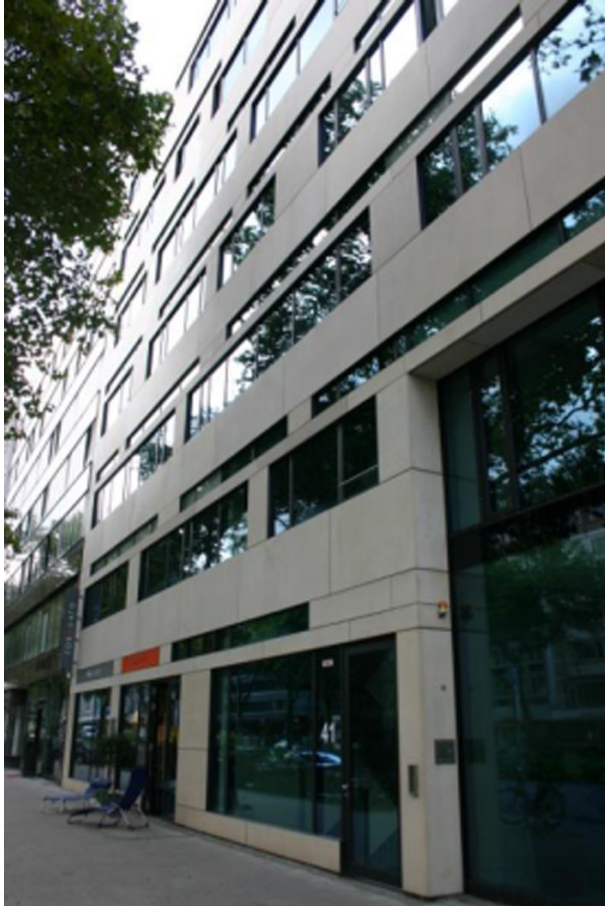
FIGURE 9.10 Separate clerestory windows above eye level with special glass for redirection of sunlight deep into the room. Duesseldorfer Hypothekenbank, Germany, Koch Architects.
