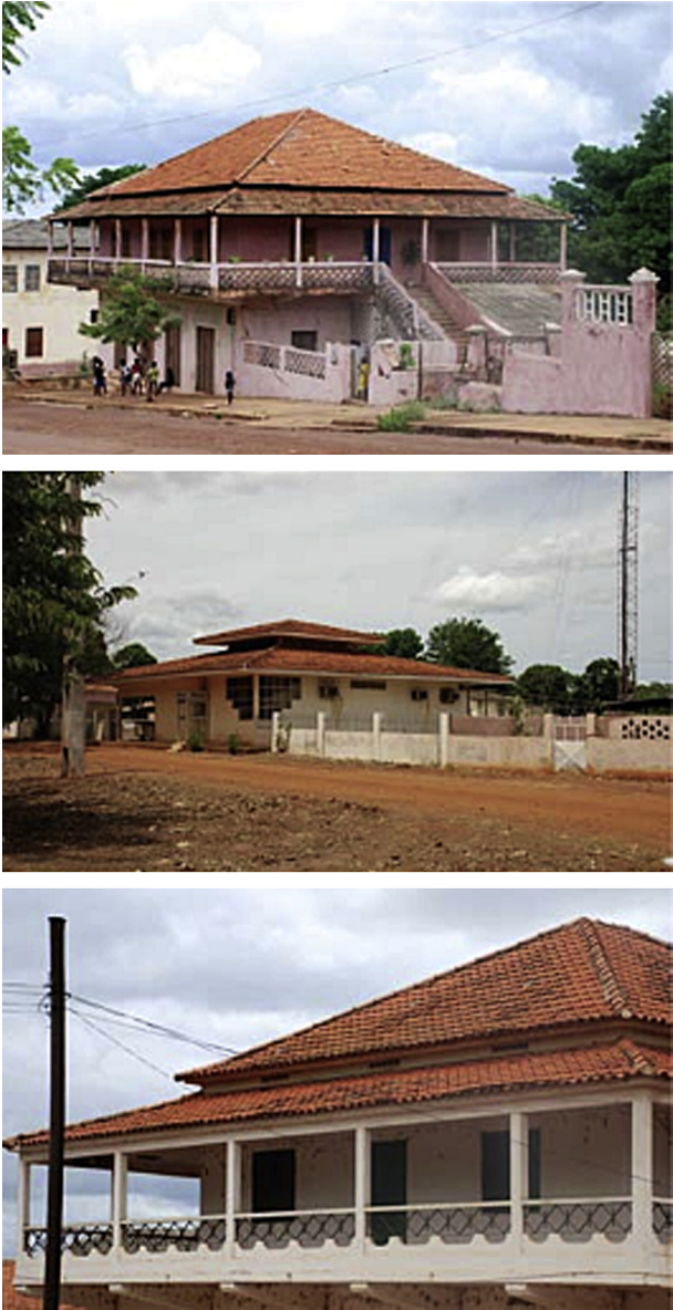
FIGURE 16.71 Ventiladed roofs in Guiné-Bissau.
