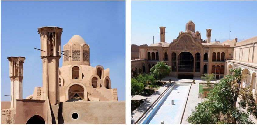
FIGURE 14.2 Various types of apertures, in combination with wind towers guaranteed maximum air circulation in a hot and dry climate; Borujerdiha House, Kashan, Iran. (Photos: Masih Mostajeran)
