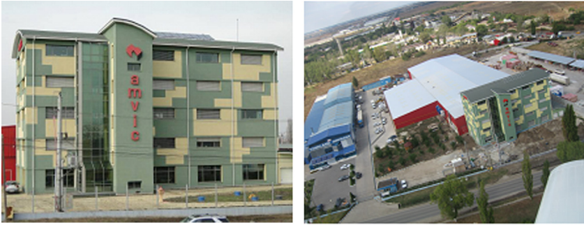
FIGURE 15.4 Amvic MARC Bragadiru Head Office, Romania.
