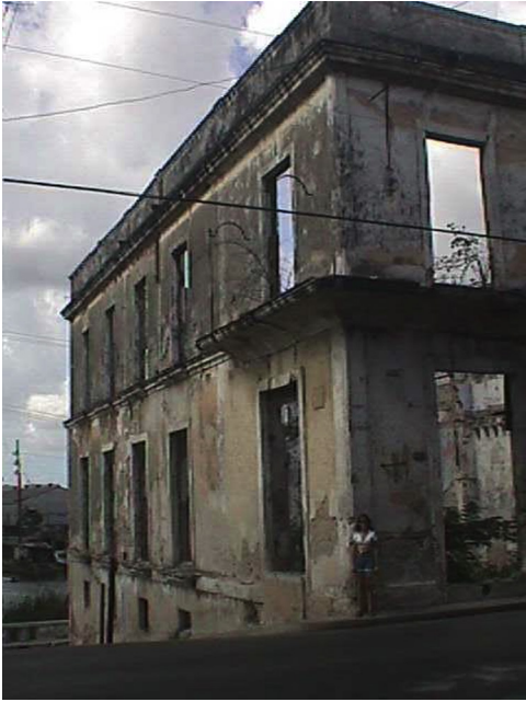
FIGURE 8.28 External wall of the preexisting building.
