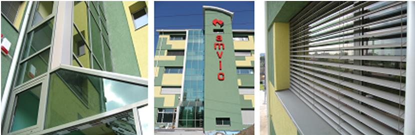
FIGURE 15.9 Amvic Marc office building, Bragadiru, Romania – passive windows and solar protection.
