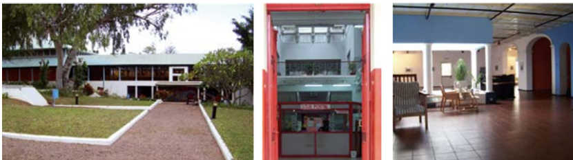
FIGURE 16.82 Ventilated atria in two buildings in Maputo, Mozambique.
