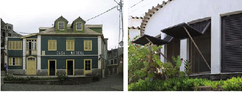
FIGURE 16.68 External venetian blinds in Ribeira Grande and in Mindelo. As well as shading, they allow and direct the flow of natural ventilation.
