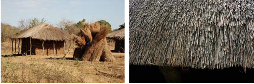
FIGURE 16.56 Vernacular houses in Praia, Cabo Verde (above) and Pemba, Mozambique (below), with thatched roofs. Thatch is an insulating material that protects the building against heat gains.
