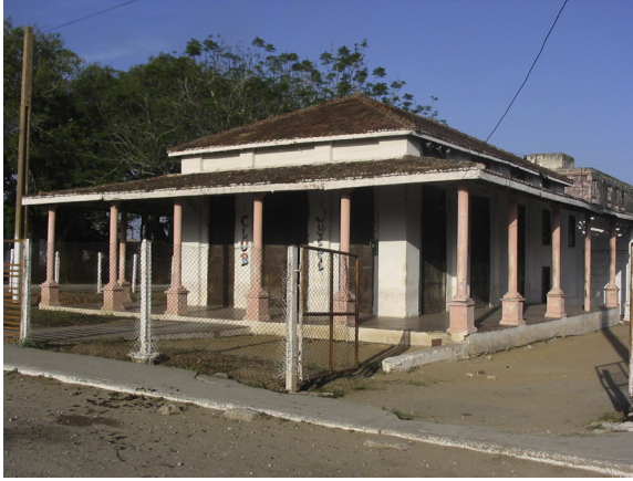
FIGURE 8.5 House surrounded by a corridor and enhancing convective ventilation in 'Oriente'.
