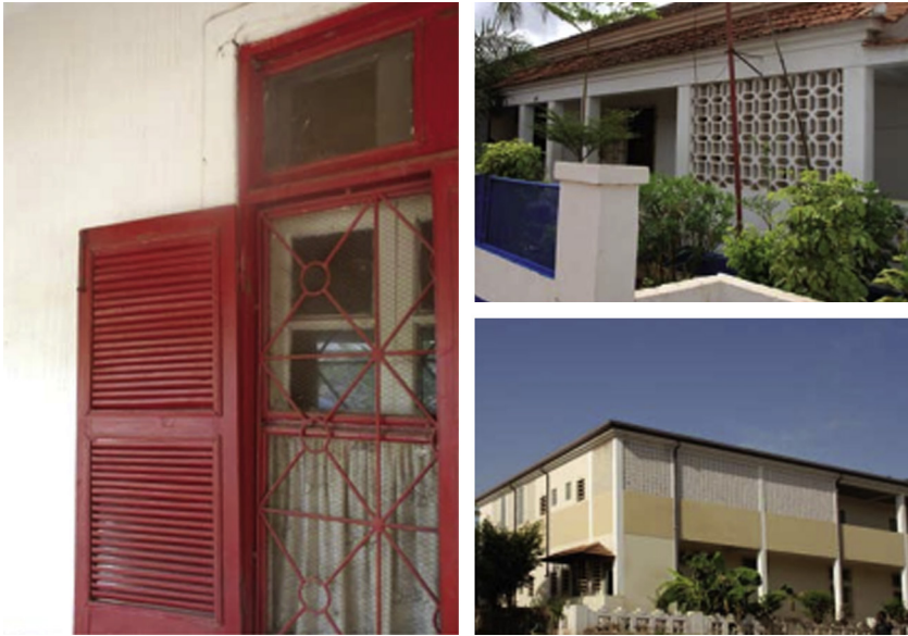
FIGURE 16.70 External fixed shading systems in Guiné-Bissau. As well as shading, they allow and direct the flow of natural ventilation.
