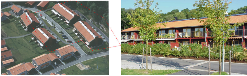
FIGURE 12.6 The situation of the four sets of buildings in Lindås (left), and one of the four blocks of buildings (right).
