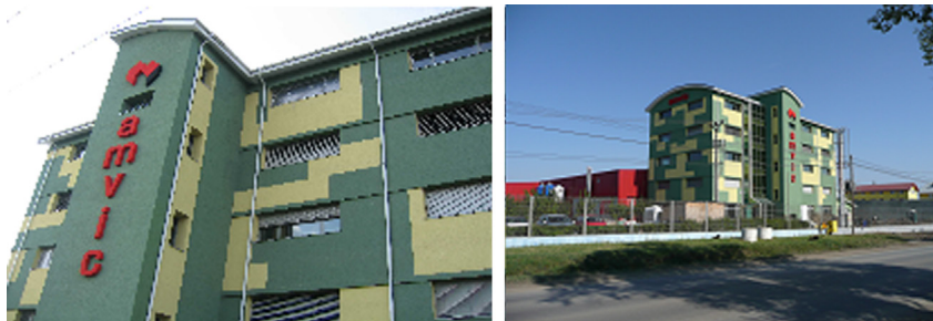
FIGURE 15.6 Amvic MARC Bragadiru Head Office Romania.
