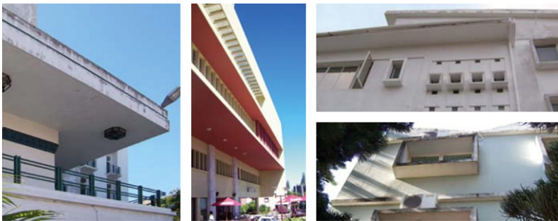
FIGURE 16.43 Fixed shading in modern buildings, Maputo, Mozambique.
