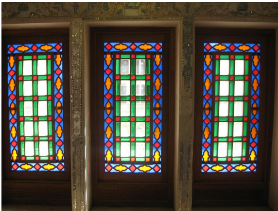
FIGURE 14.6 Stained glass on windows of traditional houses could restrict the entry of daylight and view; Abbasian House, Kashan, Iran.
