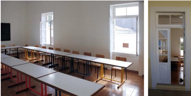
FIGURE 16.77 The interior of a school in Mindelo. (1): The inner openings have a generous height, allowing the flow of ventilation at a higher level, and contributing to a good performance in terms of natural lighting. (2): open windows for natural ventilation when the outside temperature is comfortable during the day.
