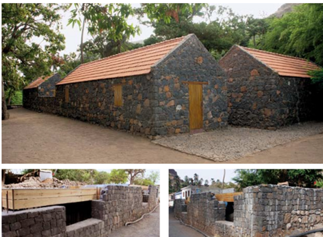
FIGURE 16.110 Hostel designed by Alvaro Siza in Cidade Velha. New construction using materials with high thermal inertia (stone and concrete).
