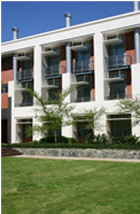
FIGURE 9.17 Light shelves for daylighting and shading. BP headquarters, Capetown, South Africa, Architects.
