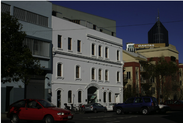
FIGURE 13.18 60 Leicester Street, Melbourne – rooftop with thermal chimneys and atrium glazing.
