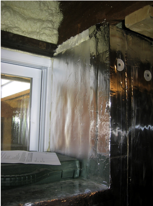
Interior foundation insulation.
