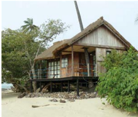
FIGURE 16.112 Guiné-Bissau: the use of lightweight buildings may offer advantages in zones with low thermal amplitudes (below 8°C between night and day during most of the year), where thermal inertia has little effect. Building features like elevated structures, ventilated roofs and wind-catching verandas can be used to improve ventilation.
