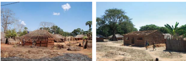
FIGURE 16.113 In Mozambique, the use of massive building materials, like earth, stone, bricks or concrete, can be observed throughout the country. Above: adobe and stone vernacular houses in Ilha de Moçambique. Below: brick and concrete construction in Maputo.
