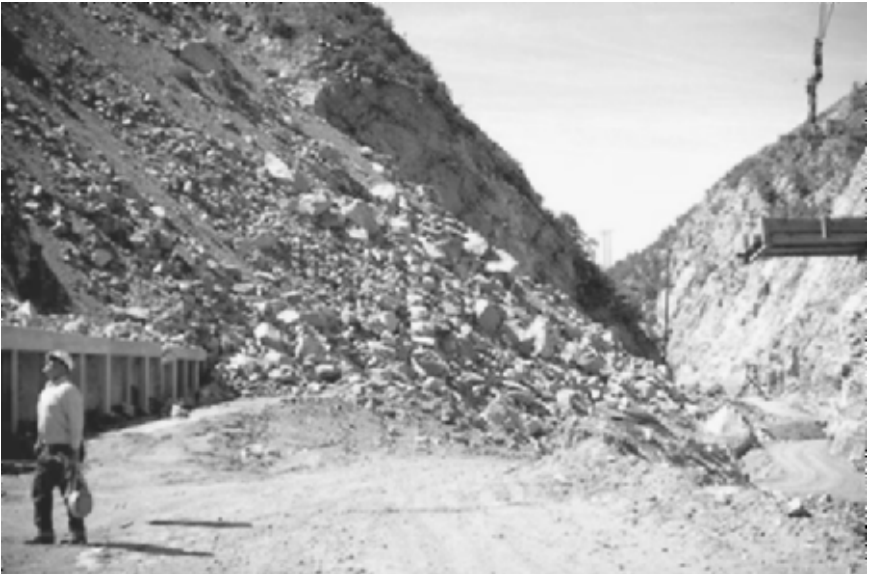
FIGURE 9.4 Rock slide at the Pacoima Dam caused by the San Fernando earthquake in California on February 9, 1971. (Photograph from the Steinbrugge Collection, EERC, University of California, Berkeley.)
