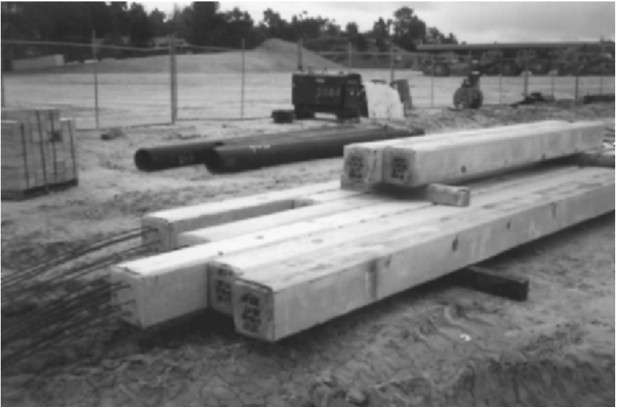
FIGURE 13.19 Prestressed concrete piles stockpiled at the job site.
