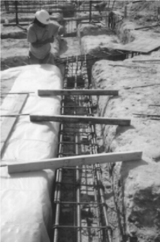
FIGURE 13.12 Steel reinforcement is being installed within the grade beam excavation.
