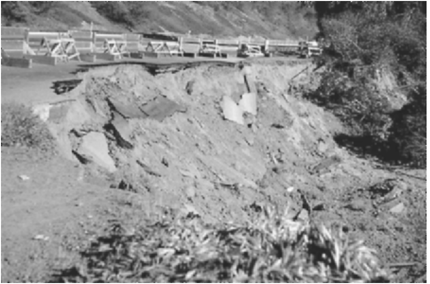
FIGURE 9.36 One of several earthquake-induced slides along Skyline Boulevard at Lake Merced, San Francisco. The slides were caused by the Daly City earthquake in California on March 22, 1957. (Photograph from the Steinbrugge Collection, EERC, University of California, Berkeley.)
