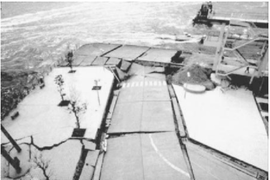
FIGURE 3.29 Settlement and lateral spreading damage due to retaining wall movement caused by the Kobe earthquake on January 17, 1995. The location is near the northwest corner of the Port Island Bridge. (Photograph from the Great Hanshin Bridge Collection, EERC, University of California, Berkeley.)
