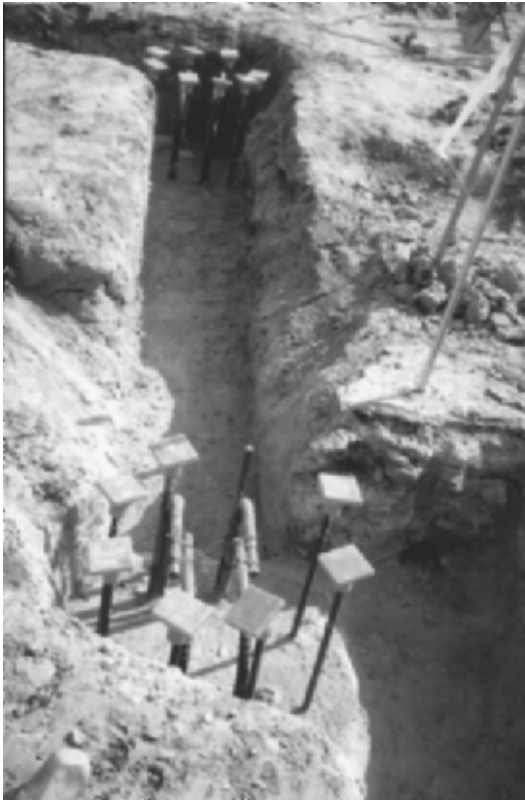
FIGURE 13.11 Excavation for the grade beam that will span between the two piers.
