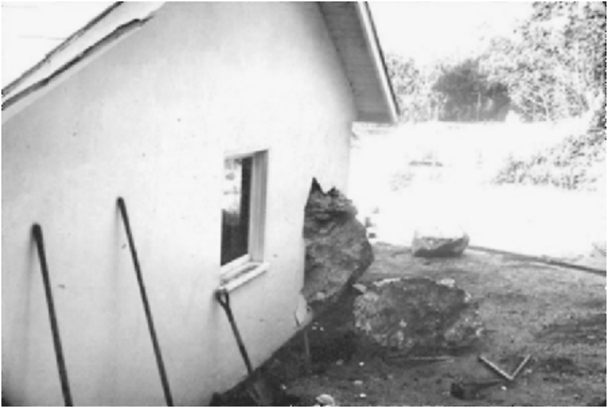
FIGURE 9.1 A rockfall that struck a house located at the mouth of Pacoima Gorge. The rockfall was caused by the San Fernando earthquake (magnitude 6.6) in California on February 9, 1971. (Photograph from the Steinbrugge Collection, EERC, University of California, Berkeley.)
