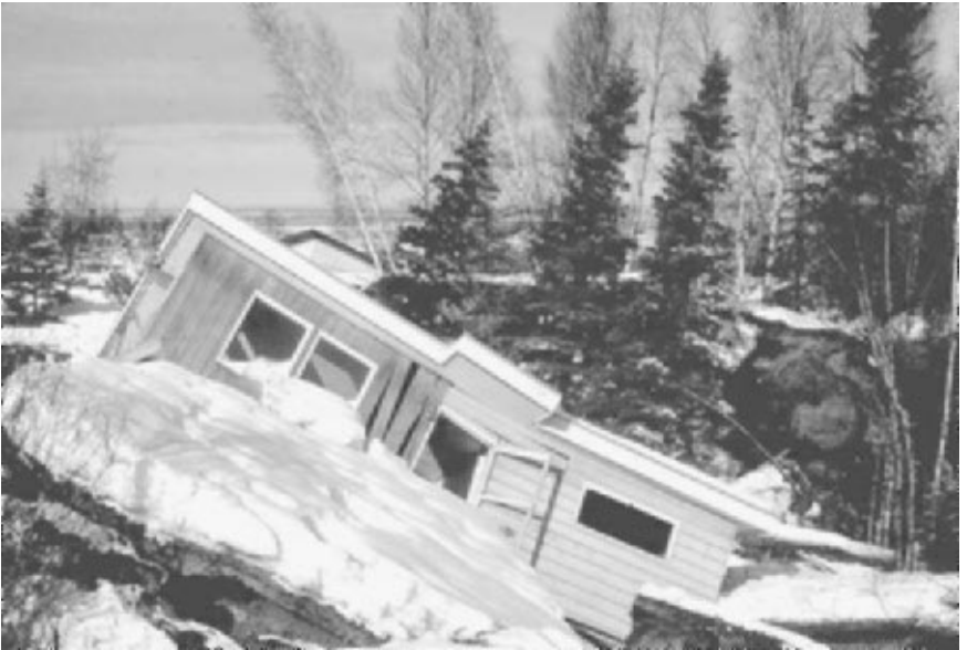
FIGURE 3.48 Damage caused by movement of the Turnagain Heights landslide during the Prince William Sound earthquake in Alaska on March 27, 1964. (Photograph from the Steinbrugge Collection, EERC, University of California, Berkeley.)
