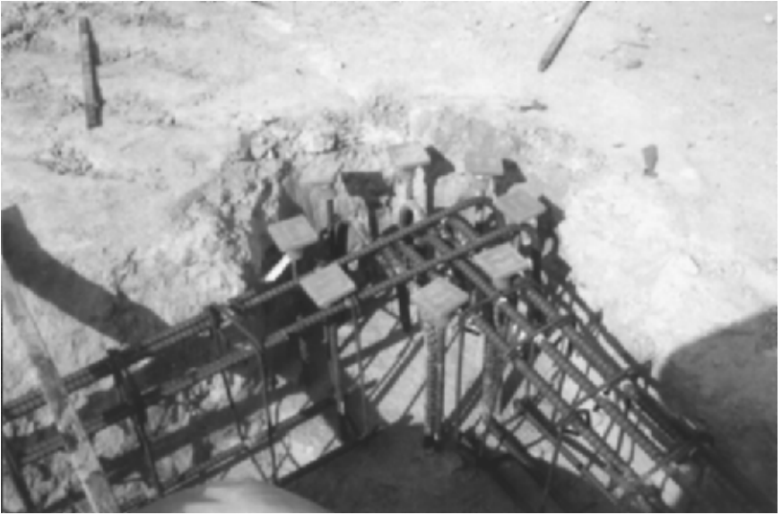
FIGURE 13.13 Corner of the building where the steel reinforcement from the two grade beams has been attached to the steel reinforcement from the pier.
