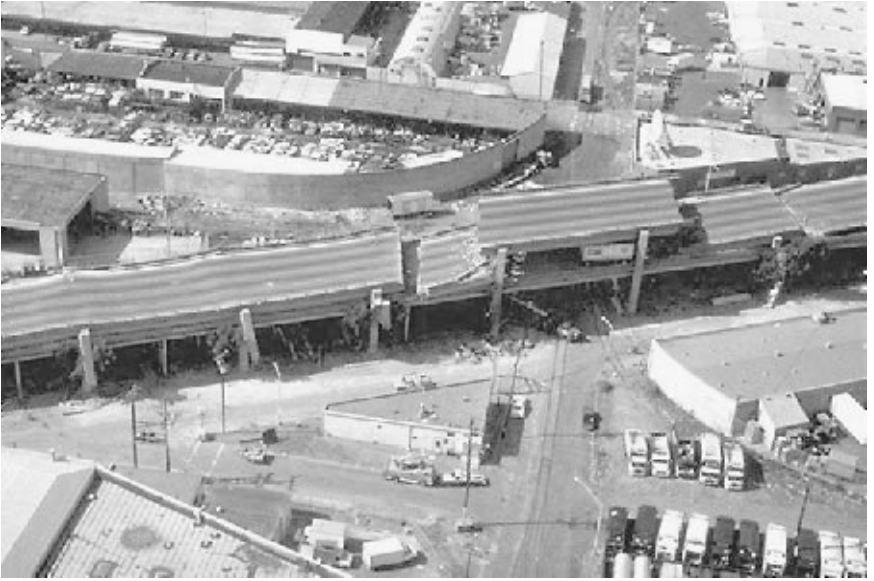
FIGURE 4.27 Overview of the collapse of the Cypress Street Viaduct caused by the Loma Prieta earthquake in California on October 17, 1989. (From USGS.)
