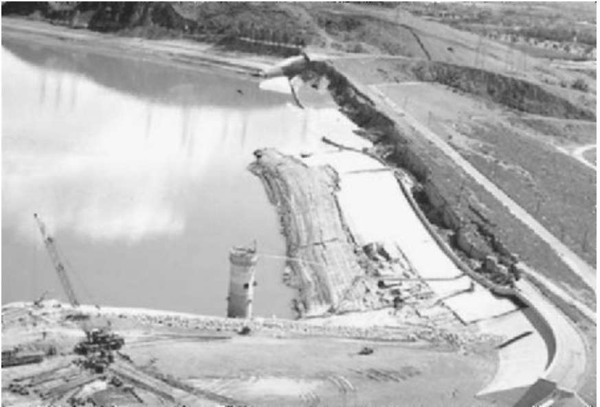
FIGURE 3.39 Flow slide of the Lower San Fernando Dam caused by the San Fernando earthquake on February 9, 1971. The photograph is a view to the east, and the main flow slide is at the eastern end of the dam. (Photograph from the Steinbrugge Collection, EERC, University of California, Berkeley.)
