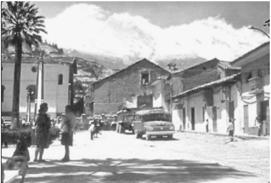
FIGURE 3.43 This photograph was taken before the earthquake-induced debris avalanche with the photographer standing in the Plaza de Armas in the central part of Yungay. Note the palm tree on the left and the large white wall of the cathedral just behind the palm tree. Compare this figure with Fig. 3.44. (Photograph from the Steinbrugge Collection, EERC, University of California, Berkeley.)
