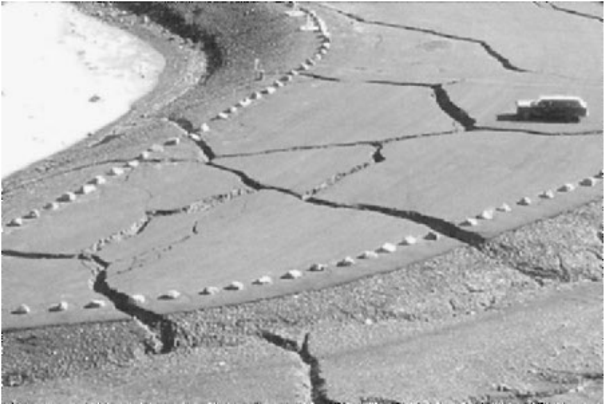
FIGURE 3.42 Lateral spreading caused by the Prince William Sound earthquake in Alaska on March 27, 1964. (Photograph from the Steinbrugge Collection, EERC, University of California, Berkeley.)
