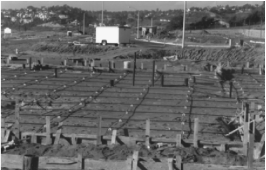
FIGURE 13.38 Construction of a post-tensioned foundation for a single-family residence.
