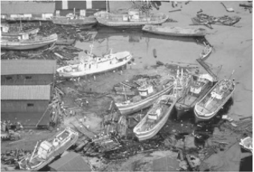
FIGURE 3.57 Tsunami damage caused by the Niigata earthquake in Japan on June 16, 1964. (Photograph from the Steinbrugge Collection, EERC, University of California, Berkeley.)
