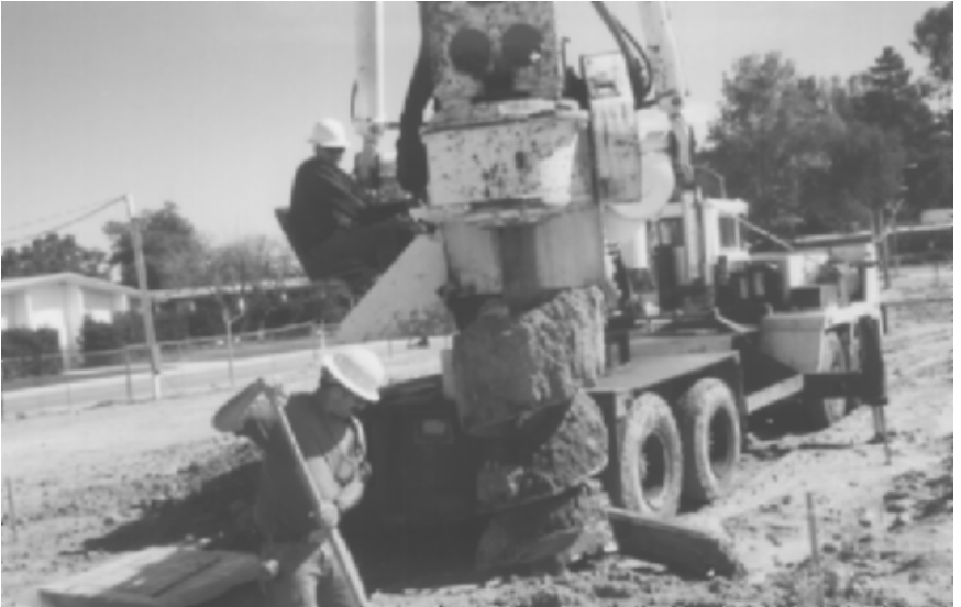
FIGURE 13.8 Close-up of auger being extracted from the ground with soil lodged within its grooves.
