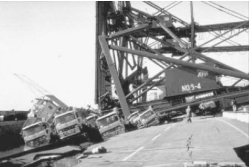
FIGURE 3.34 Collapse of a crane due to about 2 m of lateral movement of the retaining wall on Rokko Island. There was also about 1 to 2 m of settlement behind the retaining wall when it moved outward during the Kobe earthquake on January 17, 1995. (Photograph from the Kobe Geotechnical Collection, EERC, University of California, Berkeley.)
