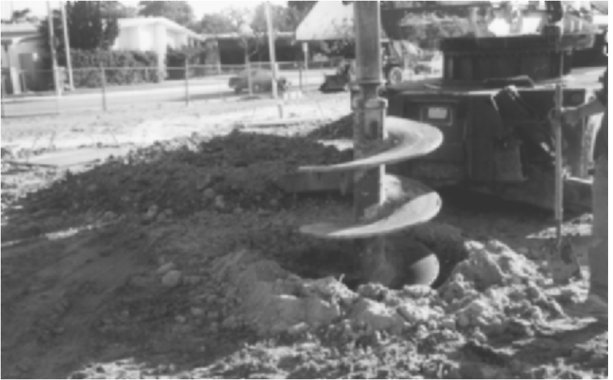
FIGURE 13.7 Close-up of auger being pushed into the soil.
