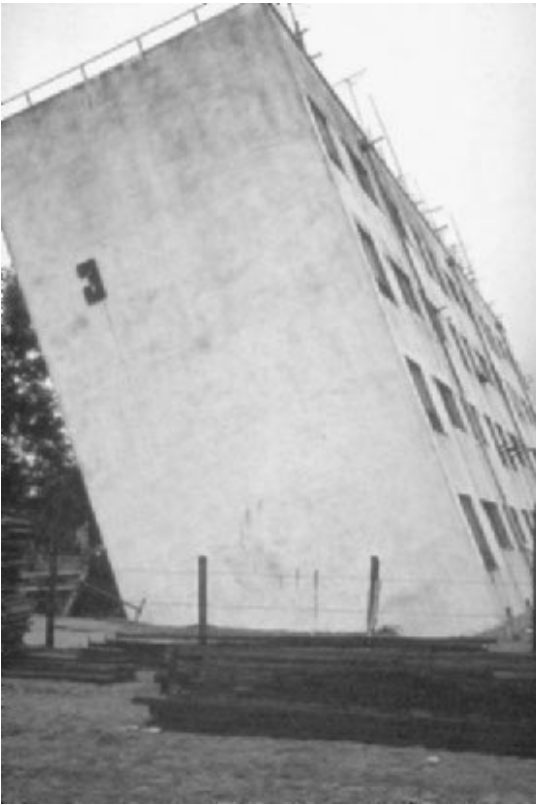
FIGURE 3.22 Settlement and tilting of an apartment building located in Niigata, Japan. The building suffered liquefaction-induced settlement and tilting during the Niigata earthquake on June 16, 1964. (Photograph from the Steinbrugge Collection, EERC, University of California, Berkeley.)
