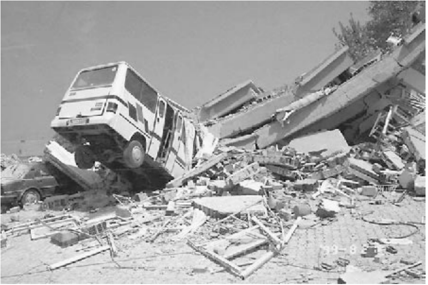
FIGURE 4.15 Pancaking of a building, which also partially crushed a bus, during the Izmit earthquake in Turkey on August 17, 1999. (Photograph from the Izmit Collection, EERC, University of California, Berkeley.)
