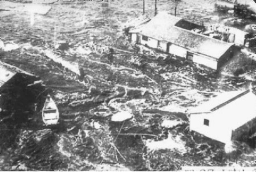
FIGURE 3.55 Tsunami in progress. The site is the village of Kiritoppu, near Kushiro Harbor, Hokkaido, Japan. The Tokachi-oki earthquake in Japan generated the tsunami on March 4, 1952. (Photograph from the Steinbrugge Collection, EERC, University of California, Berkeley.)
