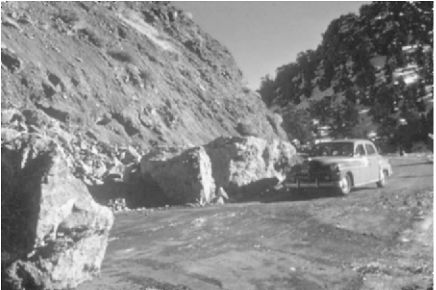
FIGURE 9.2 Large rocks from a rockfall that rolled onto the road located on the west side of Carroll Summit. The rockfall was caused by the Dixie Valley–Fairview Peaks earthquake (magnitude 7.0) in Nevada on December 16, 1954. (Photograph from the Steinbrugge Collection, EERC, University of California, Berkeley.)
