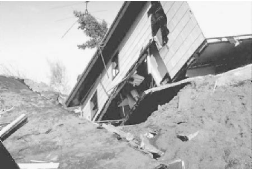
FIGURE 3.49 Damage caused by movement of the Turnagain Heights landslide during the Prince William Sound earthquake in Alaska on March 27, 1964. (Photograph from the Steinbrugge Collection, EERC, University of California, Berkeley.)
