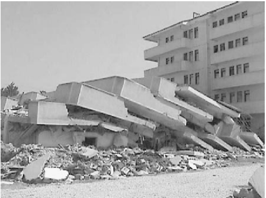
FIGURE 4.14 Pancaking of a building during the Izmit earthquake in Turkey on August 17, 1999. (Photograph by Mehmet Celebi, USGS.)
