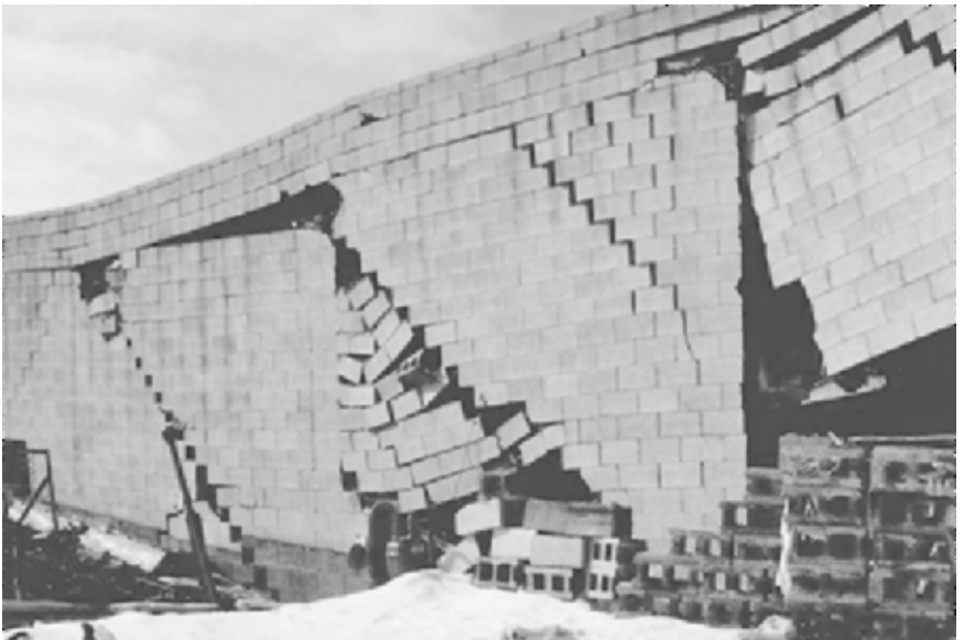
FIGURE 9.37 Building damage caused by the Fourth Avenue landslide, Anchorage, Alaska. The landslide movement occurred during the Prince William Sound earthquake in Alaska on March 27, 1964. (Photograph from the Steinbrugge Collection, EERC, University of California, Berkeley.)
