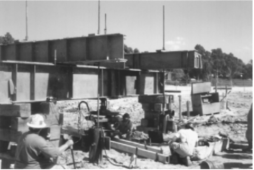
FIGURE 13.26 Pile load tests. The reaction frame has been set up, and the hydraulic jack and load cell are in place.
