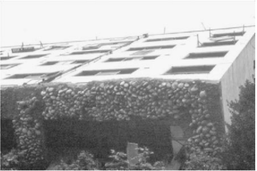
FIGURE 3.21 View of the bottom of a Kawagishi-cho apartment building located in Niigata, Japan. The building suffered a liquefaction-induced bearing capacity failure during the Niigata earthquake on June 16, 1964. (Photograph from the Steinbrugge Collection, EERC, University of California, Berkeley.)
