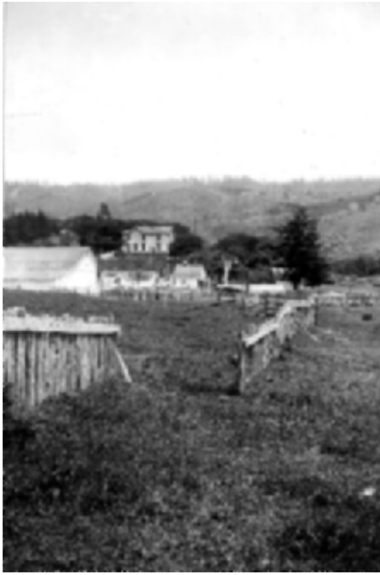
FIGURE 2.9 San Francisco earthquake, 1906. The fence has been offset 8.5 ft by the San Andreas fault displacement. The location is 0.5 mi northwest of Woodville, Marin County, California. (Photograph courtesy of USGS.)
