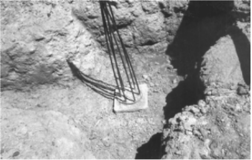
FIGURE 13.32 Close-up view of one of the prestressed piles showing a trimmed top surface with the strands extending out the top of the pile.
