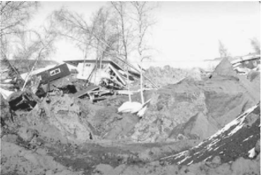
FIGURE 3.50 Damage caused by movement of the Turnagain Heights landslide during the Prince William Sound earthquake in Alaska on March 27, 1964. (Photograph from the Steinbrugge Collection, EERC, University of California, Berkeley.)
