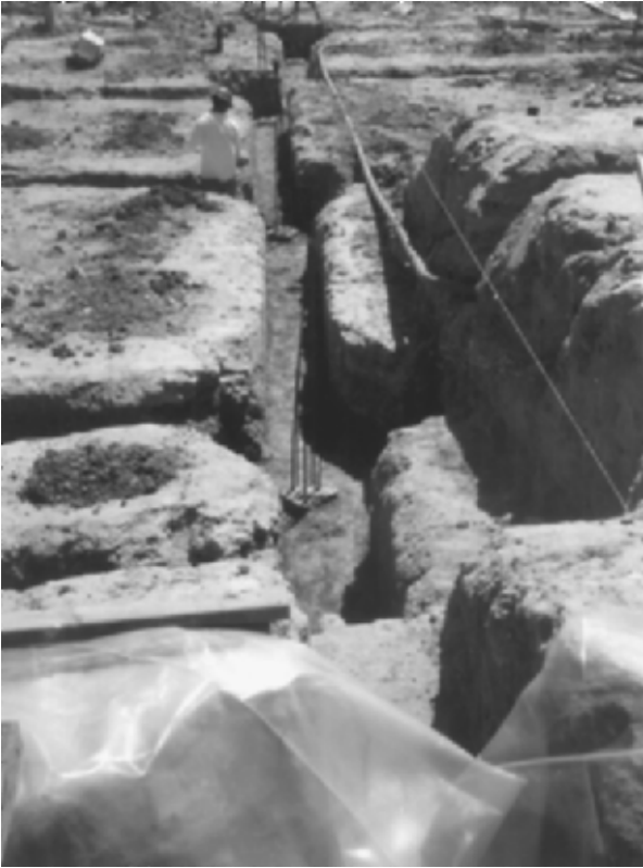
FIGURE 13.31 The excavation for the grade beams is complete, and the tops of the prestressed piles are trimmed so that they are relatively flush.
