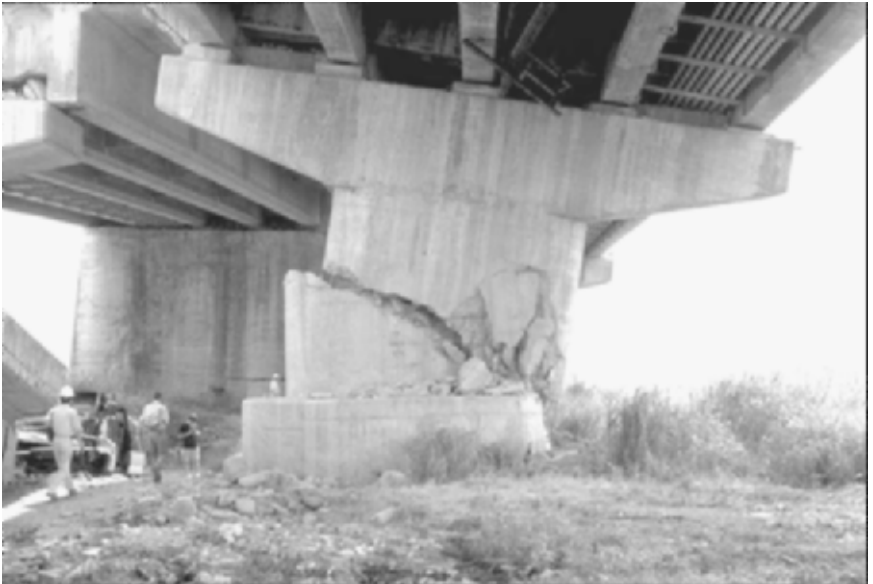
FIGURE 3.7 Close-up view of bridge pier (Wu-His Bridge) damaged by surface fault rupture associated with the Chi-chi (Taiwan) earthquake on September 21, 1999. (Photograph from the Taiwan Collection, EERC, University of California, Berkeley.)
