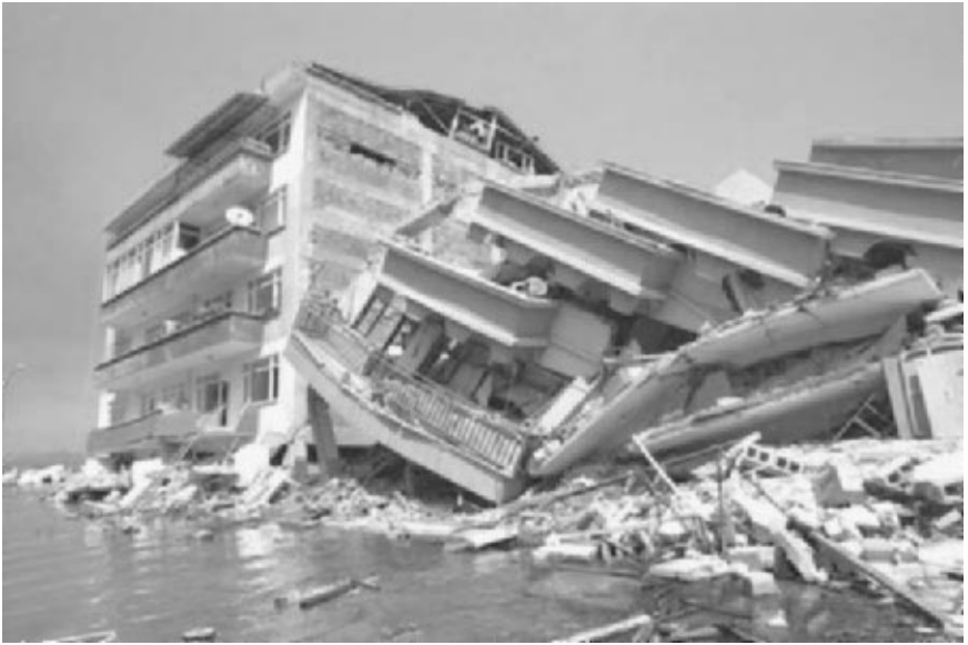
FIGURE 3.18 Flooding caused by regional subsidence associated with the Izmit (Turkey) earthquake on August 17, 1999. (Photograph from the Izmit Collection, EERC, University of California, Berkeley.)
