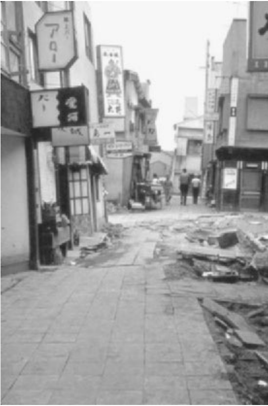
FIGURE 3.24 Settlement and tilting of relatively light buildings located in Niigata, Japan. The buildings suffered liquefaction-induced settlement and tilting during the Niigata earthquake on June 16, 1964. (Photograph from the Steinbrugge Collection, EERC, University of California, Berkeley.)
