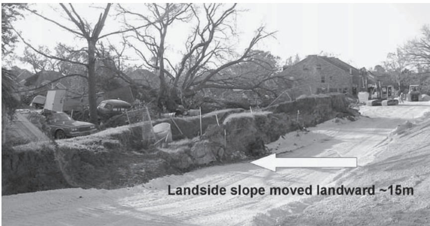
Figure 12.4 Slide at 17th St. Canal levee, New Orleans, 2005 (photo by T. Wolff).
