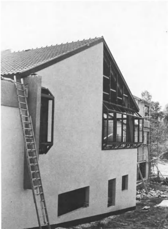
Figure 21. Detail of north-west facade (under construction)
