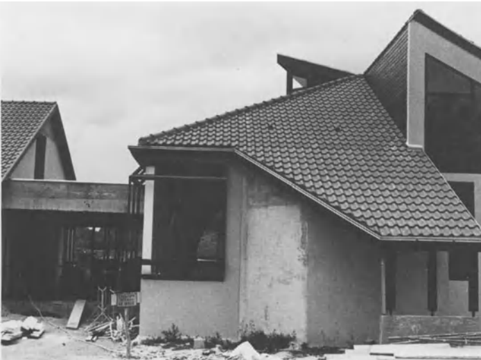
Figure 16. Detail of south-east facade (under construction)
