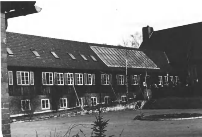
Figure 14. View of the glazed roof.
