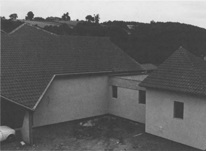
Figure 12. View of north-east wall with no windows
