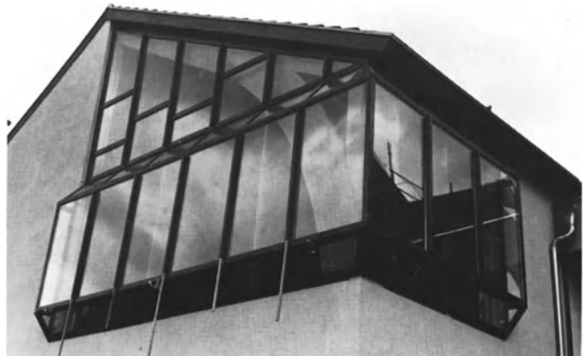
Figure 11. South-west bay window
