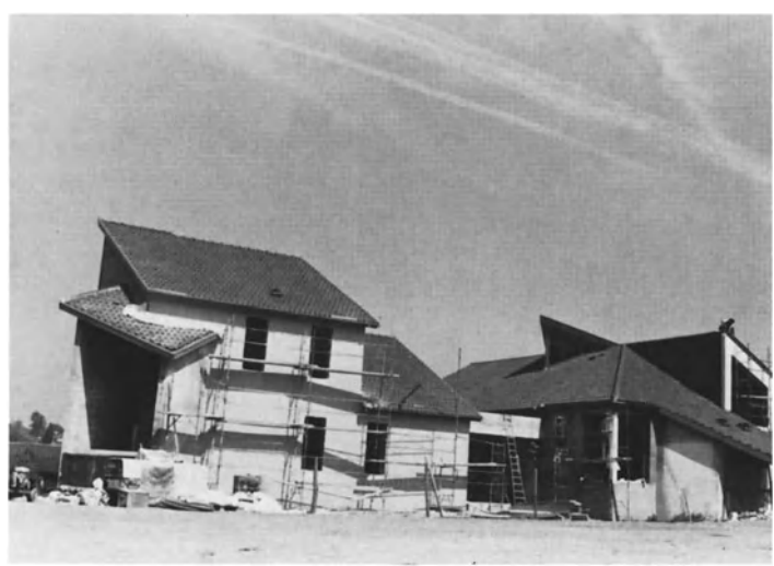
Figure 8. View of the south-east facade (under construction)
