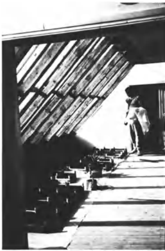
Figure 13. The foyer under the glazed roof in use as a plant nursery
