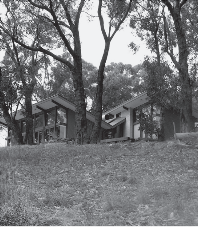
6.1 A 'solar efficient' house: Norton Summit house, architects Energy Architecture, designed with solar oriented glass, thermal mass, solar power, solar hot water and self-contained sewage system (photographer Terry Williamson).
