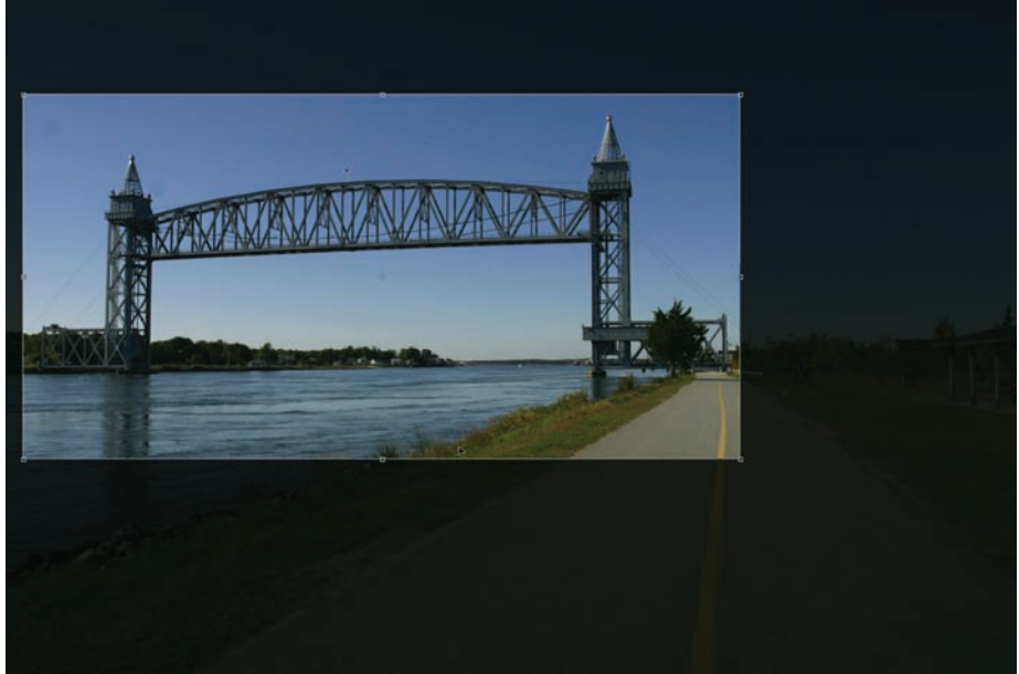
Figure 30.7. Crop the source image to the edges of the bridge before selecting.
