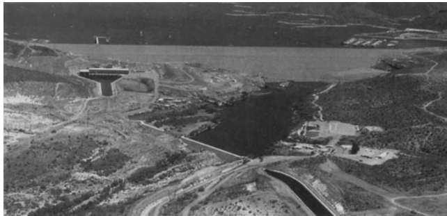
Figure 13.1.5 New Waddell Dam on the Agua Fria River in Arizona impounds Lake Pleasant. Shown downstream of dam and intake structure is the Waddell Pump/Generating Plant, which lifts Central Arizona Project (CAP) 192 feet from the canal into Lake Pleasant. The Waddell Canal connects the main CAP aqueduct with the dam. (Courtesy of Central Arizona Project.)
