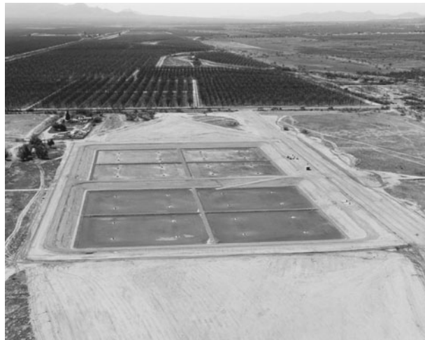
Figure 19.3.5 Pima Road recharge basin near Tucson, Arizona. (Courtesy of central Arizona Project.)
