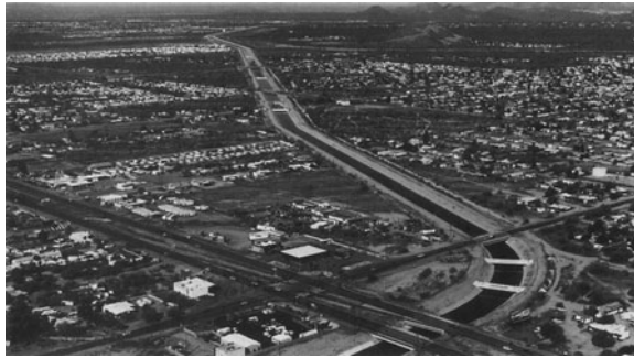
Figure 11.4.5 CAP through a residential area in Scottsdale, Arizona. (Courtesy of Central Arizona Project.)
