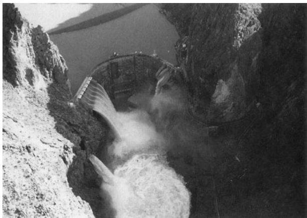
Figure 17.2.8 Horse Mesa Dam on the Salt River in Arizona showing releases in January 1993. (Courtesy of the U.S. Bureau of Reclamation, photograph by J. Madrigal, Jr. (1993).)
