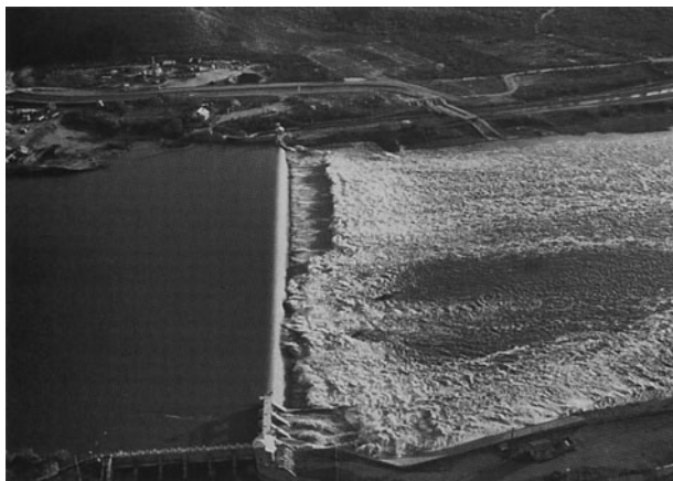
Figure 17.2.11 Granite Reef Dam on the Salt River in Arizona showing releases in January 1993. (Courtesy of the U.S. Bureau of Reclamation, photograph by J. Madrigal, Jr. (1993).)
