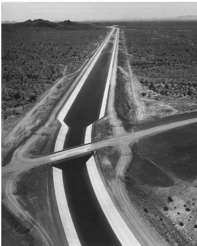
Figure 5.1.2 Hayden-Rhodes Aqueduct, Central Arizona Project. (Courtesy of the U.S. Bureau of Reclamation (1985), photograph by Joe Madrigal Jr.)
