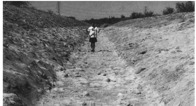
Figure 15.3.1 Views of constructed reach of Cave Creek below Cave Buttes Dam, Phoenix, Arizona. The constructed reach is straight, and cross-sections are trapezoidal in shape. The bottom and sides of the channel are composed of rounded cobbles imbedded in a matrix of cement (approximate mean diameter of the rock projections was 80 mm, about half of which seemed to be exposed to flow). Roughness elements are constant throughout the reach. The channel gradient increases from about 0.002 ft/ft at cross-section 1 to about 0.010 ft/ft at cross-section 8. The stream is ephemeral, and flow is regulated by Cave Buttes Dam (from Phillips and Ingersoll (1998)).
