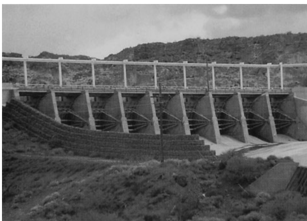
Figure 17.2.10 Stewart Mountain Dam on the Salt River in Arizona. (a), (b) Radial gates on the spillways. (Photographs by L. W. Mays.)
