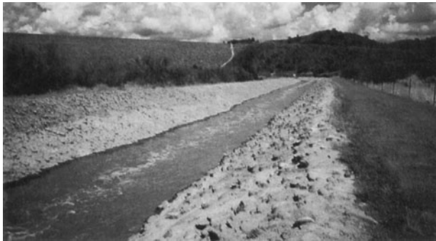
Figure 15.3.1 Views of constructed reach of Cave Creek below Cave Buttes Dam, Phoenix, Arizona. The constructed reach is straight, and cross-sections are trapezoidal in shape. The bottom and sides of the channel are composed of rounded cobbles imbedded in a matrix of cement (approximate mean diameter of the rock projections was 80 mm, about half of which seemed to be exposed to flow). Roughness elements are constant throughout the reach. The channel gradient increases from about 0.002 ft/ft at cross-section 1 to about 0.010 ft/ft at cross-section 8. The stream is ephemeral, and flow is regulated by Cave Buttes Dam (from Phillips and Ingersoll (1998)).
