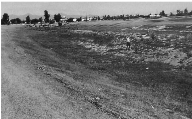
Figure 15.3.2 Views of Indian Bend Wash in Scottsdale, Arizona. The constructed channel is uniform and cross-sections are trapezoidal in shape (channel bottom is firm earth with seasonal growth of grasses and small brush) (from Phillips and Ingersoll (1998)).
