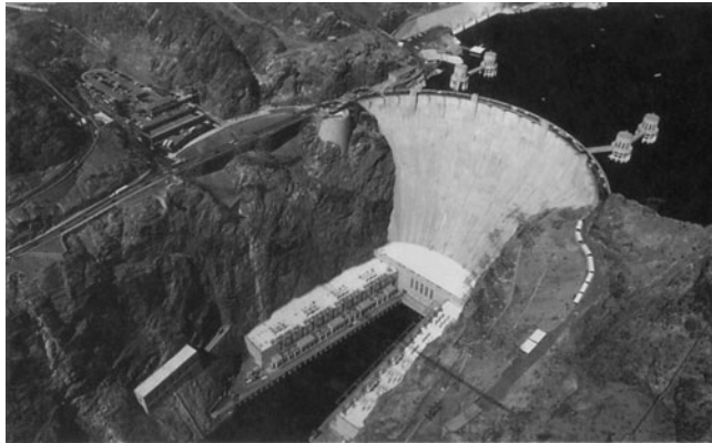
Figure 13.1.4 Hoover Dam and power houses on Colorado River in Arizona. Example of storage project having maximum reservoir storage of 34.852 \times 10^6 \text{ m}^3 . Present rated capacity is 1951 MW with planned rated capacity of 2451 MW. (Courtesy of U.S. Bureau of Reclamation, photograph by A. Pernick, March 31, 1996.)
