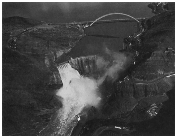
Figure 17.2.7 Roosevelt Dam on the Salt River in Arizona showing releases in January 1993. (Courtesy of the U.S. Bureau of Reclamation, photograph by J. Madrigal, Jr. (1993).)
