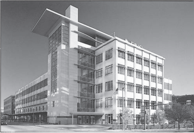
Figure 1-1(B). Commercial construction.
