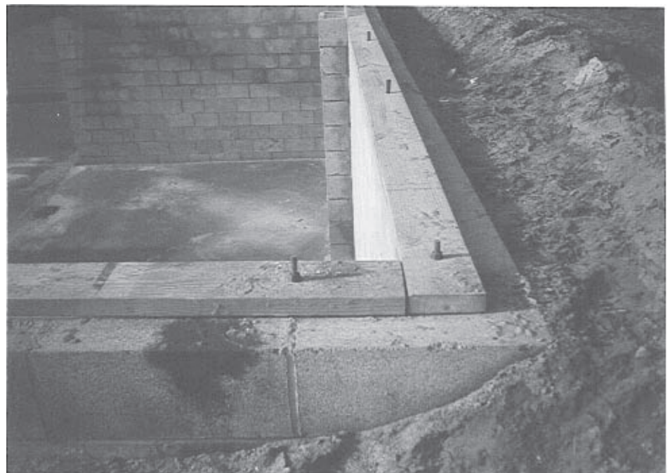
Figure 17-1. Sill plate.
