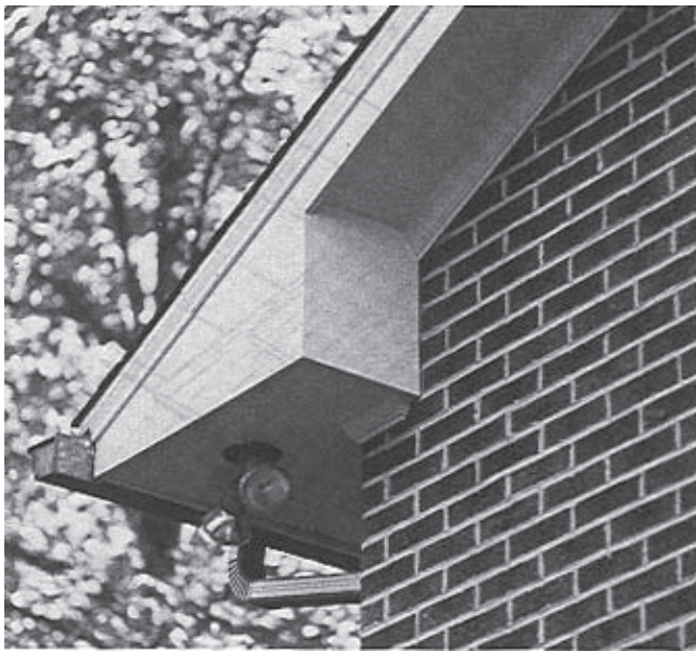
Figure 24-9. Cornice return. Courtesy of Richard T. Kreh, Sr.
