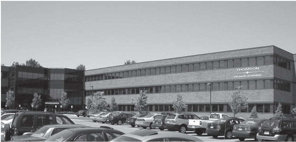
Figure 37-1. Generally, medium to large commercial buildings are very functional in design.
