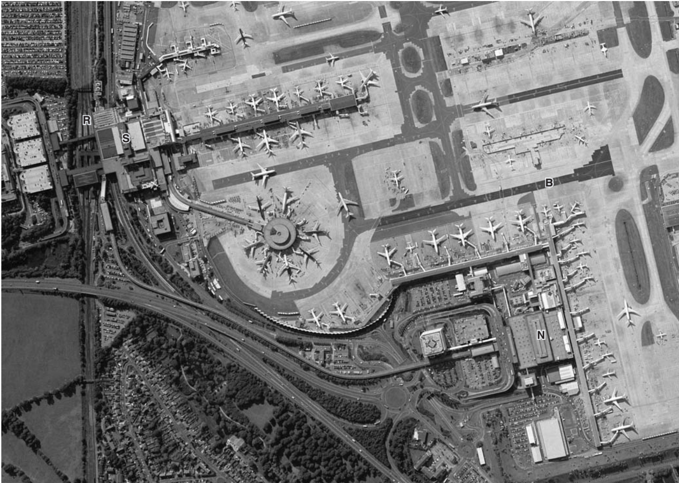
▲ 6.51 Gatwick Airport: aerial photo (courtesy of www.baa.com/photolibrary).
