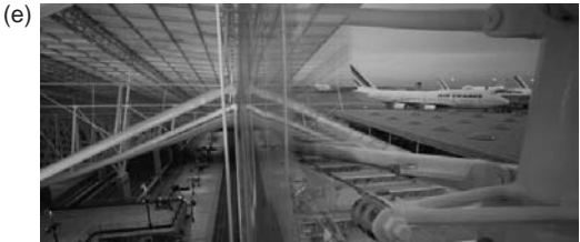
▲ 6.34 (a–e) Views of rail station and adjacent aircraft stands (Courtesy of Aeroports de Paris).
