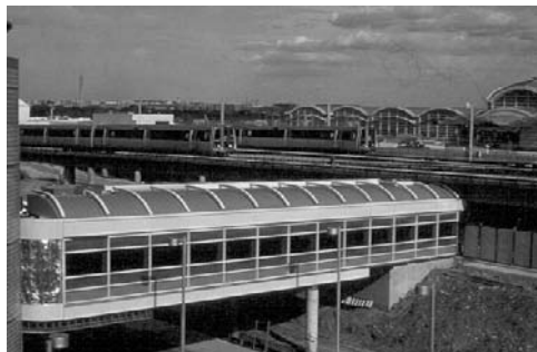
▲ 6.100 (a, b) Metro at airport terminal (Courtesy of Metropolitan Washington Airport Authority).
