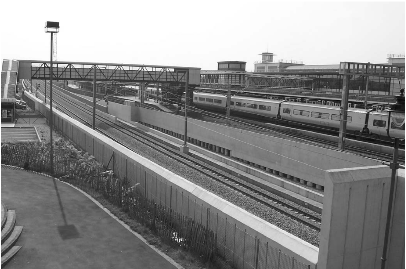
▲ 6.126 Railway-side photo showing bypass for non-stop trains, domestic platform, international station and terminal building in background.
