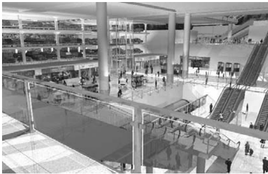
▲ 4.1 The rail parkway: circulation area and LRT platforms (Figures 4.1–4.6 courtesy of Halliburton KBR/YRM Architects Designers Planners).
