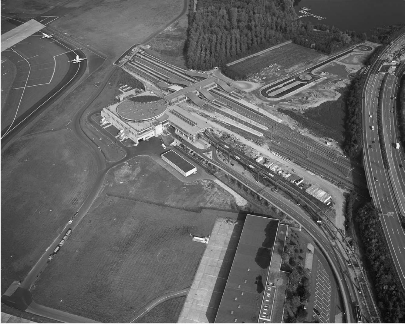
▲ 6.114 Aerial photo of rail station (Courtesy of Düsseldorf International).
