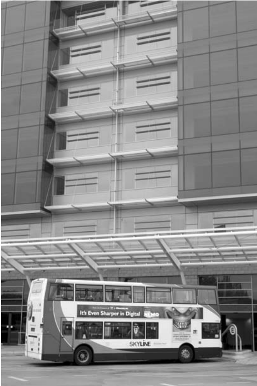
▲ 6.78 Ground Transport Interchange: bus station view (Courtesy of MA plc).
