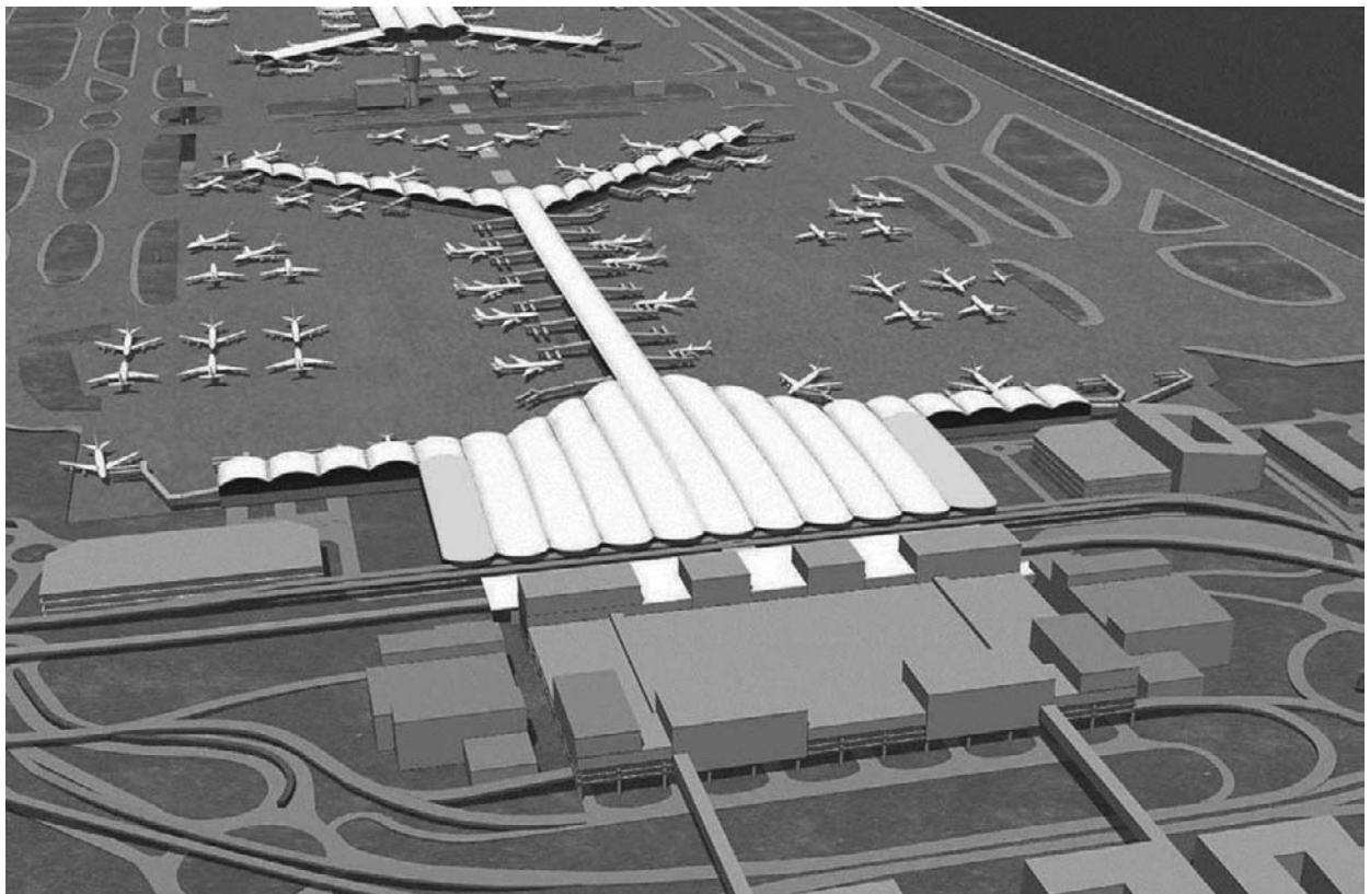
▲ 6.54 Terminal aerial view with ground transport interchange in foreground (Source: website www.hongkongairport.com ).
