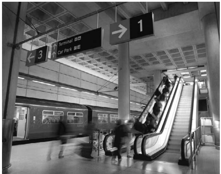
▶ 6.50 View of station platform and escalator (from Stansted Express website).
