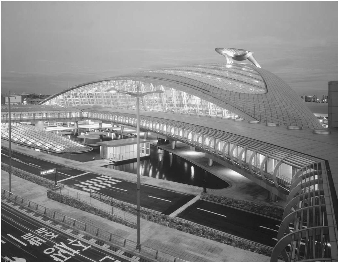
▲ 6.105 Transportation Centre, night view (Courtesy of Terry Farrell & Partners, architects).
