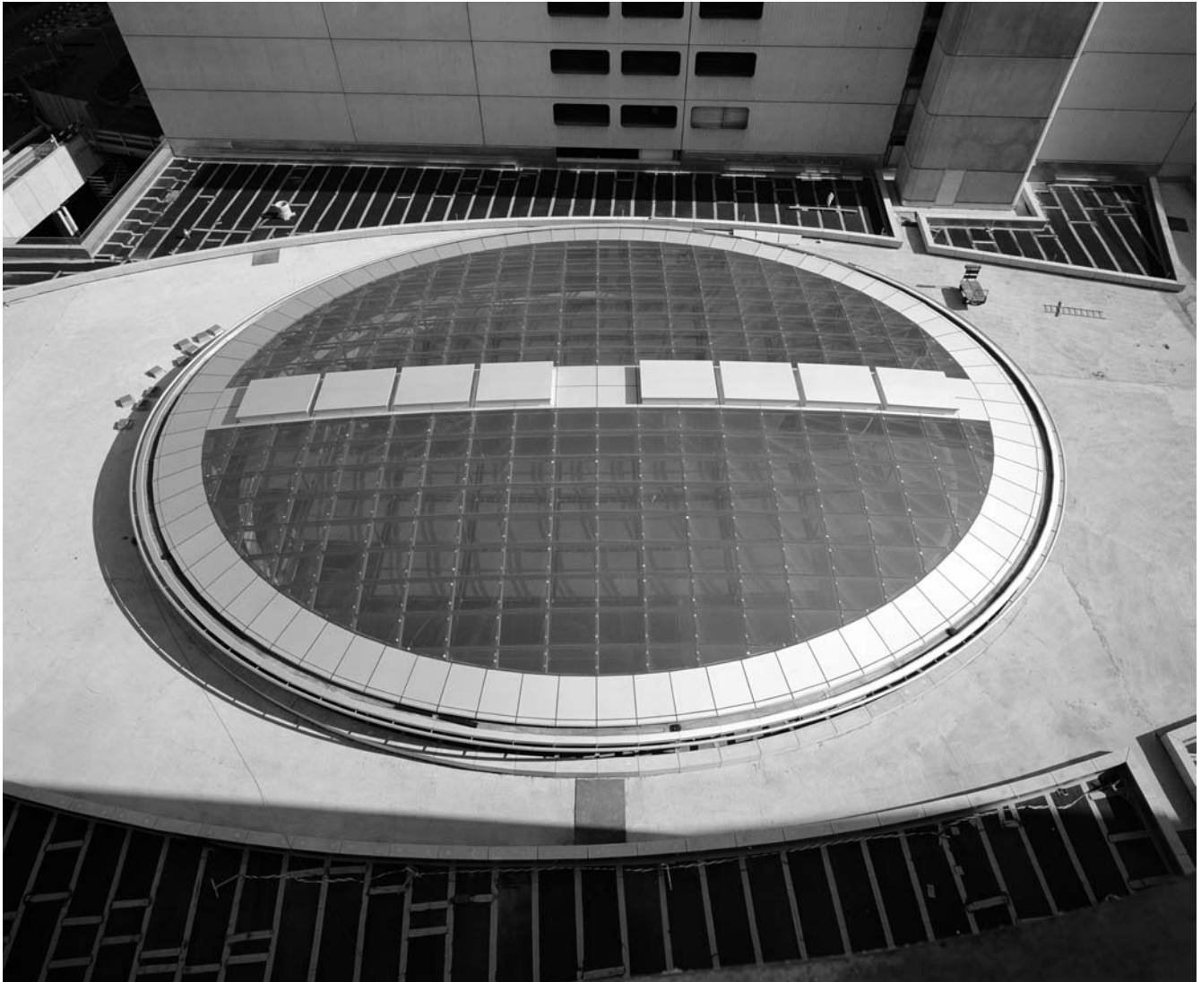
▲ 6.3 Roof of Landside Centre (Courtesy of Nicholas Grimshaw & Partners).
