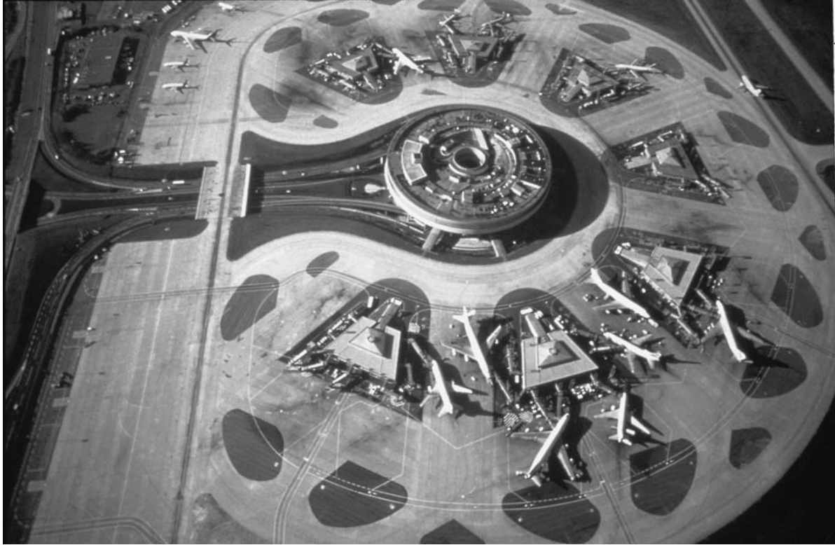
▲ 6.35 Terminal 1 aerial view, inflexible but intended to multiply (Courtesy of Aeroports de Paris).
