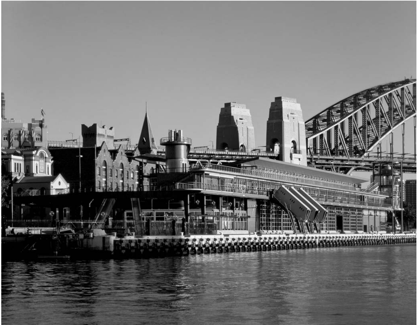
▲ 6.162 Close-up photo at water level (Courtesy of Lawrence Nield & Partners).
