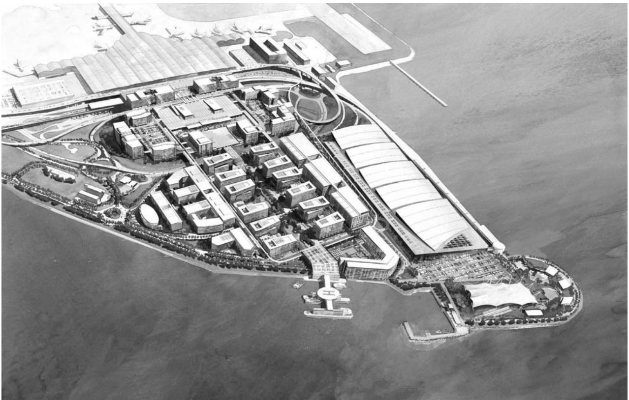
▲ 6.56 SkyCity (and ferry jetty) (Source: website www.hongkongairport.com ).
