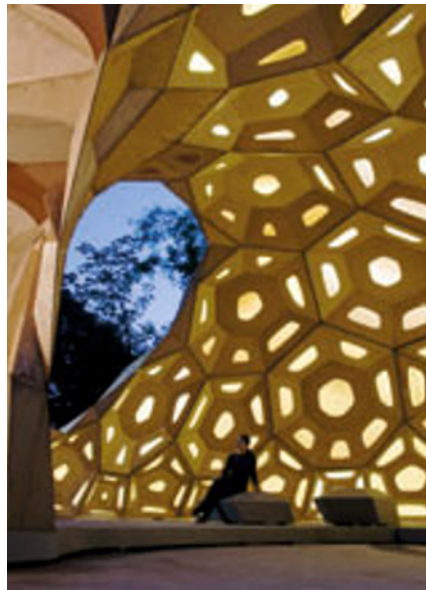
Figure 16 The prototype structure ICD/ITKE Research Pavilion 2011 consists of more than 850 geometrically unique, robotically fabricated plate morphologies with more than 100,000 individual finger joints. The use of 6.5mm plywood only demonstrates the system's structural performance capacity.
