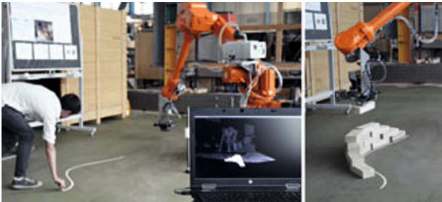
Figure 1 Brick wall robotically fabricated along gestured path. Gramazio & Kohler, ETH Zurich
