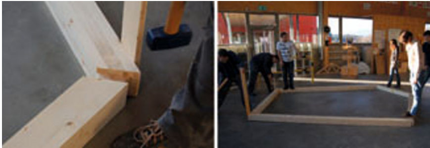
Figure 9 Assembling the pentagonal frames.
