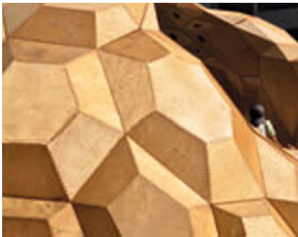
Figure 1 Close-up of the robotically fabricated finger joints connection (left); Interior view of the finished full-scale pavilion (right)
