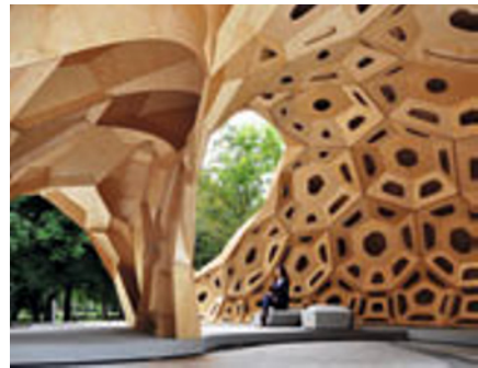
Figure 1 Close-up of the robotically fabricated finger joints connection (left); Interior view of the finished full-scale pavilion (right)
