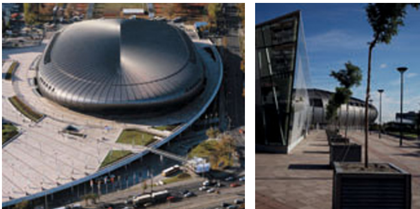
Figure 6 Papp László Budapest Sportsarena, Budapest, Hungary (completion Feb 2003); architecture: KÖZTI (Skardelli György, Pottyondy Péter), Hungary; photos: KÖZTI
