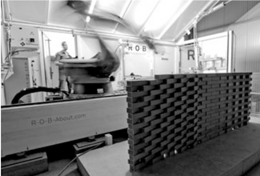
Figure 1 Robotic setup of automated brickwork process
