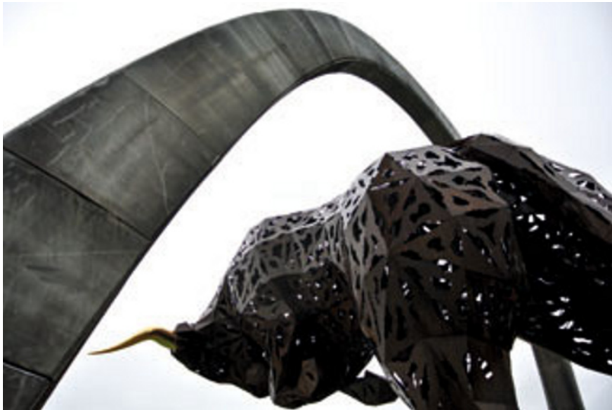
Figure 6 Traces of robotic toolpaths on the finished arch
