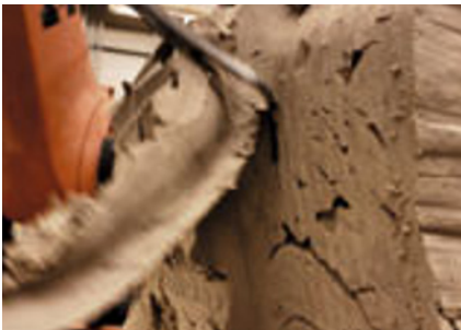
Figure 7 Air pockets found after the first pass. They were patched over and quickly recut, resulting in a smooth surface.
