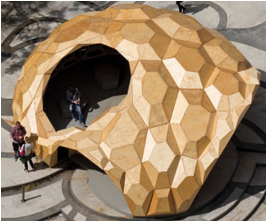
Figure 4b The development of a lightweight system of wood plate structures is based on the morphological variance of the finger joint plates enabled by robotic fabrication.
