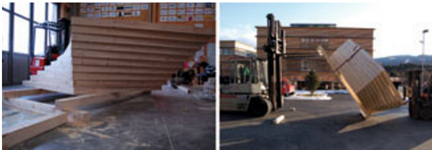
Figure 10 Combined transportable units (left); tilting the units into an upright position (right).
