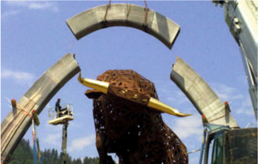
Figure 5 Mounting of aluminium-cast arch segments
