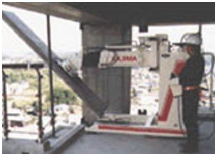
Figure 3 The KAJIMA “Mighty Hand” panel-holding construction robot
