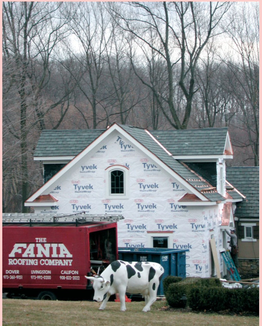
A Tyvek-wrapped house in New Jersey.
