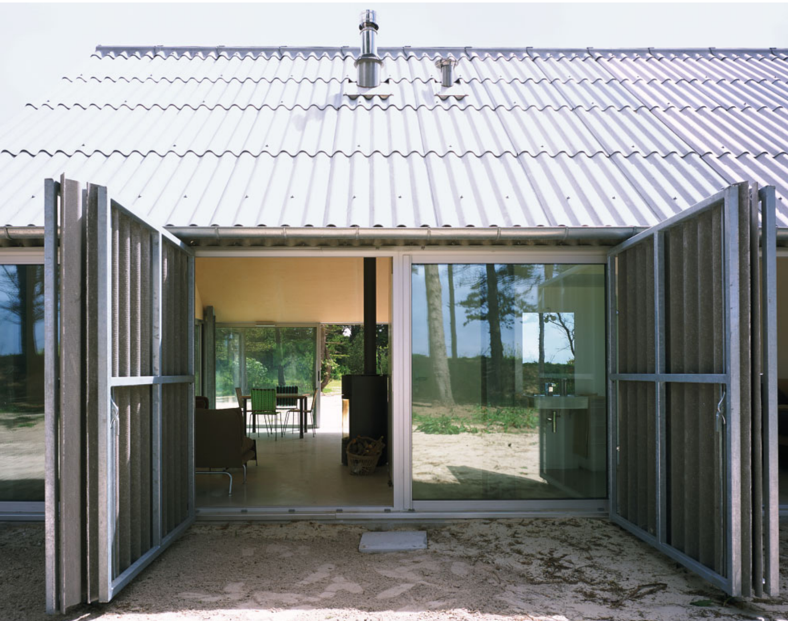
Lacaton Vassal, House in Keremma, Brittany, France, 2005
