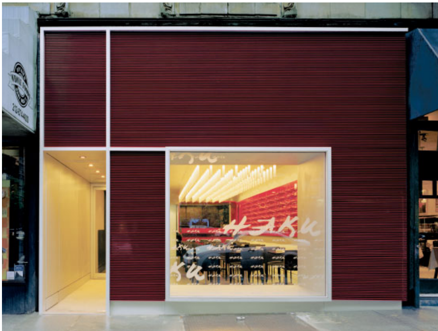
Exterior store-front elevation of Haku restaurant showing powder-coated red, custom-extruded aluminium profiles surrounding a large showcase window. Theatrical interior surface effects are exposed as an urban spectacle for all to see.
