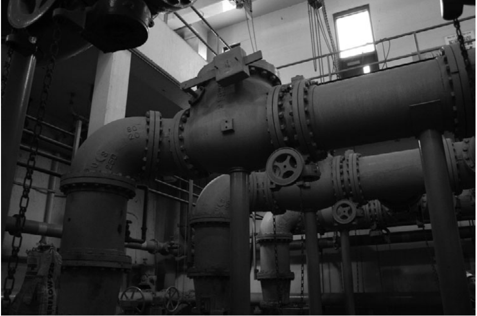
Figure 8-11. Swing check valve installed in a wastewater treatment plant.
