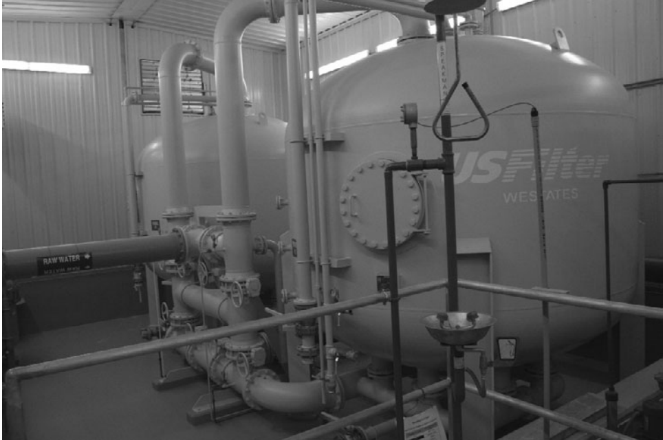
Figure 7-1. Closed-vessel ion-exchange process.
