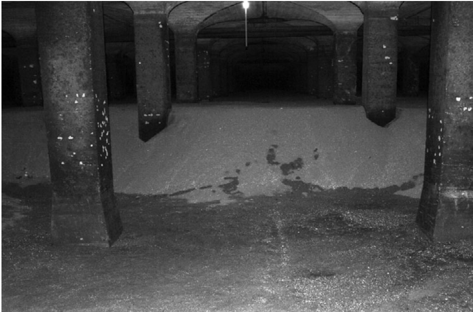
Figure 7-2. Slow sand filter, open-vessel filter process. Above the media is open to atmospheric pressure.
