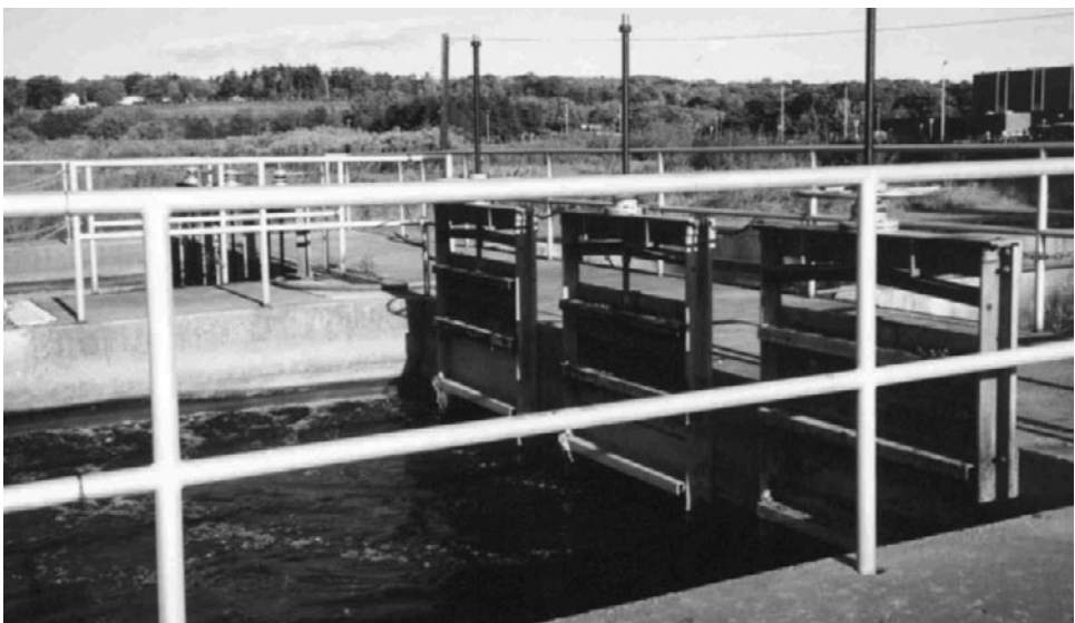
Figure 1-7. Wastewater flowing through open channels to gates.
