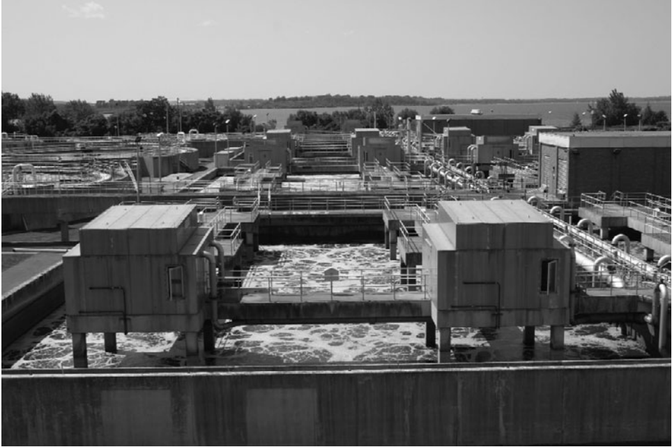
Figure 1-4. Activated sludge aeration tank in a domestic wastewater treatment facility.
