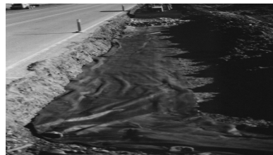
Figure 10. Backfilling on Geotextile
