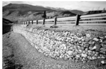
Figure 8. Completed Gabion Wall
