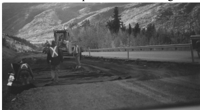
Figure 9. Laying of Geotextile
