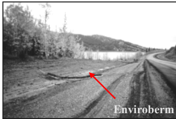
Figure 12 Enviroberm in Ditch
