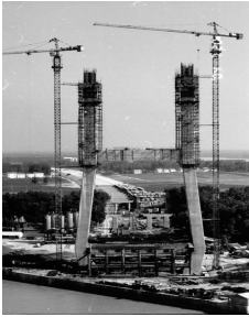
Fig. 4 Main pylon Construction
