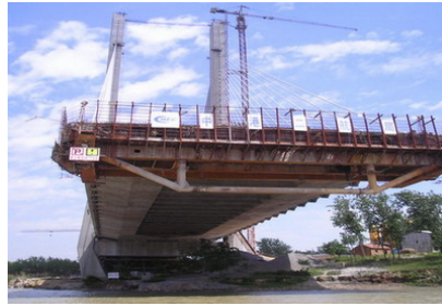
Fig. 5 Balanced cantilever construction
