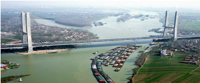
Fig.6 The Completed Wuhekou Cable-stayed Bridge
