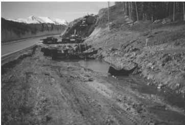
Figure 11. Silt Fence in Ditch
