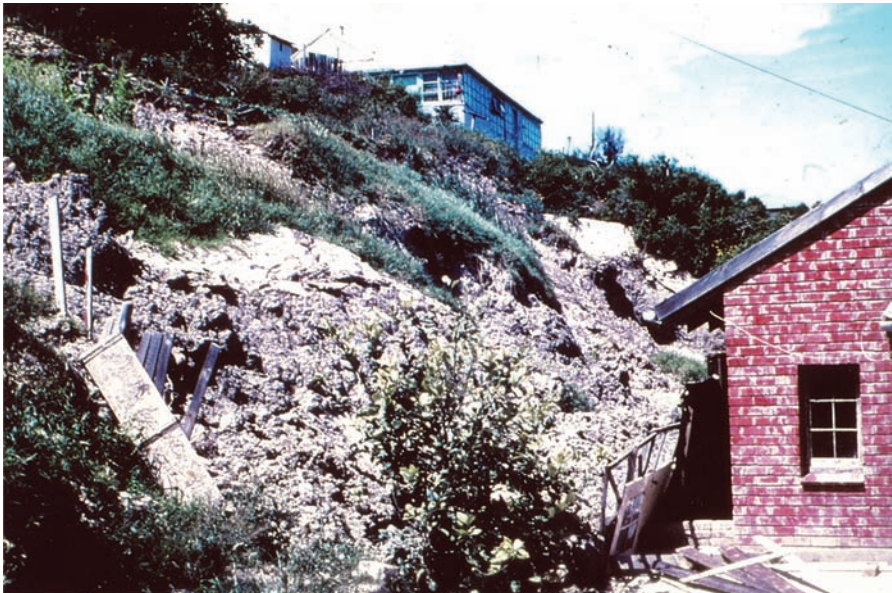
C.28 One of a series of recurrent slides in slope of residual mudstone.
