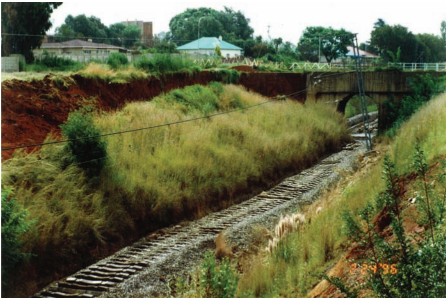
C.30 Slide in 65 year old cut in residual andesite lava.
