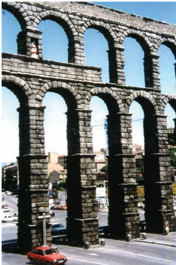
C.22 Roman aqueduct in Toledo, Spain showing little sign of weathering after 2000 years of exposure.
