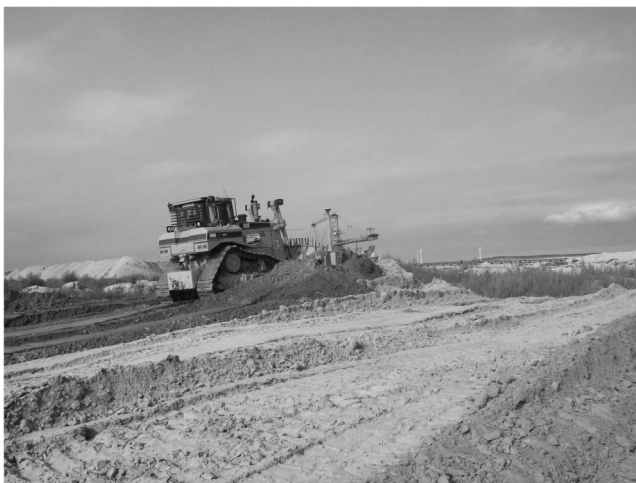
Figure 5 Levelling of stockpiled topsoil during the reclamation of a mine in Eastern Germany. The weight of machinery and degradation of the soil in the stockpile presents challenges to physical conditions for crop production if land is returned to agricultural production.
