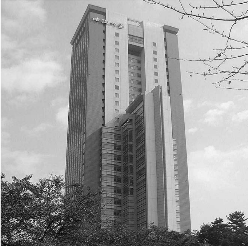
Figure 5.2 Boissonnade Tower on the Ichigaya Campus, Tokyo
