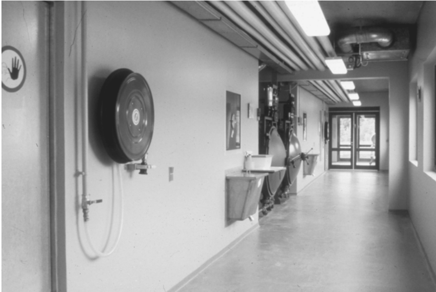
Figure 11.6 The outside of two separated barrier units. The shower entrance of barrier 1 is closest followed by a diptank for chemical disinfection into barrier 1, autoclave for barrier 1, autoclave for barrier 2, diptank for barrier 1, shower entrance and chemical disinfection lock for barrier 2 (M&B Ltd, Denmark).
