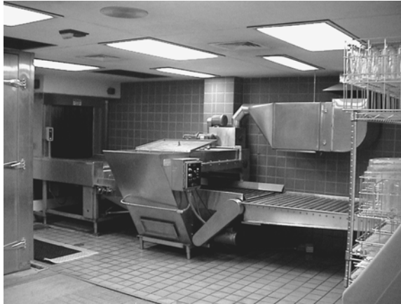
Figure 8.23 In the center of this figure is a bedding dispenser at the discharge end of a tunnel washer. As cages exit the tunnel washer (top left) open side down, they are automatically turned over, as they tumble onto the lower bedding dispenser belt so the open side of the cage is up. Upon exiting the bedding dispenser, the cages collect on the roller conveyor to the right of the dispenser. Above and to the right of the dispenser is a vacuum cleaner that collects bedding dust generated by the dispenser. Note the ceramic tile floor and wall coverings with epoxy grout and a corner of a grate-covered floor pit at the bottom left of the figure in front of the rack washer.
