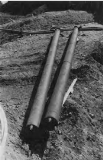
Figure 12-5b Jetting Casings.
