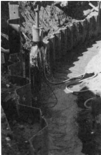
Figure 12-5c Driving the Jetting Nozzles.
