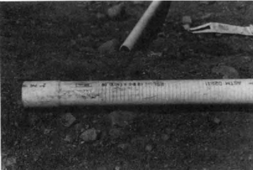
Figure 12-5a Filtering Pipes Used in Dewatering Process.
