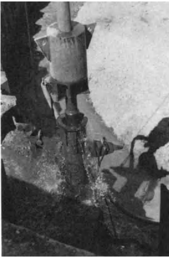
Figure 12-5d Withdrawing the Jetting Nozzles.
