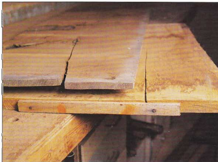
LEFT: End-grain, split and nailed
