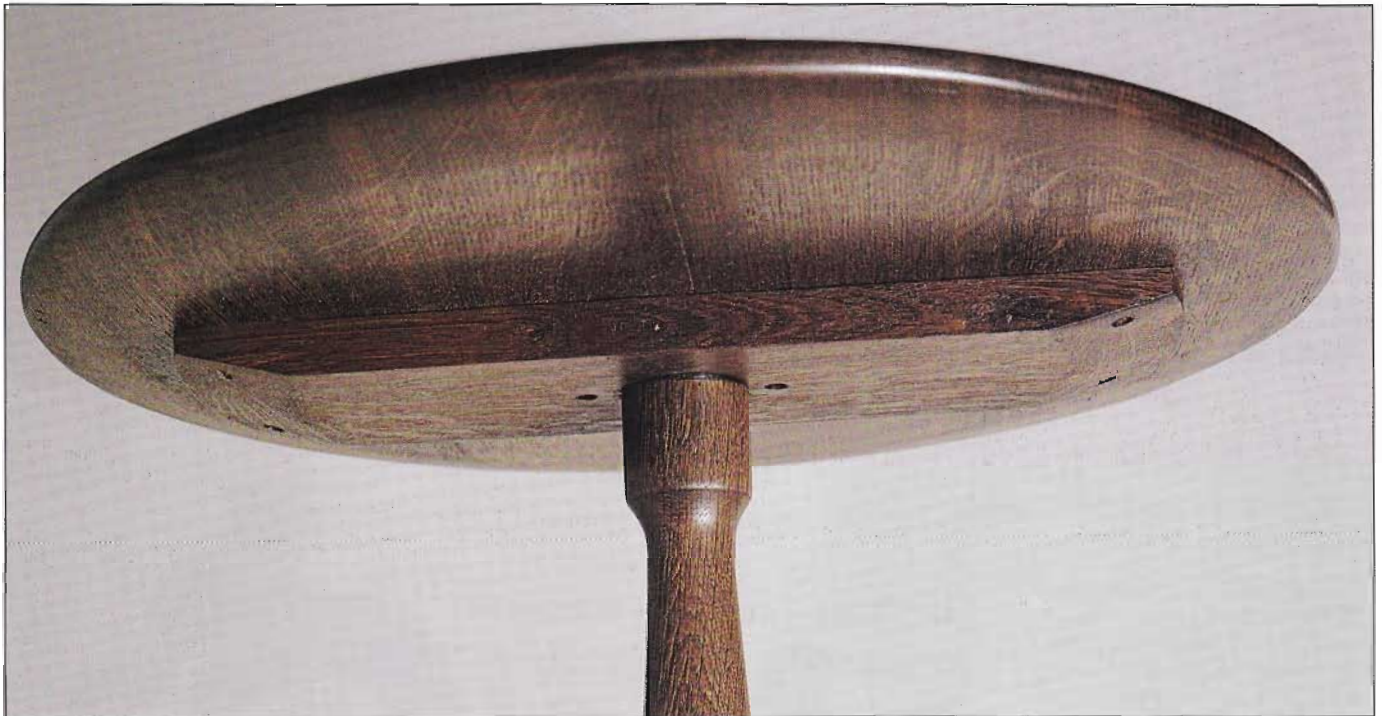
TOP: Underside of table showing brace connecting the column to the top
