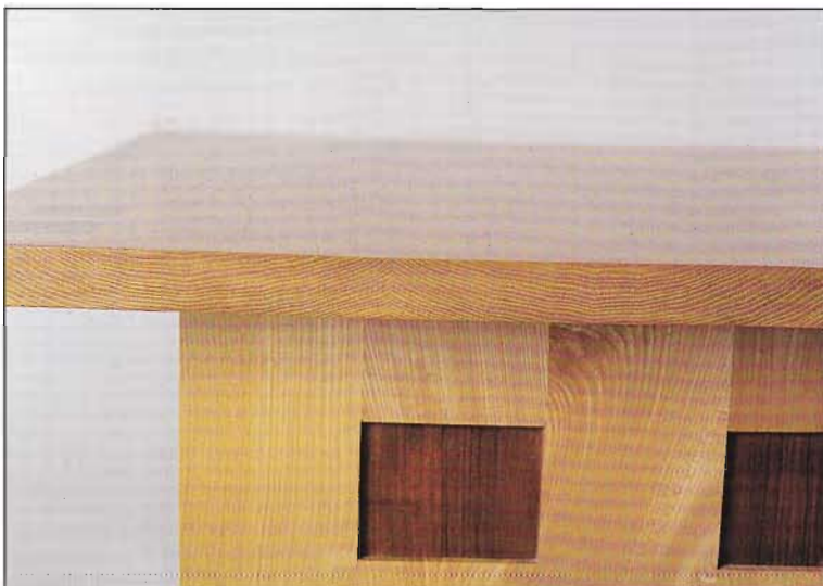
ABOVE: Tangentially-sawn elm end-grain table top — wrong
