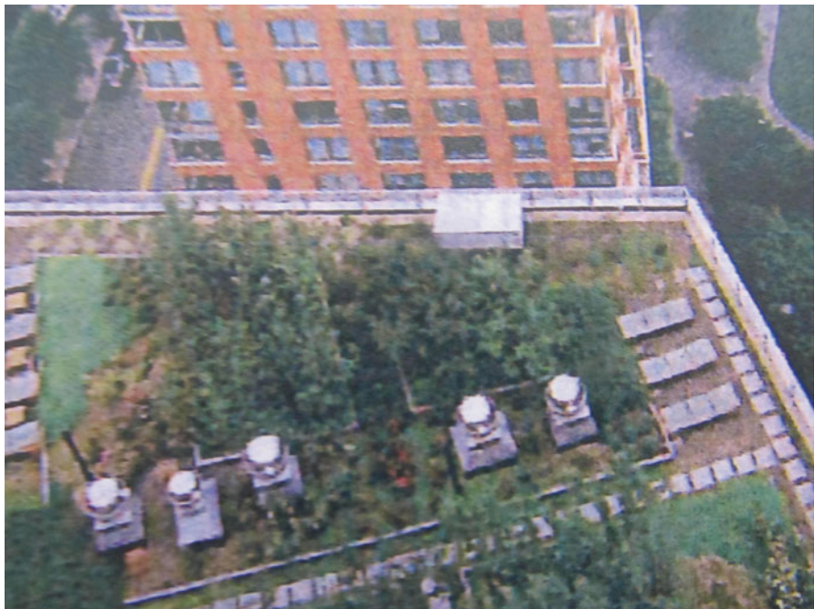
Plate 2.12 Roof top gardens and solar installation. Location: Battery Park City, Manhattan (Source: The Green Building Handbook (2010). New York City Economic Development Corporation)
