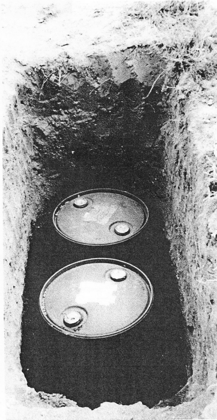
Septic barrels when first placed in holes.
