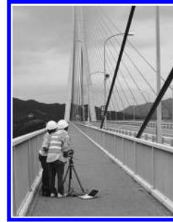
Figure 3. Application to tensile force measurement of cables.
