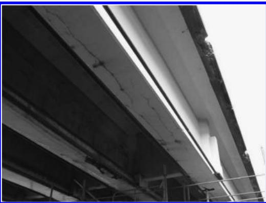
Figure 1. Cracks at the lower-flange of the girders occurred along the bridge axis.
