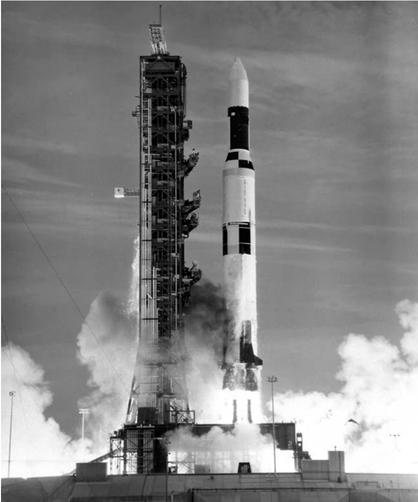
16. Skylab was launched as the third stage of a modified Saturn v rocket.
