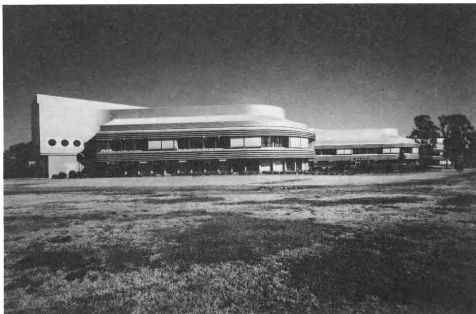
Fig. 4 Mt. Druitt Hospital, NSW: north-east elevation showing horizontal solar control (photo by Max Dupain)
