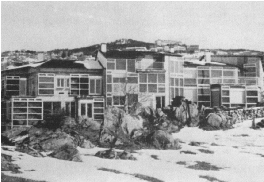
Fig. 4.43. Trombe wall house at Odeillo.
