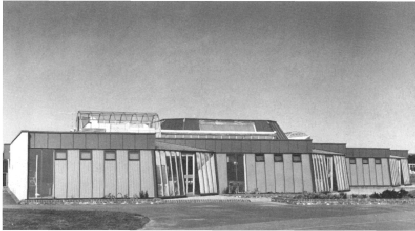
Fig. 13.8. St John's School, Clacton on Sea, Essex. (a) Exterior. (b) Plan. (c) Schematic of energy systems. (Courtesy of Essex County Council.)
