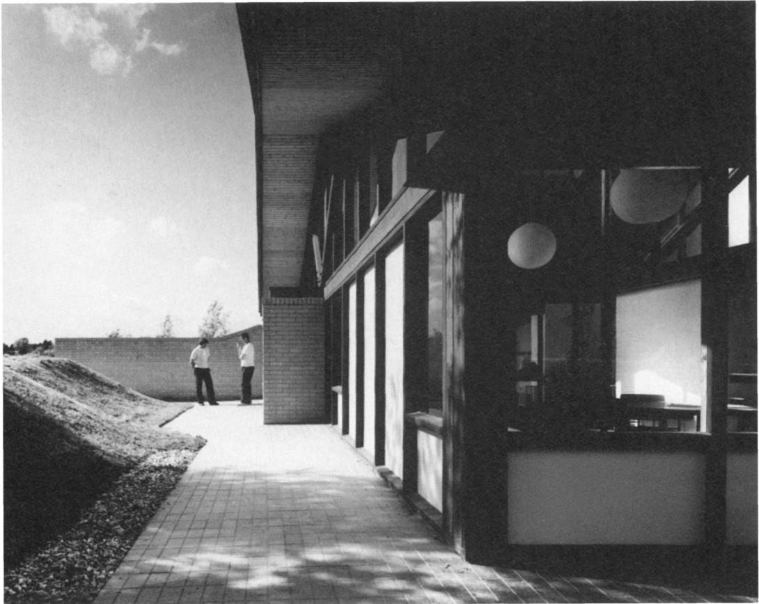
Fig. 13.7. Yateley Newlands School, Hampshire. (a) Exterior. (b) Plan. (c) Conservatory. (Courtesy of R. Bryant and The Architects Journal .)
