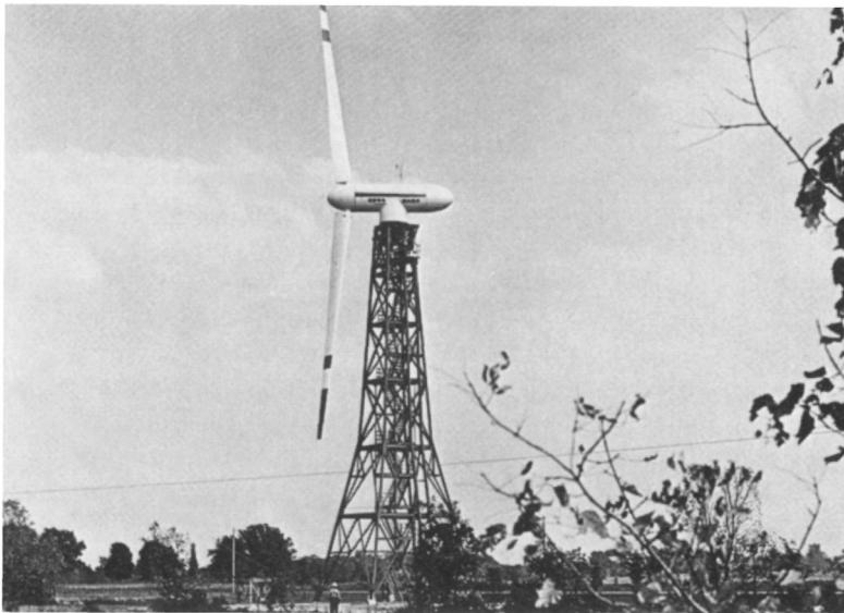
Fig. 8.14. ERDA/NASA 100 kW wind turbine at Plum Brook, near Cleveland, Ohio.
