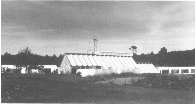
Fig. 4.4. Kalwall glazing to the 'Ark' on Prince Edward Island. (Courtesy of Kalwall Corporation, Manchester, New Hampshire.)
