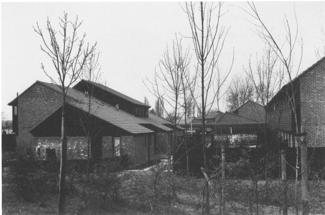
Fig. 2.7. View of Basildon Northlands 1 Housing showing insolation of south facades over lower buildings. [21] (Courtesy of Antoine Rafaul.)
