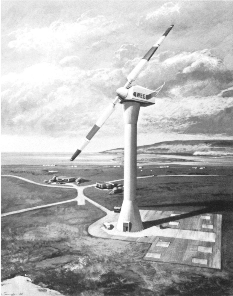
Fig. 8.1. 60 m diameter, 3 MW turbine to be built on Burger Hill, Orkney, by the Wind Energy Group (a joint venture of Taylor Woodrow Construction, GEC Power Engineering and British Aerospace).
