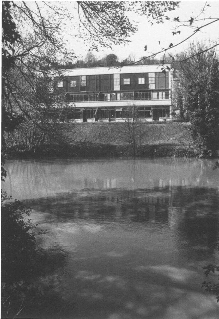
Fig. 4.49. Low cost maisonettes in Bath using mass walls with selective surfaces (designed by Feilden Clegg Associates).
