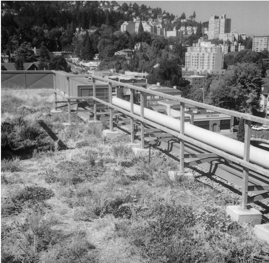
Fig. 22.1 Green roof, Portland, Oregon
