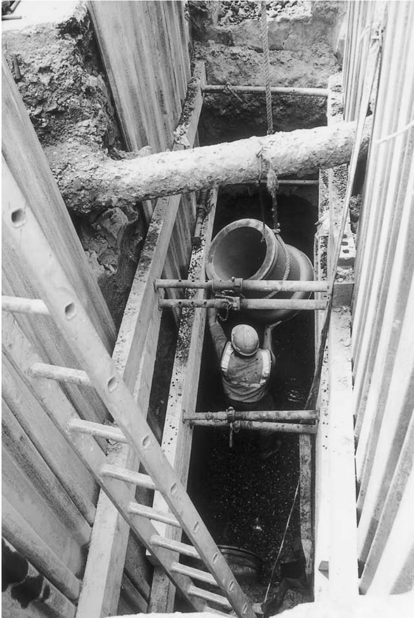
Fig. 16.1 Open-trench construction (courtesy of Clay Pipe Development Association)
