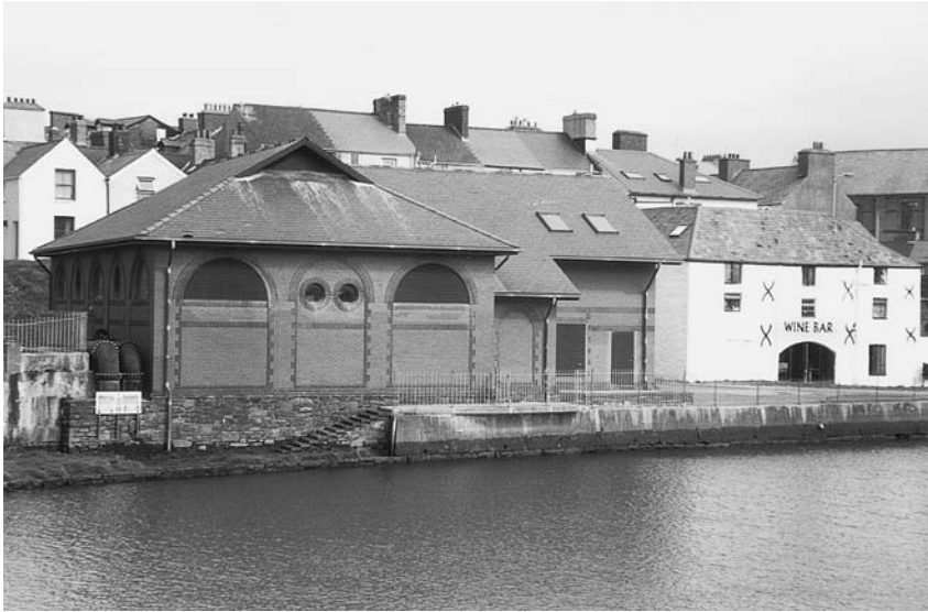
Fig. 15.11 Pumping station: architectural treatment
