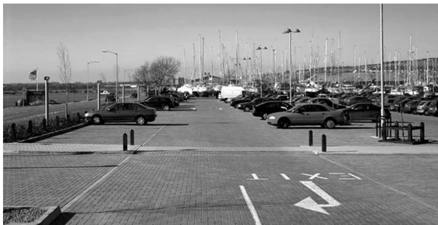
Fig. 22.5 Car park with pervious pavement (courtesy of Formpave Limited)
