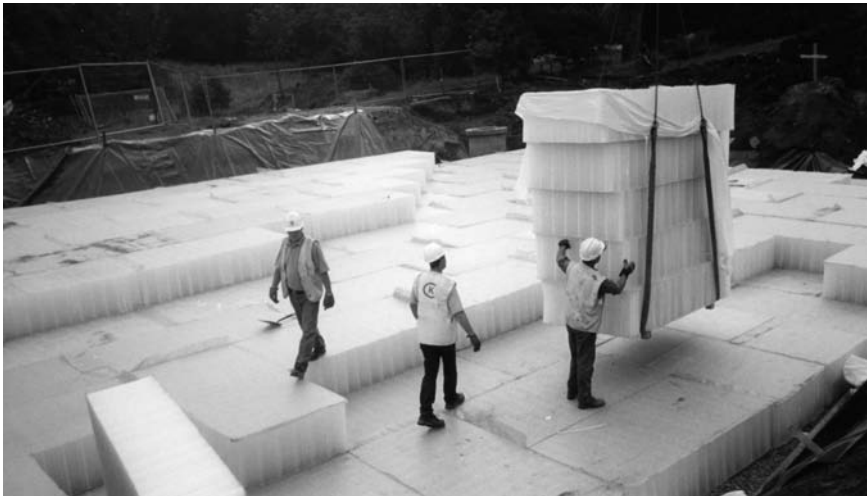
Fig. 14.2 Installation of a Stormcell® storage device (courtesy of Hydro International)
