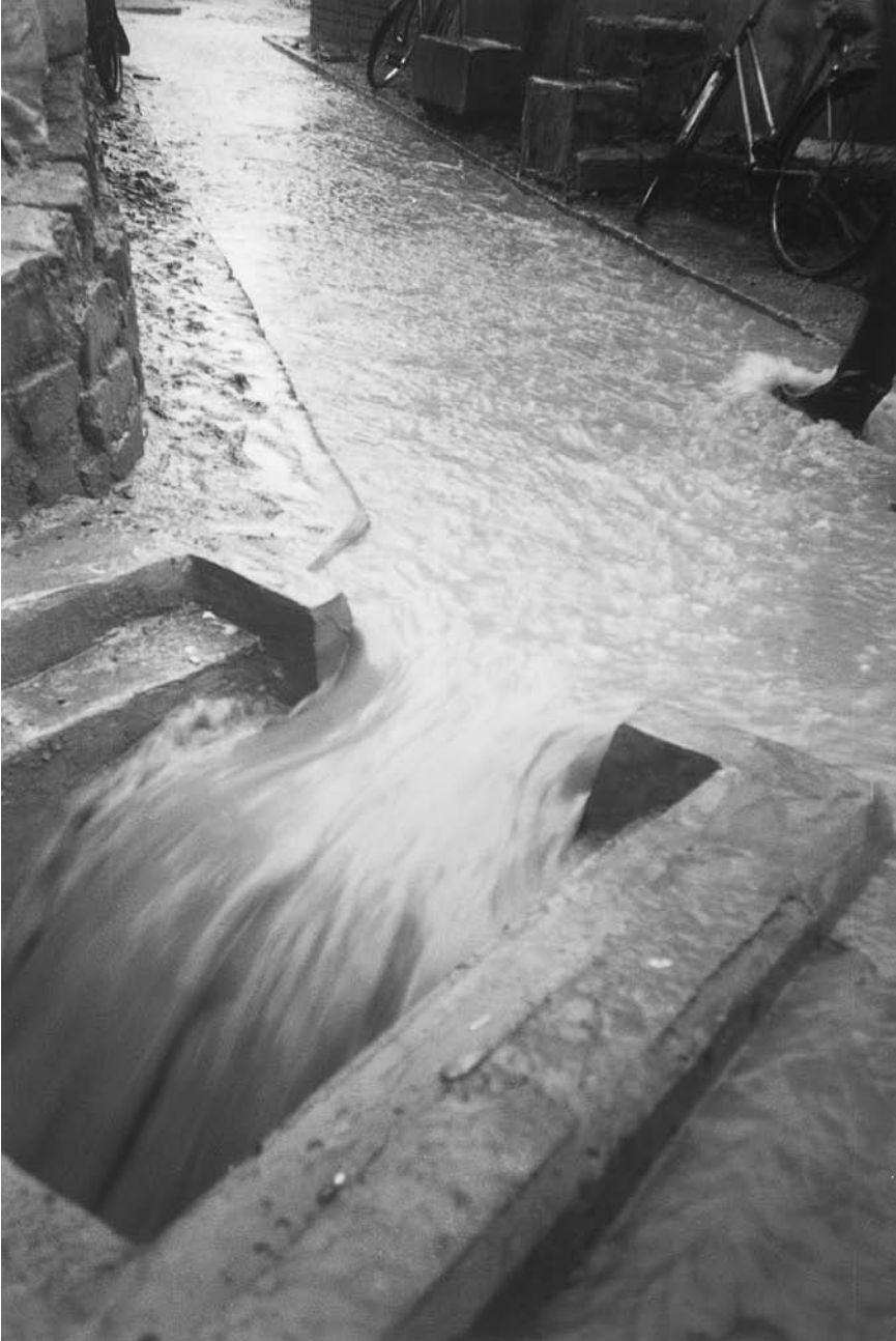
Fig. 23.7 Road-as-drain in Indore, India
