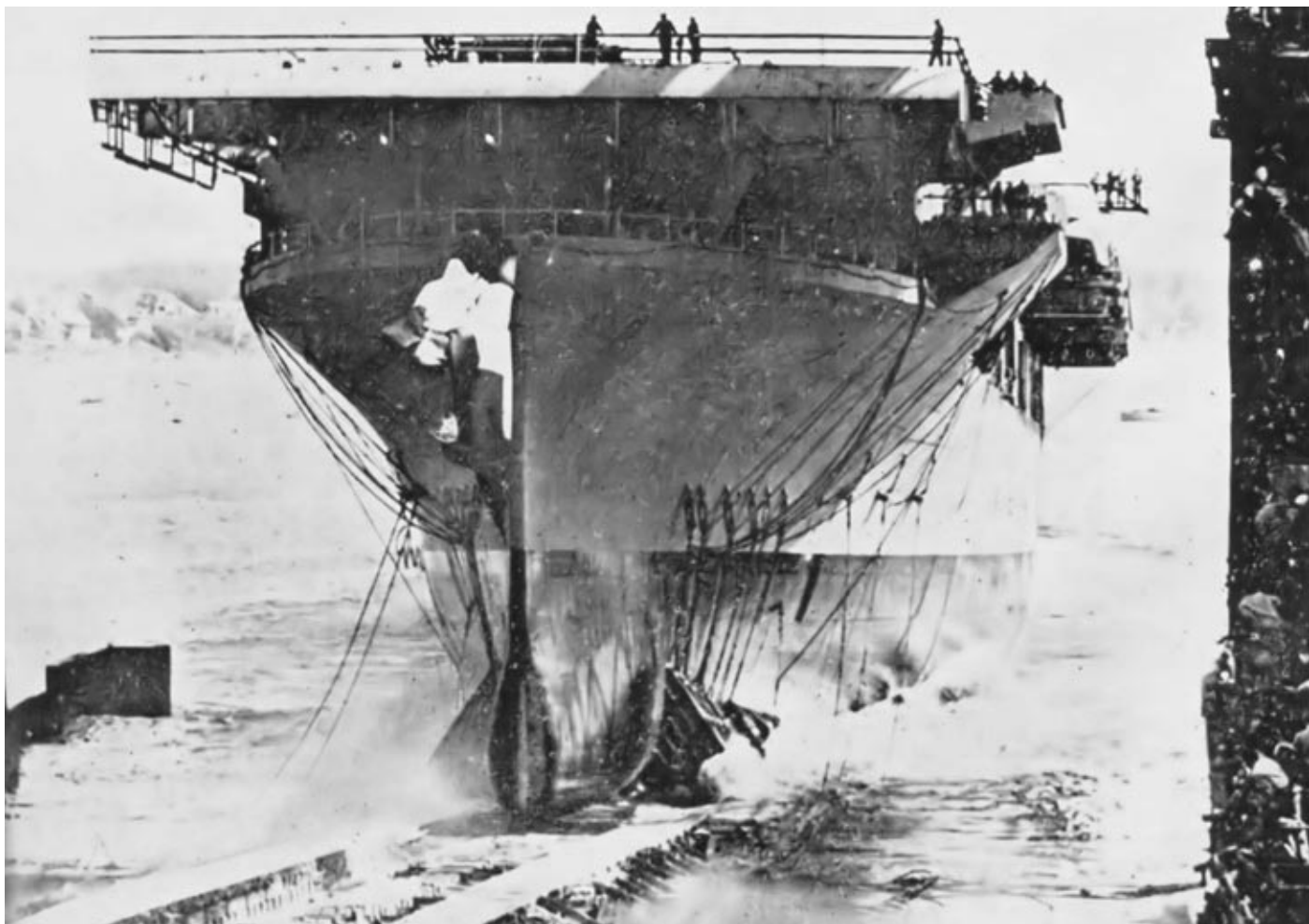
A new aircraft carrier slides into the water. Built and launched in the US Navy yard of the Bethlehem Steel Company, Massachusetts, this emergency-built carrier was one of many built during the war years.
