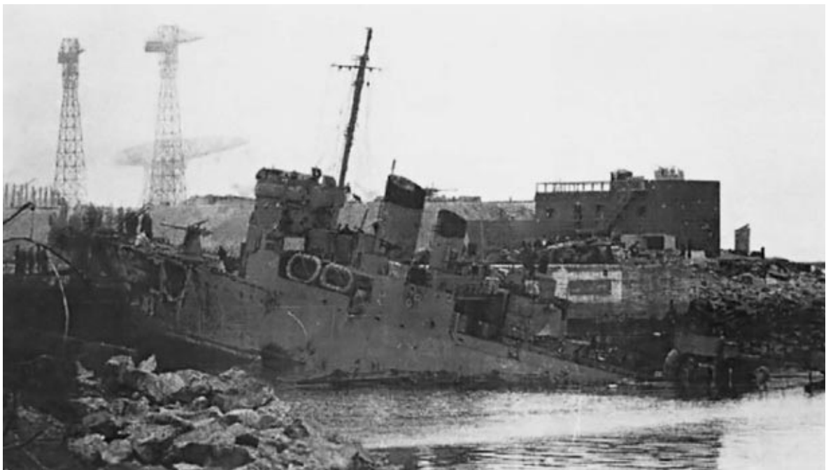
On 28 March, the British launched a raid on the dock at Saint-Nazaire. An old four-stacker, Campbeltown , was adapted (losing two of her funnels) and driven into the dock gates. Sometime after the raid had finished, explosives on the ship were detonated and serious damage was caused.
