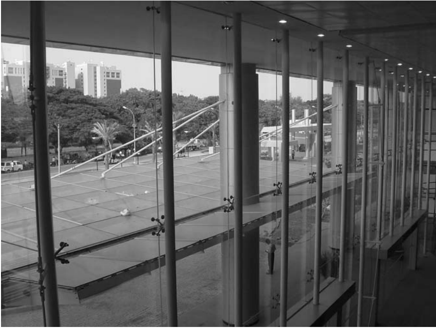
Figure 6.9 Glass interior of Ascendas IT Park—Chennai.
