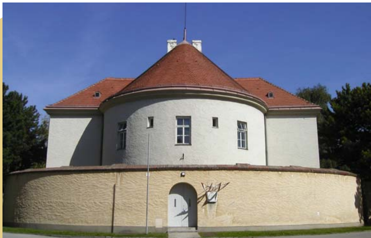
Former pump room of Neugebäude Palace, now the crematorium administration.
