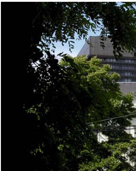
Former administration building behind.
