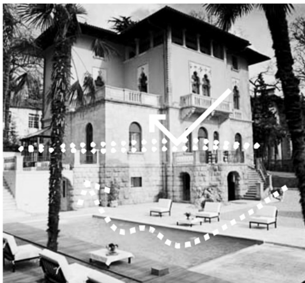
Figure 3. Villa with the swimming pool, cooling measures
