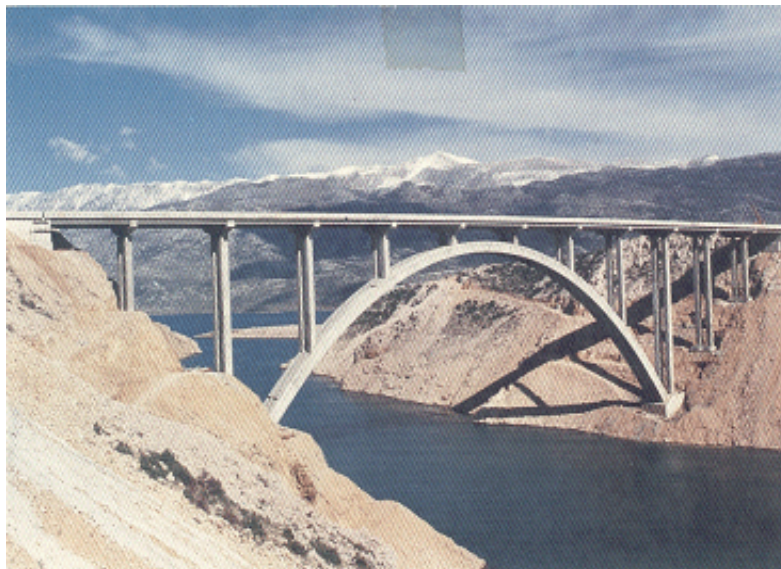
Figure 1. Panoramic view of the Maslenica bridge.
