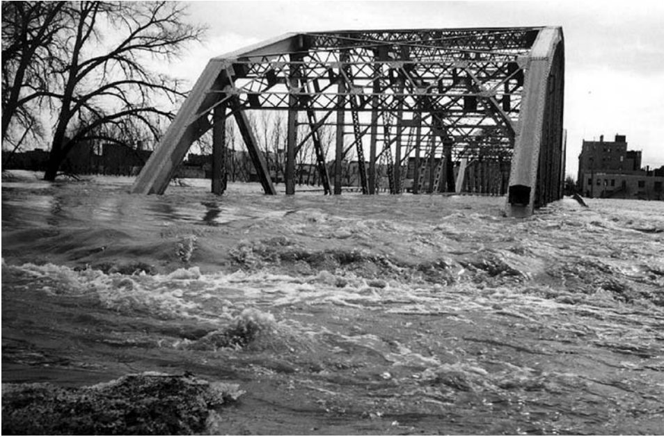
Flood water covering the Sorlie Bridge, Grand Forks, North Dakota, during the Red River Flood of 1997. (U.S. Geological Survey)
