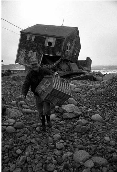
Coastal home in Scituate, Massachusetts, destroyed by a 1991 Nor'easter storm; the owner is recovering the remains of his home. (AP/Wide World Photos)
