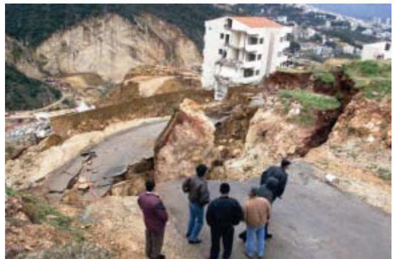
■ FIGURE 15.25 Landslides not only modify the landscape but also can cause much destruction when buildings are constructed in areas susceptible to mass movements.
