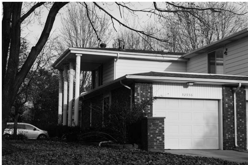
Fig. 5.4 Newer and larger houses in North Warren, also facing foreclosure
