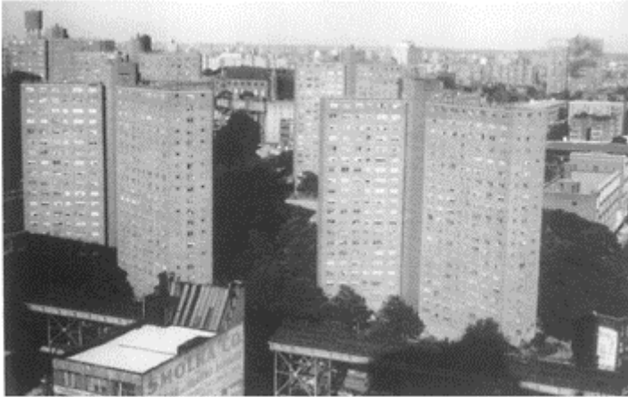
c Public housing, Harlem, New York. Such housing partially replaces nineteenth and early twentieth-century tenements, many very run down, some undergoing gentrification
