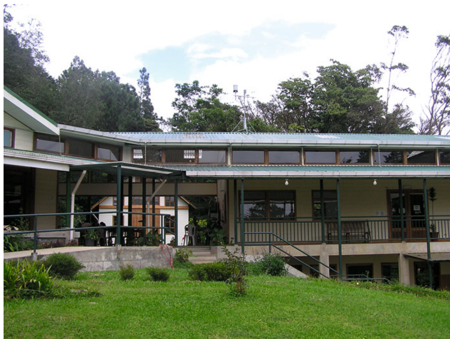
Main offices and entrance of the Monteverde Institute, village of Monteverde. Photo by N. Blum
