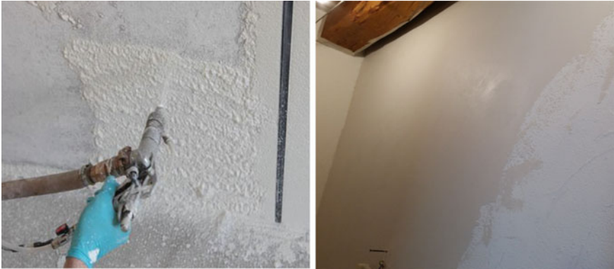
Fig. 2.6 In situ application of the aerogel-based plaster (courtesy of Agosti Fabrizio, Agosti Nanotherm s.r.l., Naturalcalk-Tillica 2015)
