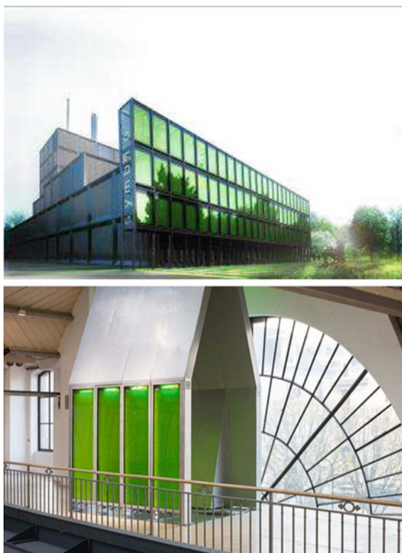
Fig. 17.3 Biofaçade in a waste processing plant in Nantes and the L'Algo-Nomad Pavilion, with 4 PBRs in one façade
