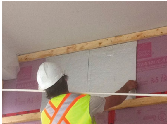
Fig. 7.14 Installation of VIPs with adhesives (MacLean et al. 2011)
