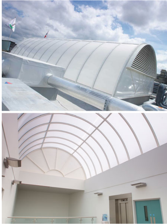
Fig. 3.10 Application of aerogel in skylight systems (16 mm clear polycarbonate with Lumira Aerogel): Lafarge Cement Reception hall, UK (Courtesy of Roda—EMB, Germany)
