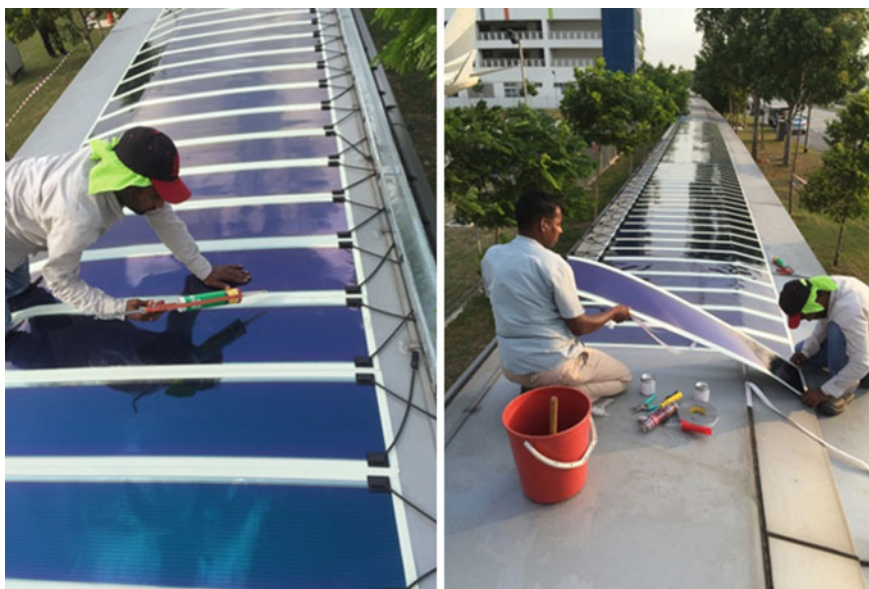
Fig. 11.16 Installation of Heliafilm on the Seletar walkway (courtesy of Heliatek)
