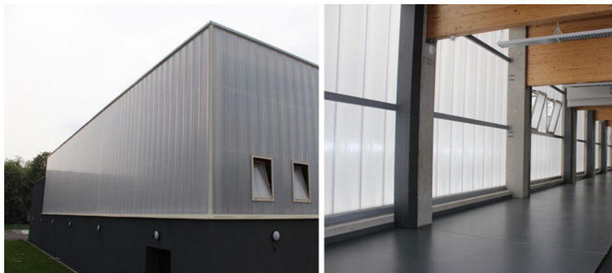
Fig. 3.8 Example of the application of Lumira ® aerogel in polycarbonate sheets (Gymnasium at BBS Mainz, outside and inside view of the building. Courtesy of Roda—EMB, Germany)
