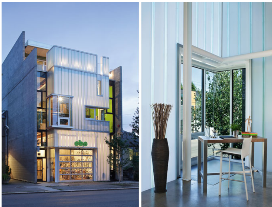
Fig. 3.9 Example of the application of aerogel in polycarbonate sheets in a multifunctional building in Seattle, Washington's Fremont District, Building 115 © William Wright Photography. Image courtesy of Technical Glass Products
