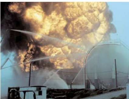
Example of a LPG sphere that required heavy cooling during a nearby tank fire.
