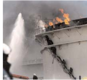
Attack of a rimseal fire from stairway—see how much manpower is needed to deploy flexible hoses when there is no fixed dry risers.
