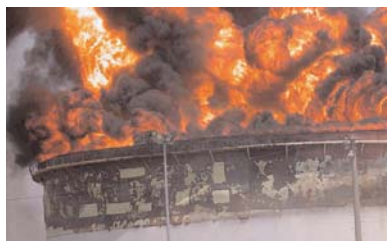
Fire once the roof lost buoyancy
