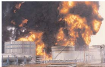
e. Three tanks fully involved
