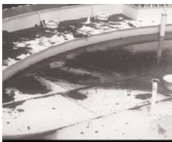
Example of a roof with waxy deposits
