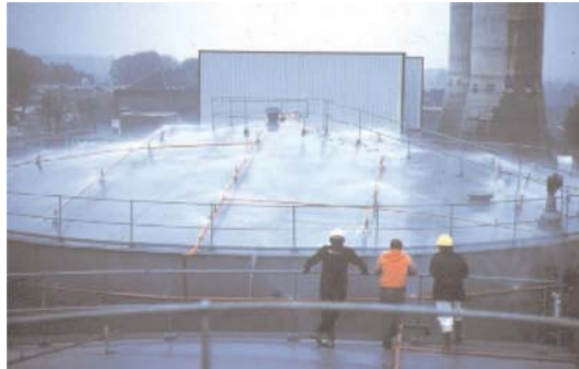
Tank shell and roof waterspray tests
