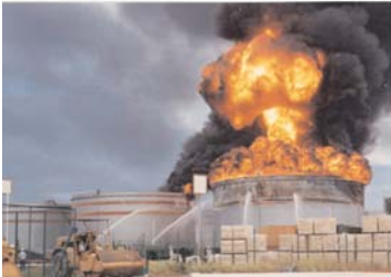
c. Adjacent tank beginning to burn
