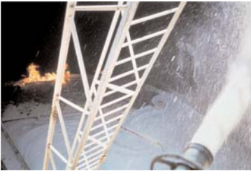
Example of a seal fire being attacked from the gaugers platform with a hand-held foam monitor.
