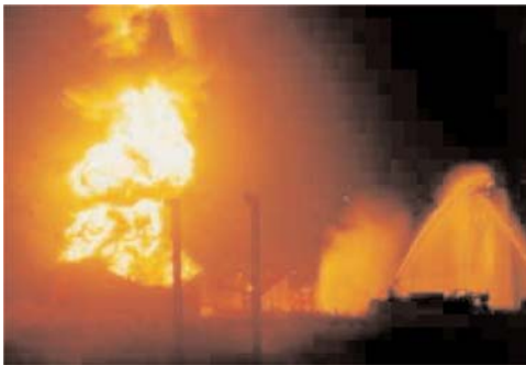
Example of cooling adjacent tanks with mobile equipment
