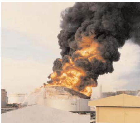
Typical example of cooling water effect when applied only to one side. The non cooled side is folding and the shell is subjected to extreme stress.
