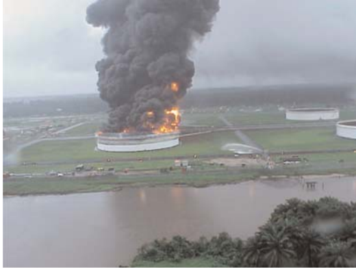
This crude tank fire could not be extinguished due to lack of resources. Despite boilovers occurring, adjacent tanks were unharmed, due to a sound design that included large tank spacing.
