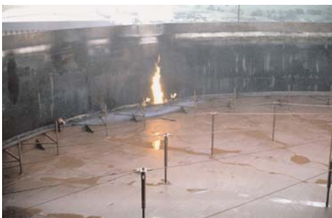
Rimseal fire at an early stage
