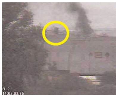
Early stage of the rimseal fire as captured by security camera. Note flying pontoon plate in yellow circle
