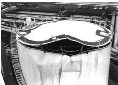
Another incident where a storage tank fails at shell-to-roof seam (fish mouth) due to overpressure.
