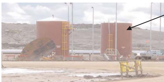
Tank after roof blew off.
