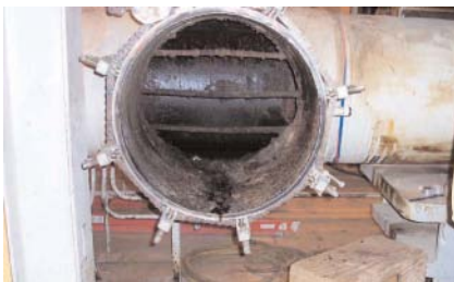
View of the 28 inch (71 cm) pipe
