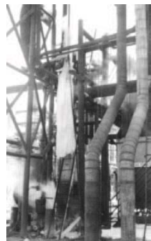
Figure 21b Ice from steam traps.
