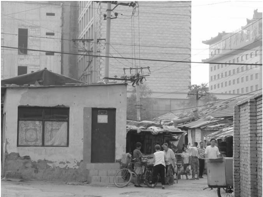
4. Half-destroyed inner city neighborhood in Beijing (August 2004)
