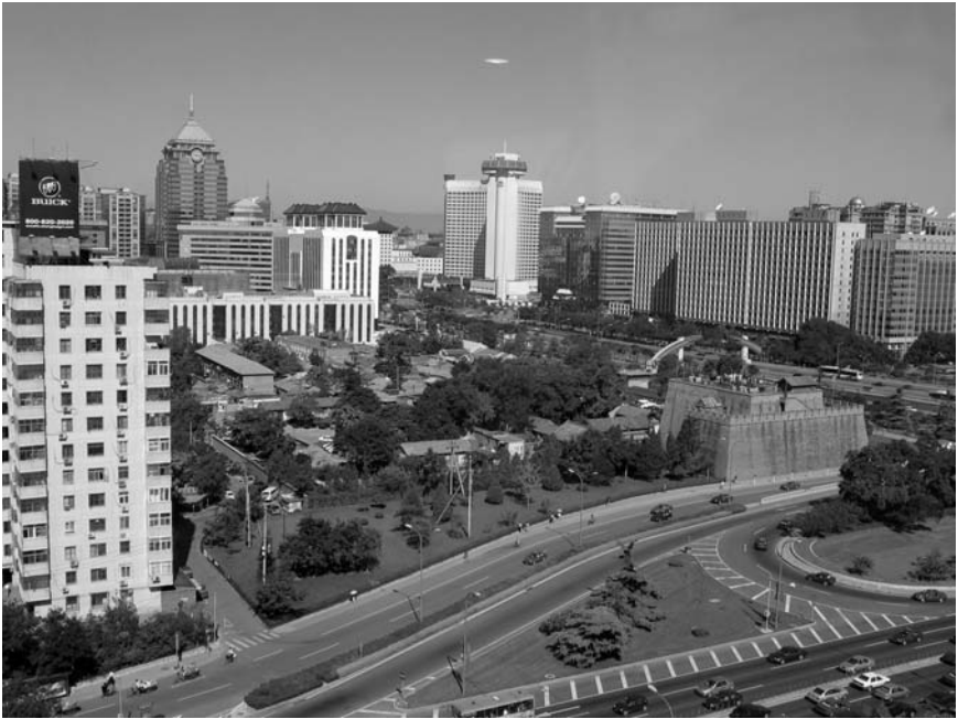
1. Traditional courtyard housing encroached by new buildings in inner city Beijing (June 2004)
