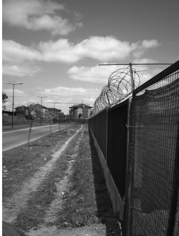
Fig. 3 The barrier of the new Caledonian campus during construction
