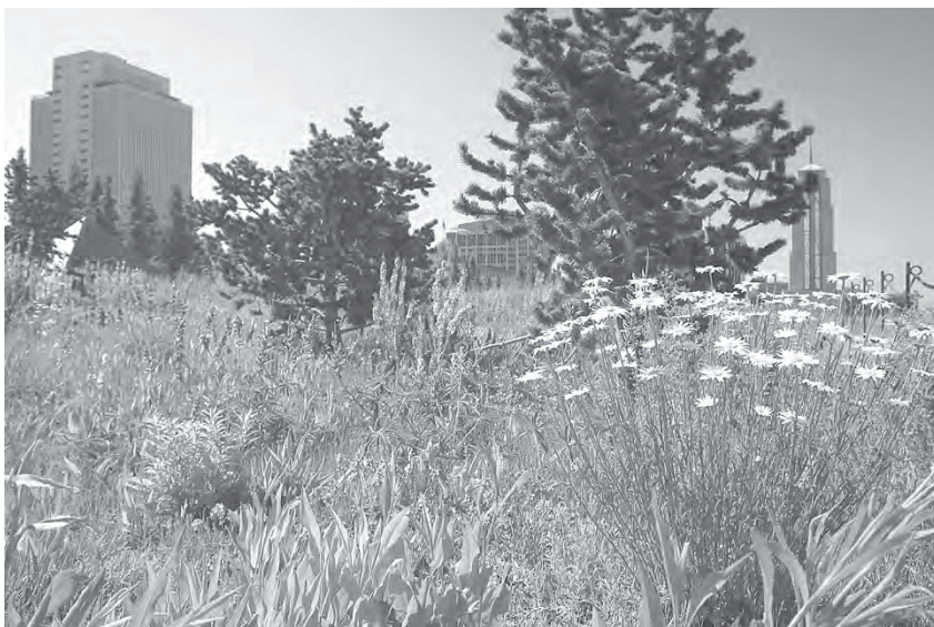
Figure 3.19 The LDS Convention Center in Salt Lake City supports lush "intensive" roof gardens, even forest. (Project: Olin Partnership. Photo: Craig Widmier.)
