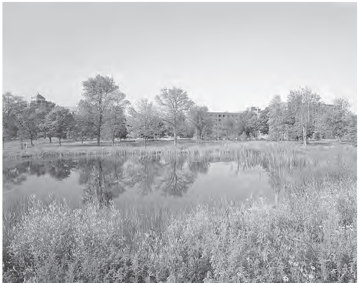
Figure 4.8a–c This constructed wetland was (a) carefully excavated to specific depths required by wetland plants, then (b) lined. Planted with marsh-tolerant sedges (c), the completed wetland treats graywater organically for reuse, reducing this Michigan convent’s water use by half. (See p. 239 for project description.) ( Project and Photo: Veridian Landscape Studio. )
