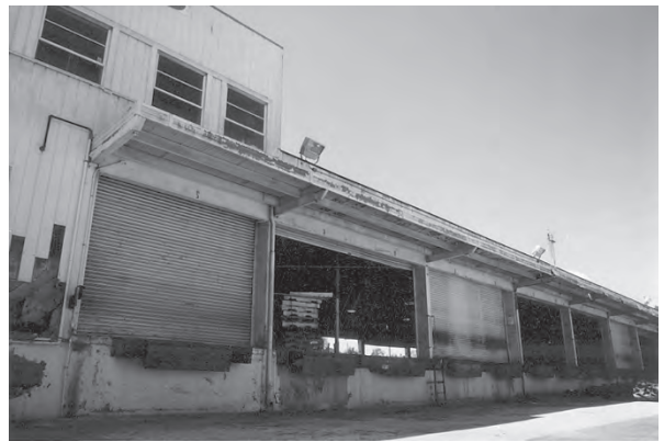
Figure 6.6 This unpromising site was reborn as a garden for Monnens Addis Studio—without major demolition. (Photo: Jeffrey Miller.)
