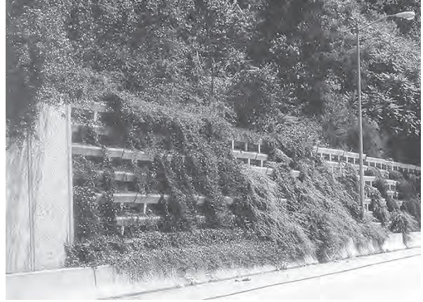
Figure 3.9 The Evergreen “trough” greenwall serves both as retaining wall and as noise wall on Philadelphia's Blue Route (I-476). (Project and Photo: Synterra Ltd.)
