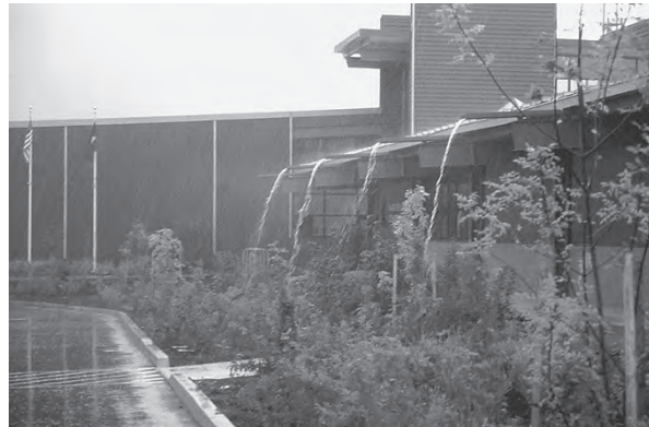
Figure 4.23 Collected on the Portland Water Pollution Control Lab’s roof, water spouts from scuppers in rhythmic jets. (Project: Robert Murase. Photo: Tom Liptan.)
