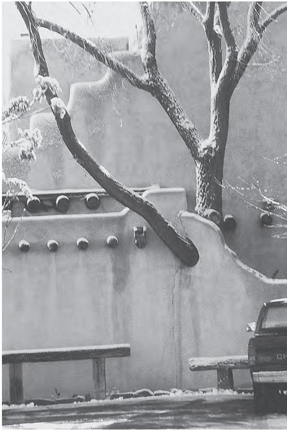
Figure 6.10 Adobe is one of the most flexible materials to work with, and inspires site-specific construction that celebrates existing features like this tree. (Photo: Kim Sorvig.)
