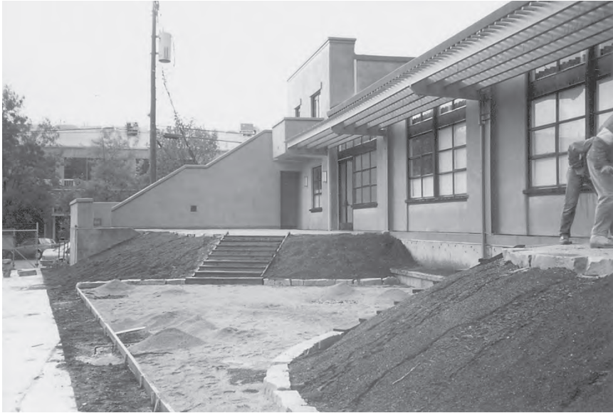
Figure 6.7 The Monnens Addis renovation in progress. (Project: Miller Co. Photo: Jeffrey Miller.)
