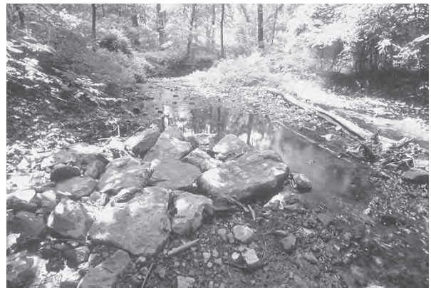
Figure 4.13 Stone deflector in restored Wheaton Branch unobtrusively guards the stream bank from floods. (Project: Washington Council of Governments. Photo: Walt Callahan.)
