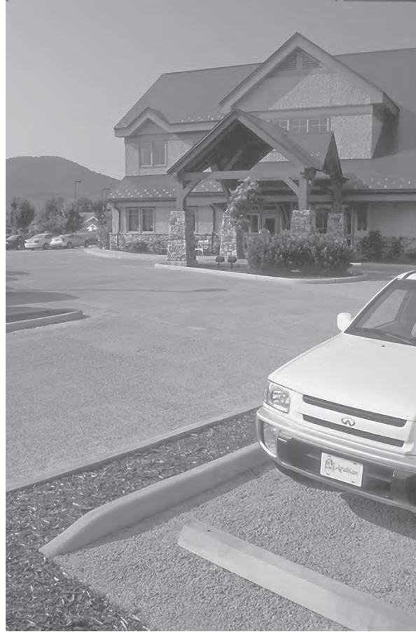
Figure 5.6 Porous parking is separated from standard driving lanes. This stormwater management tactic can also create strong aesthetics. (Project: Spaceplan [arch.]; Petrus [pervious paving]. Photo: Bruce Ferguson.)
