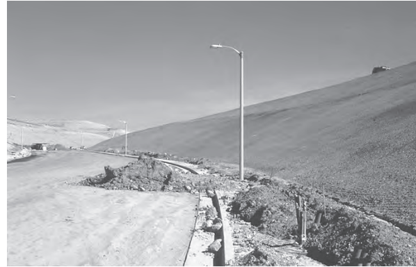
Figure 2.9 Conventional grading insists on uniform, planar slopes. Until recently, objections to this approach have been aesthetic, but recent research shows environmental disadvantages, too. (Photo: H. J. Schor.)
