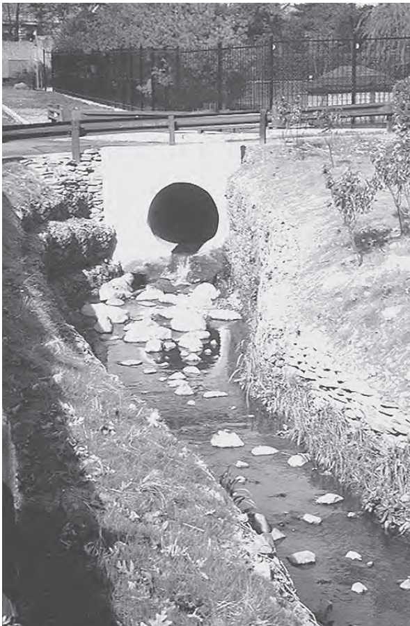
Figure 4.17 Maguire Avenue after installation of gabions, boulders to deflect culvert outflow, and plantings. (Project: New York City Department of Environmental Protection. Photo: Dean Cavallaro.)
