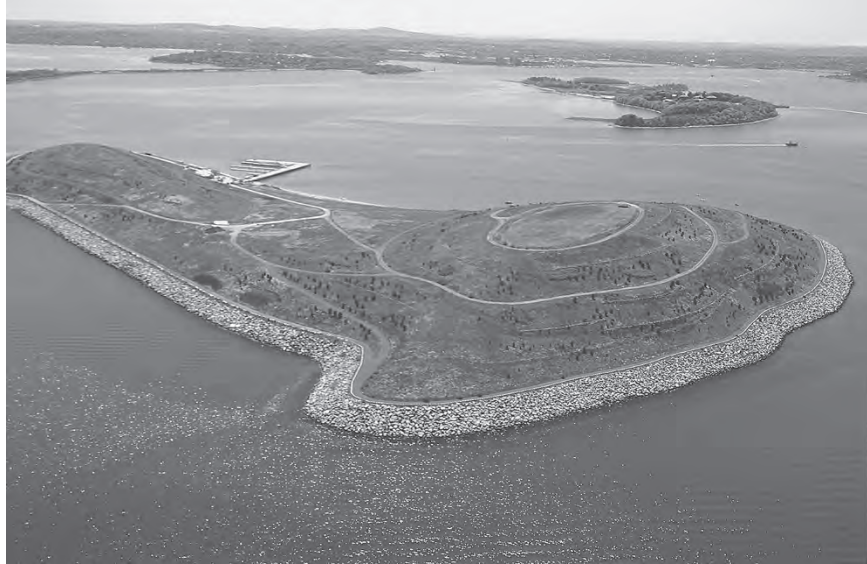
Figure 2.16 Spectacle Island in Boston Harbor is a recreational landscape salvaged from a toxic dump. (Project: P. Craul with Brown and Rowe. Photo: Massachusetts Turnpike Authority.)
