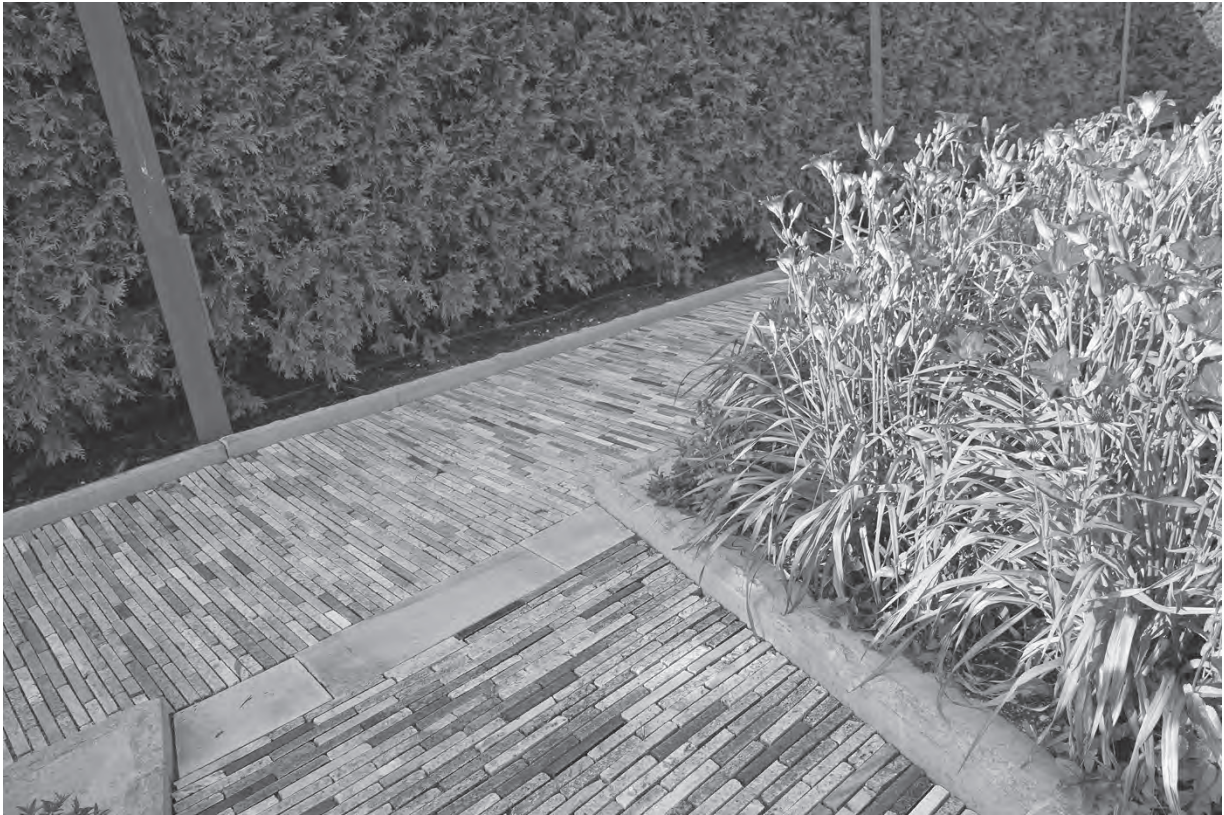
Figure 6.11 Reuse of stone can be monumental (see Parque de la Cidade, Oporto, p. 275, and Malinalco, p. 267) or small-scale. At Millennium Park’s Lurie Garden in Chicago, stone countertop scrap gives textured detail to walkways, recalling similar uses of broken tile in traditional gardens. ( Project: Terry Guen Design Assoc. Photo: Ryan Mikulenska.)
