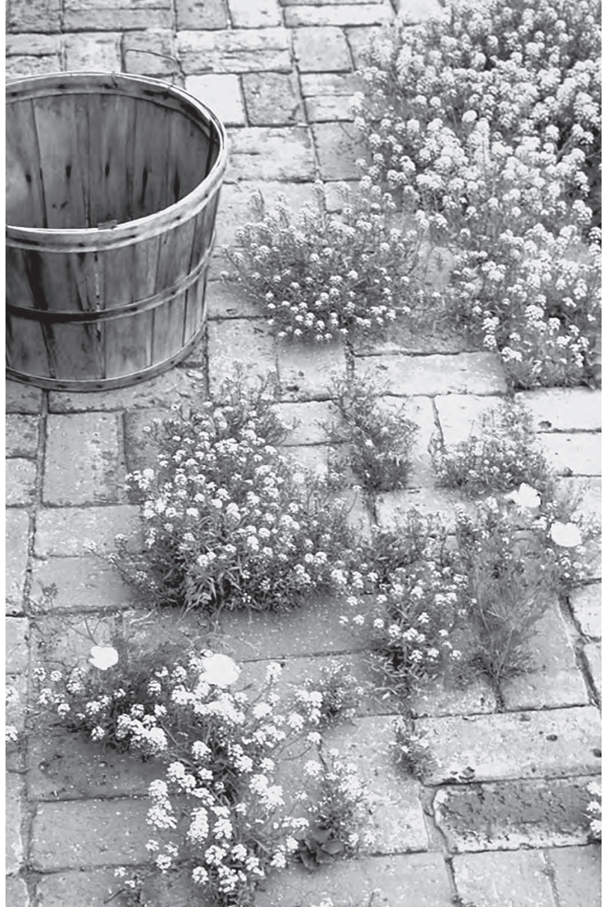
Figure 5.18 In small-scale, low-traffic areas, unit pavers can even support wildflowers. (Project: R. and V. Sorvig, Photo: Kim Sorvig.)
