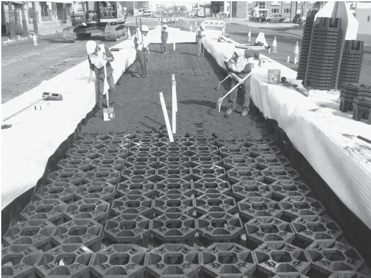
Figure 3.26 “Cells” to support suspended pavement are a relatively recent addition to the toolkit for protecting street trees. Strata Cells, shown here, are designed to stack for efficient shipping (right rear). (Project and Photo: Citygreen.)
