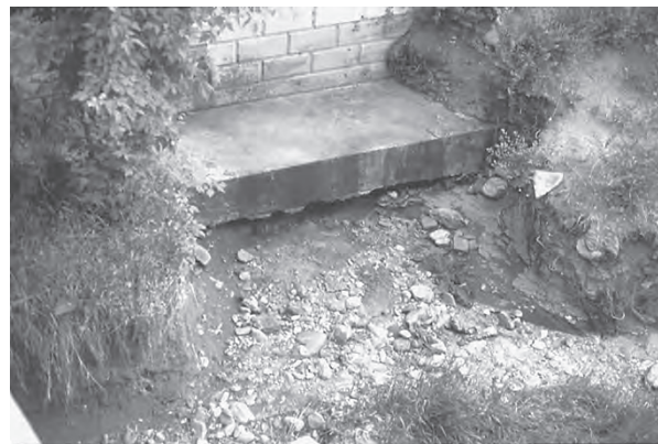
Figure 2.I4 Rigid structures protect only the soil they can shield from water. Along the hard edges, erosive undercutting is actually increased. (Photo: Kim Sorvig.)
