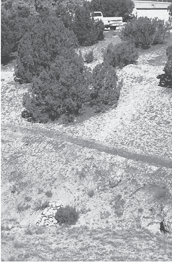
Figure 4.3 Contour-line infiltration trenches, plus check dams in the gully at bottom, stop erosion and raise soil moisture in this Permaculture project in arid New Mexico. (Project: Arina Pittman. Photo: Kim Sorvig.)
