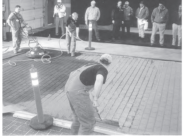
Figure 5.20 Decorative color coatings for asphalt can lighten the surface, decreasing heat-island effects. Integral color, mixed into hot asphalt, is also becoming available. (Photo: StreetPrint, Scott Hind.)
