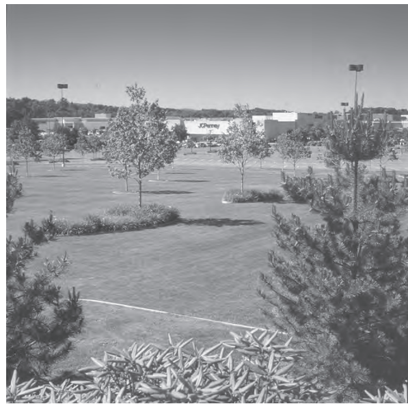
Figure 5.13 Overflow parking at Westfarms Mall uses Gravelpave 2 instead of impervious asphalt. (Photo: Invisible Structures.)
