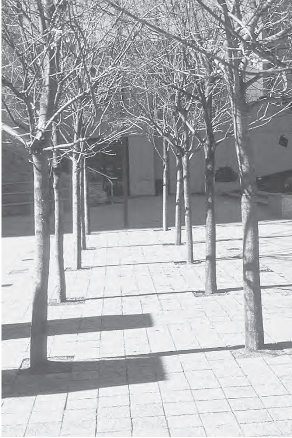
Figure 5.15 Henry Arnold has used open-jointed unit pavers at large plazas in Atlanta GA, Brooklyn NY, and Newport NJ, usually with extra aeration vents. (Project and Photo: Henry Arnold.)
