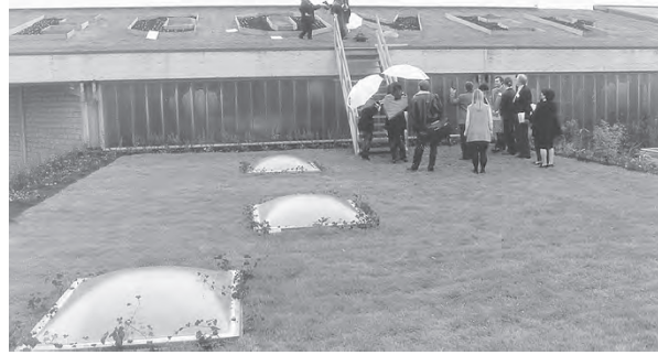
Figure 3.20 The ecoroof atop Ecover's headquarters helps meet the company's goal of a green factory producing green products. (Project: Ecover. Photo: Peter Malaise.)
