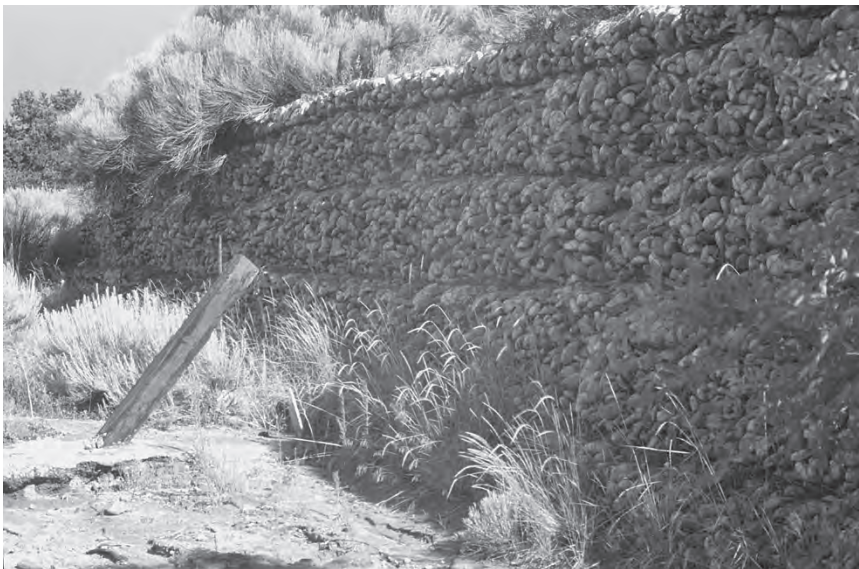
Figure 3.8 Gabions cause fewer problems than impervious walls because they allow water to seep through. Over time or by design, gabions can support vegetation. (Photo: Kim Sorvig.)
