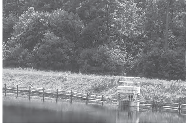
Figure 4.7 The T-shaped opening in this wetland structure sets the water level. Small rises in level flow out through the “trunk” of the T; if major flooding raises the level higher, the top of the T permits faster drainage. (Project and Photo: Rick Scaffidi, EQR.)
