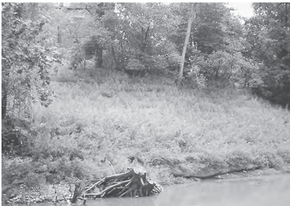
Figure 3.6a–c BTEC techniques form a flexible toolkit, often used in combination, as in stabilizing this bank at Crestwood (Houston TX). Note the large stump, left as added protection, visible in the before, during, and after photos. (Project and Photo: Robbin B. Sotir.)
