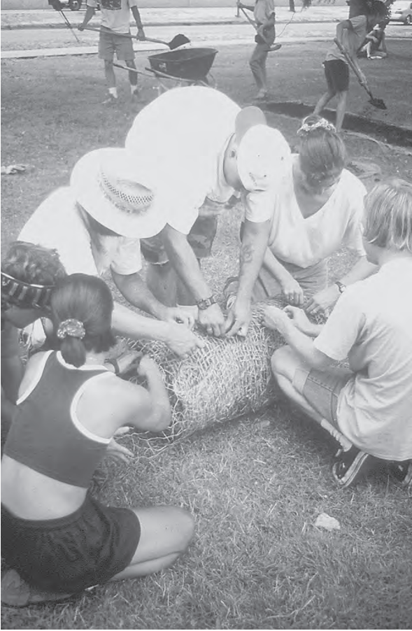
Figure 4.11 University of Oregon landscape students fabricated “soil burritos” of fabric, soil, and chicken-wire for a campus restoration, demonstrating a simple, inexpensive method. (Project and Photo: Professor Stan Jones.)
