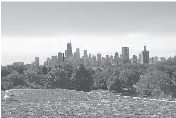
Figure 3.17 Lightweight, “extensive” greenroof covers Peggy Notebaert Nature Museum in Chicago. (Project: Conservation Design Forum. Photo: Andrea Cooper, Conservation Design Forum.)
