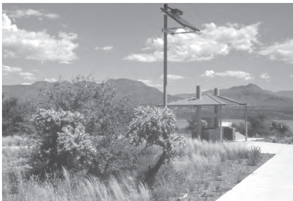
Figure 7.9 Solar electricity for lights and other uses saved hundreds of thousands of dollars in utility installation at Cholla Campground, near Phoenix. Operating costs are near zero. (Project: USFS. Photo: Kim Vander Hoek.)
