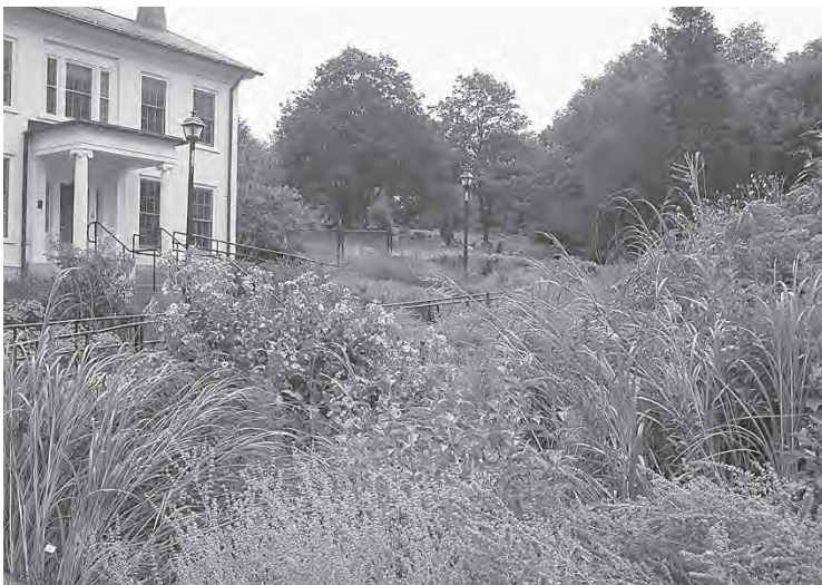
Figure 4.21a–c The Nichols Arboretum (Ann Arbor MI) creates beauty from stormwater management structures. The sequence shows construction and planting of stepped pools to control runoff. ( Project: The Nichols Arboretum. Photo: Robert E. Grese. )
