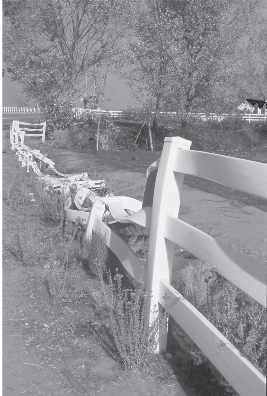
Figure 2.19 In fire-adapted ecosystems, structures must adapt. Plastic fencing melted and the house (right rear) narrowly escaped (San Diego area). (Photo: Kim Sorvig.)
