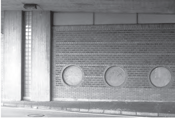
Figure 9.2 Noise walls can incorporate more than concrete, avoiding problems of shadowing and monotony. They are still not terribly effective against noise. (Project: Oslo, Norway; designer unknown. Photo: Kim Sorvig.)
