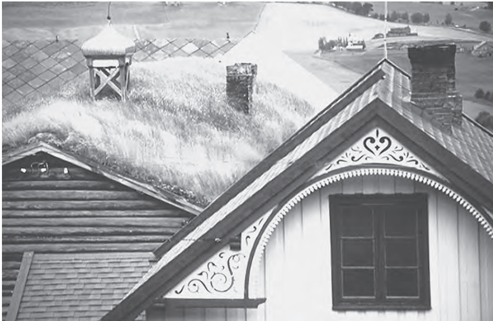
Figure 3.13 Ecoroofs are an update on traditional sod roofs—an example of revisiting past technologies to meet sustainability goals. (Photo: Kim Sorvig.)
