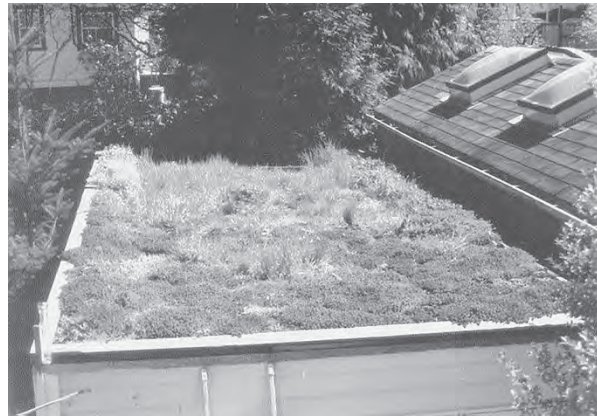
Figure 3.21 Even small-scale ecoroofs decrease runoff, support habitat, and clean the air. Tom Liptan replaced his conventional garage roof with this one. (Project and Photo: Tom Liptan.)
