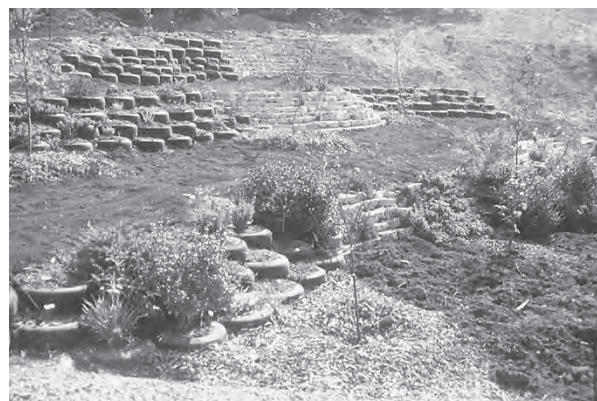
Figure 6.15 Tires and broken concrete achieve unexpected elegance as terraces at the Institute for Regenerative Studies. (Project and Photo: John Lyle.)
