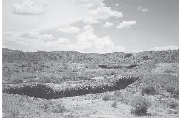
Figure 4.4 More effective than a single massive dam, a series of small check dams stop and infiltrate water throughout a stream or gully. Only the highest floods overflow spillways. (Photo: New Mexico Department of Mining and Minerals.)
