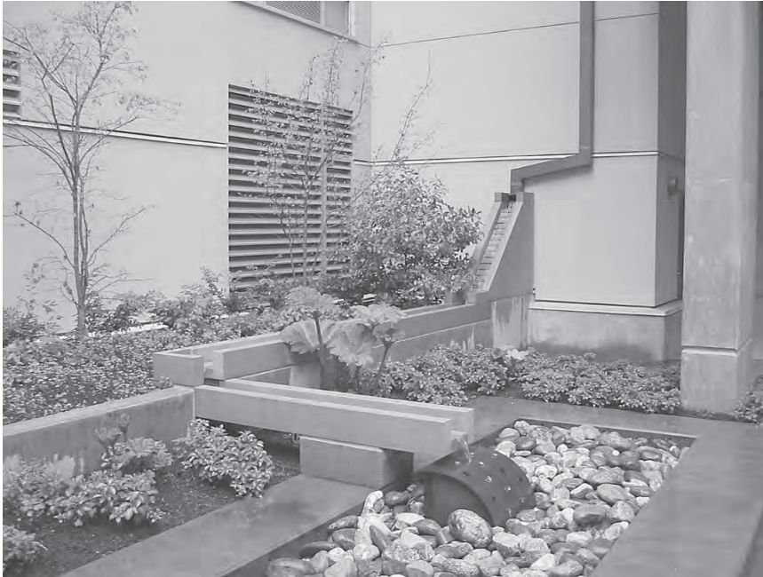
Figure 4.24 The 10th@Hoyt courtyard (Portland OR) makes rainwater visible and artful en route from roof to cistern. (Project: Steve Koch. Photo: Stuart Echols.)
