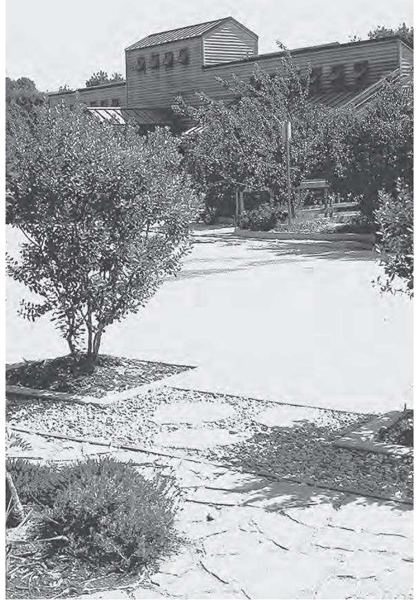
Figure 6.5 Broken concrete, reused in slabs or crushed as aggregate, demonstrates John Lyle's concepts at the Institute for Regenerative Studies. (Project and Photo: John Lyle.)
