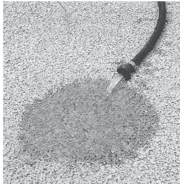
Figure 5.11 Porous concrete, shown here, and porous asphalt support vehicles but permit water to infiltrate rapidly. (Photo: Florida Concrete and Products Association/Dennis Graeber.)
