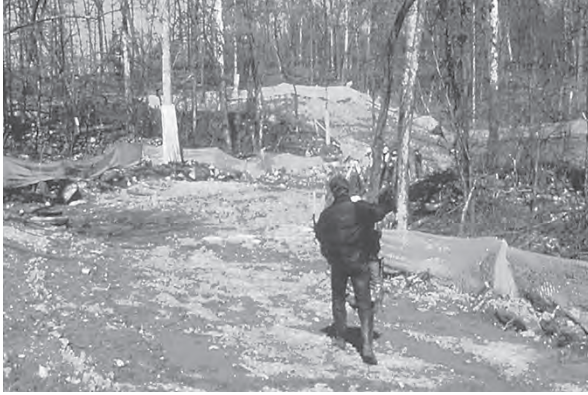
Figure I.8 This easement, in Loudon County VA, is less than half as wide as the utility's standard. Note the site protection fence. (Project: Park Authority, HOH Associates, and Rhodeside and Harwell. Photo: Doug Hays.)
