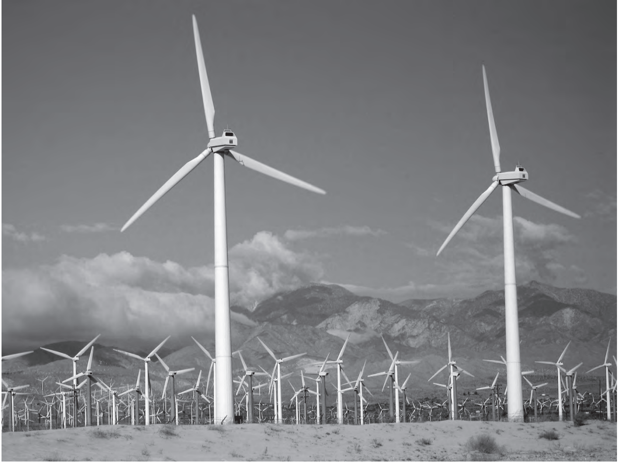
Figure 7.3 This “wind farm” in California is typical of the remote locations where such facilities are being sited, defeating the main advantage of wind (or solar) power, which is on-site, near-the-source generation. (Photo: Winchell Joshua, US Fish and Wildlife Service [public domain], via Wikimedia Commons.)
