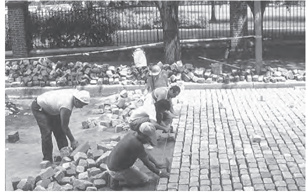
Figure 5.14 Traditional granite setts being laid on sand in Philadelphia’s historic district. Joints are somewhat permeable if not mortared. (Photo: Kim Sorvig.)
