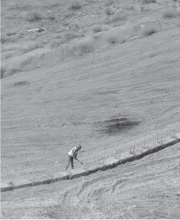
Figure 4.5 Straw bales pinned to the ground provide temporary control of erosion and sedimentation. (Photo: New Mexico Department of Mining and Minerals.)
