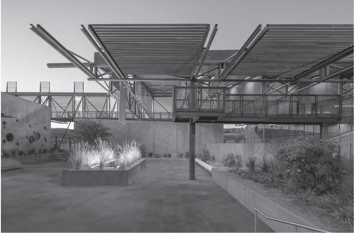
Figure 4.19 Water harvested from roof and landscape is stored for dry-season use at Mariposa Port of Entry, Nogales AZ. A 1-million-gallon tank holds the rainwater. Solar hot water and electricity, as well as recycled materials and native plantings, are other features of this building, one of many commissioned by the General Services Administration. (Project: Chris Winters & Assoc. and Jones Studio. Photo: Bill Timmerman.)
