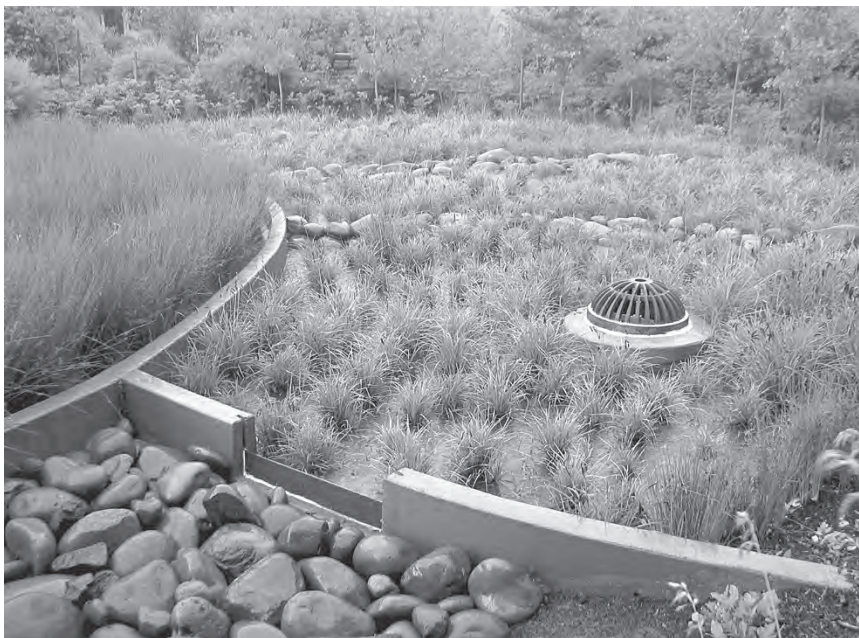
Figure 5.9 This bioswale, part of Glencoe School's green street in Portland OR, uses check dams, a “flash-board” level-setting device in the weir, and overflow drain to treat and infiltrate stormwater. (Project: Portland Bureau of Environmental Services. Photo: Kevin Robert Perry and Portland Bureau of Environmental Services.)
