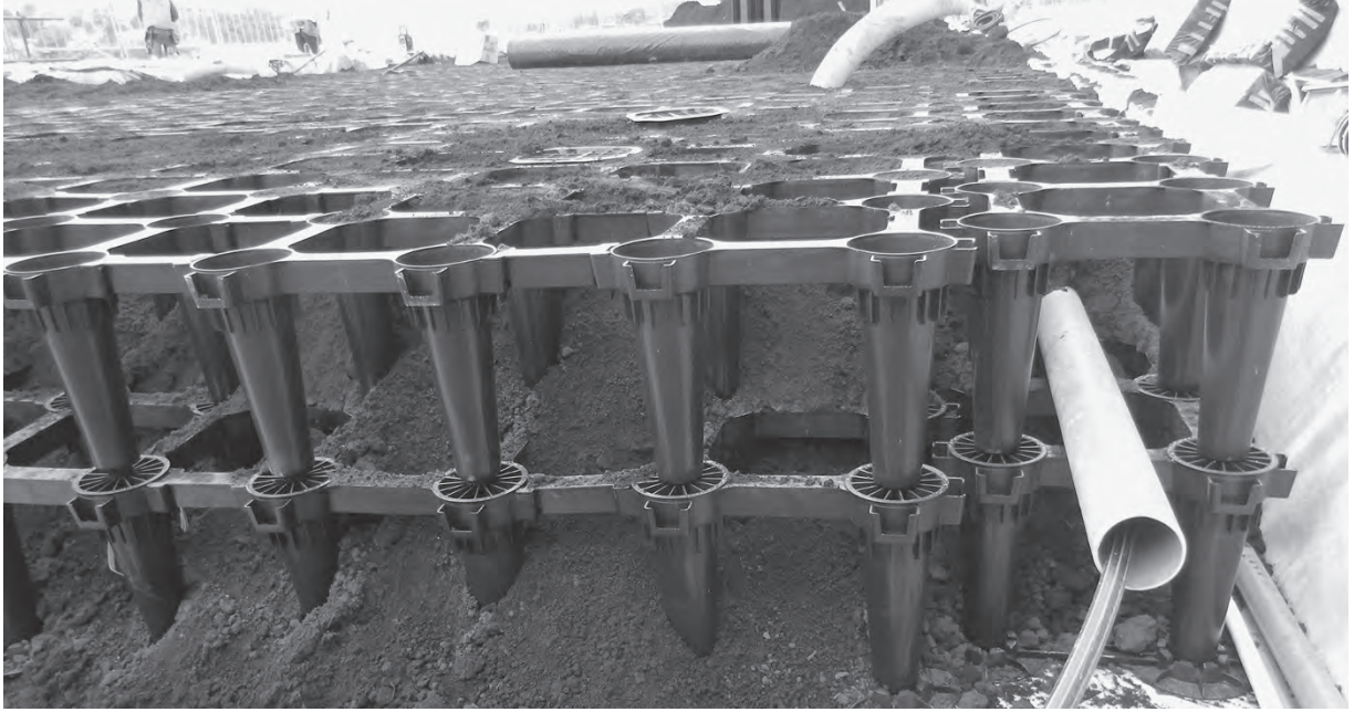
Figure 3.27 “Pits” are created by leaving out cells; the whole trench is backfilled after placing trees, and pavers rest atop the cells. Rectangular Strata Vault system is shown; Silva Cells are similarly shaped. Roots (and utilities) pass easily through such support structures. (Project and Photo: Citygreen.)
