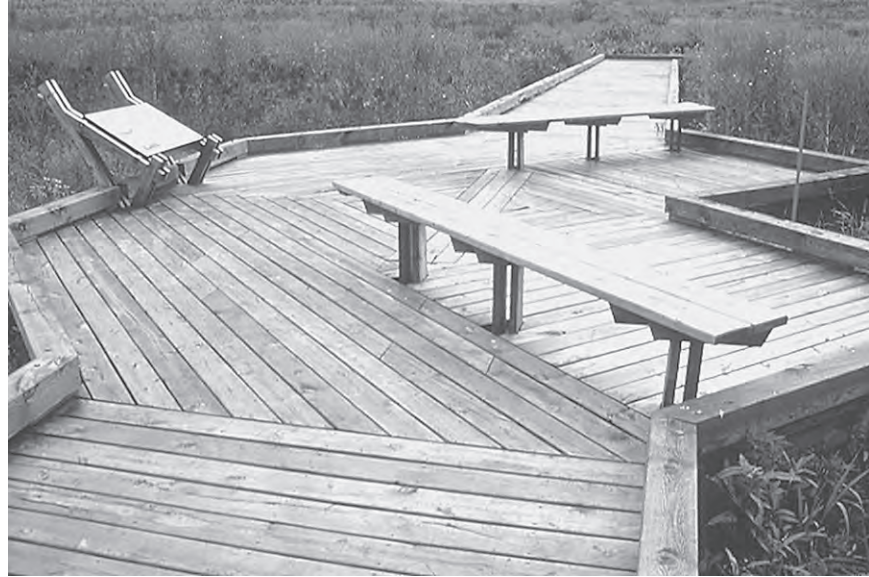
Figure 4.6 Boardwalks can make an art form of the necessity for minimum disturbance in wetlands. This is at Spring Peeper marsh in the Minnesota Arboretum. (Project and Photo: Fred Rozumalski.)
