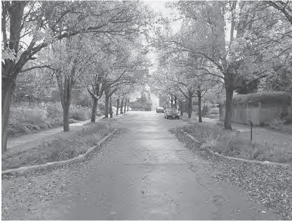
Figure 5.19 “Green streets” (like Siskyou St., Portland OR) collect water from wider areas with parking, and infiltrate it in “bump-out” planted areas that also help traffic calming. (Project: Portland Bureau of Environmental Services. Photo: Kevin Robert Perry and Portland Bureau of Environmental Services.)
