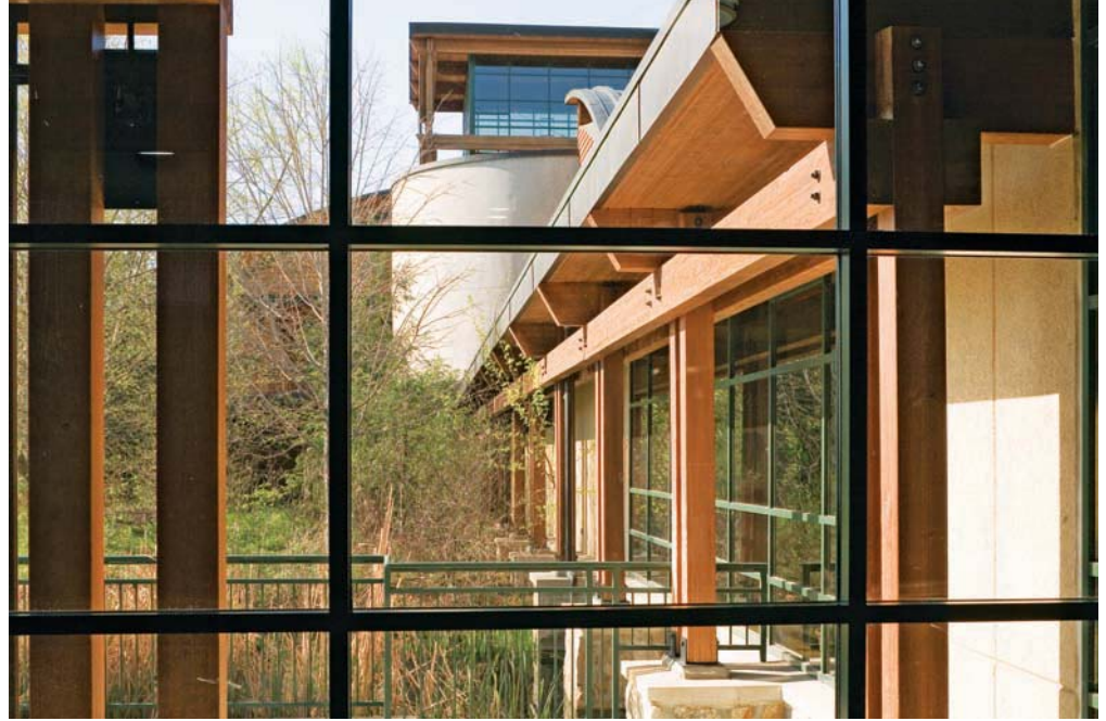
Figure 23-7: Interior View of the Deramus Education Pavilion illustrates the transition between natural and human environments.
