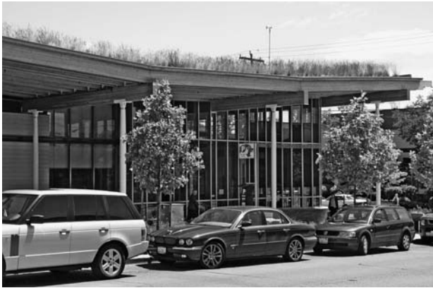
Figure 17-1: Ballard Branch of Seattle Library, Seattle Washington
