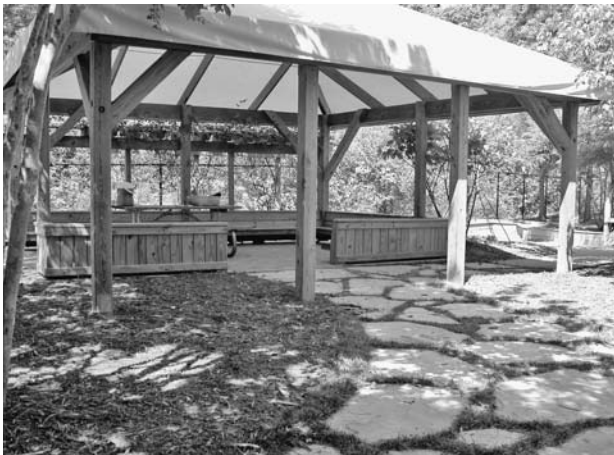
Figure 10-16: A naturalized outdoor classroom can immerse children’s learning processes in nature as well as reduce demands on interior, air-conditioned space. Roof covering is a translucent, waterproof, ultraviolet-light-resistant fabric. As they work, children can enjoy the experience of rain pouring down around them or the play of sunlight and shadow of foliage vibrating in the wind over their heads.
