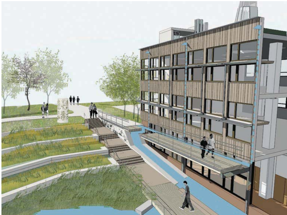
Figure 4-16: Storm water is led to overhanging fixtures at the roof edge, which guide the water to open downspouts. The water is collected in an open channel paralleling a walkway, then guided to a constructed on-site wetland. Sidwell Friends Middle School, Washington, DC.
