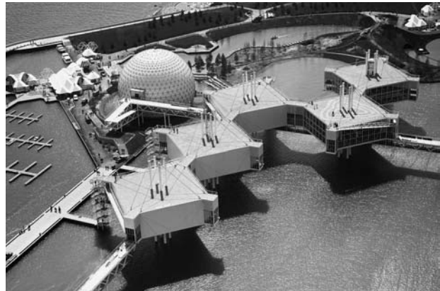
Figure 4-20: Pods holding the theater, restaurants, and other visitor attractions, cantilevered over the water at Ontario Place, a cultural, leisure and entertainment parkland in Toronto, Ontario, Canada.
