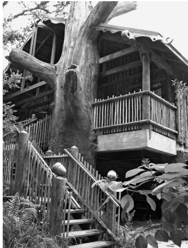
Figure 10-30: Classrooms in the trees at Brevard Zoo, Melbourne, Florida, enable the curriculum for at-risk fifth-graders to be conducted at the zoo. (See www.brevardzoo.org/education/zoo_school .)
