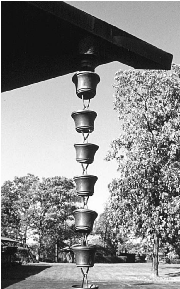
Figure 4-17: Residential gutters lead, not to enclosed downspouts, but to rain chains that conduct the water to ground level, creating animation and music on the way.
