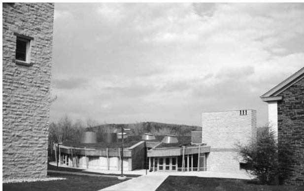
Figure 14-15: View of planted roof on dining hall
