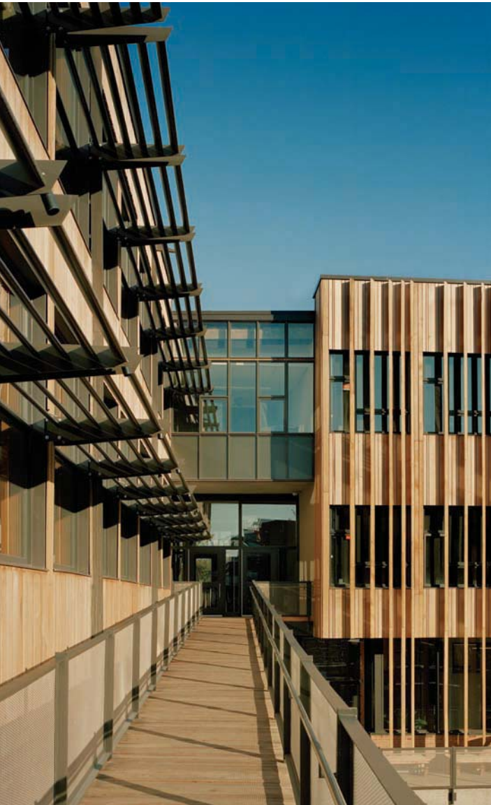
Figure 14-4: Vertical and horizontal sunscreens, Sidwell Friends Middle School
