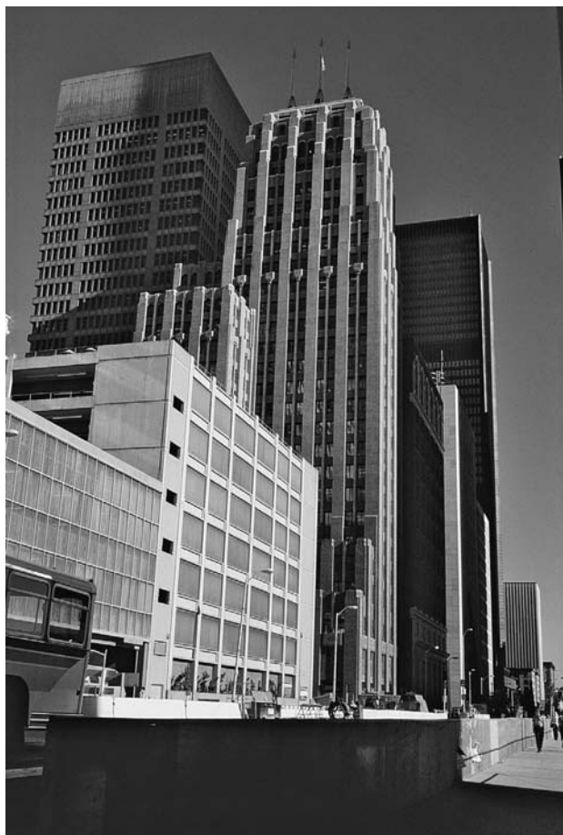
Figure 16-11: The Northern Life (now Seattle) Tower, Seattle, Washington
