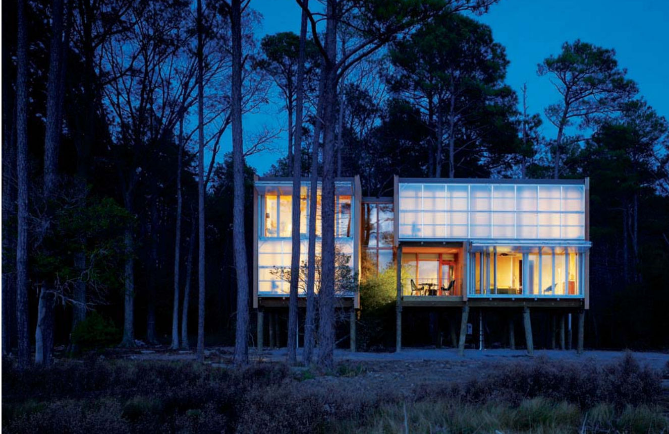
Figure 14-10: View of Loblolly House from the west
