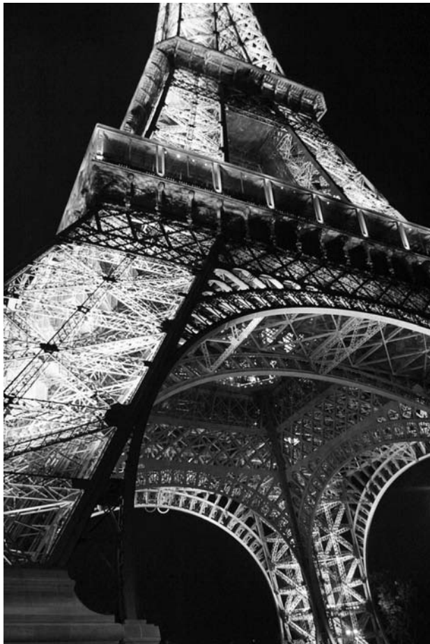
Figures 3-4a and 3-4b: The lower curve of the Eiffel Tower is based on the human femur or thigh bone, where it curves to join the hip. Both femur and tower base must accommodate off-center stresses.
