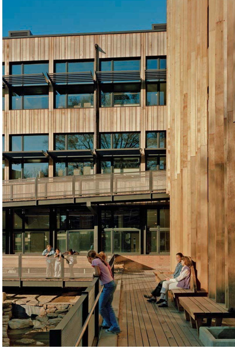
Figure 14-5: Unified multilayer skin at Sidwell made from reclaimed fermentation barrels
