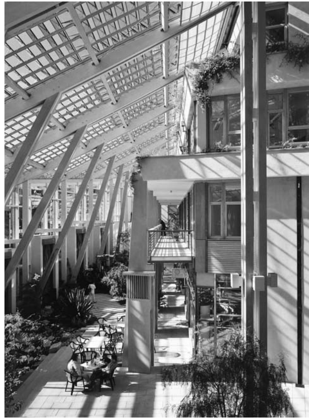
Figure 4-15: Rainfall is processed through small wetlands on the building shell, to an interior pool, then to a cistern beneath the building and an exterior pond. The water then supplies on-site greenhouses. Interior waterfalls create sound and cool the air in summer. Prisma, Nuremberg, Germany.
