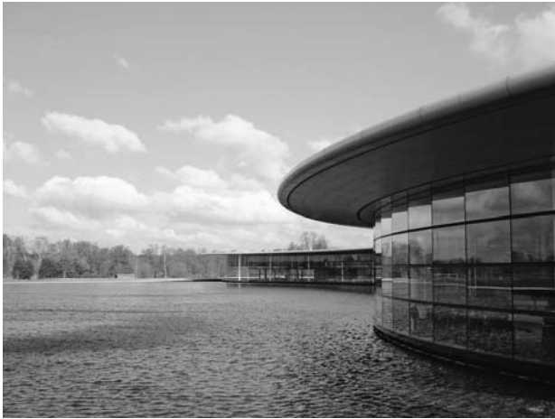
Figure 4-10: Standing water adjacent to an office complex blurs the boundaries between inside and outside. McLaren Technology Centre Research Centre, London.
