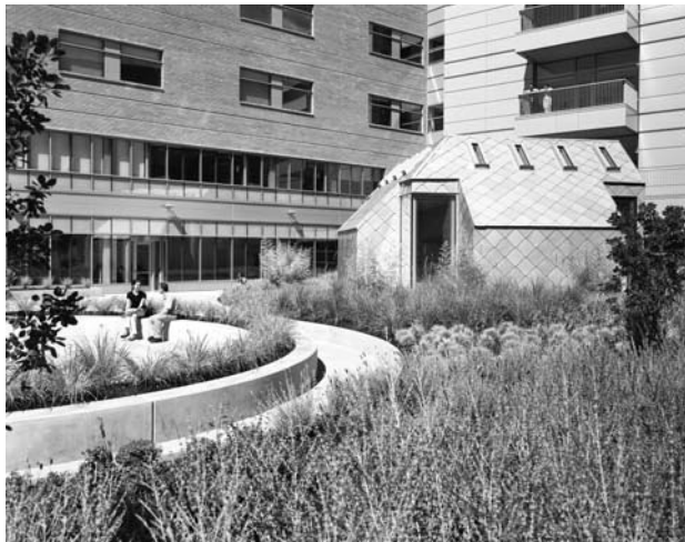
Figure 6-9: Hospital rooftop garden at Legacy Health, Salmon Creek, Washington. The garden enables users to be exposed to sun and engage in sedentary restorative activities such as viewing distant hills and forests. A meditation room juts into the garden (right center). The garden provides restorative garden window views for bedridden patients, and the berm prevents persons in the garden from looking into patient rooms and violating privacy (patient rooms are out of picture to right).
