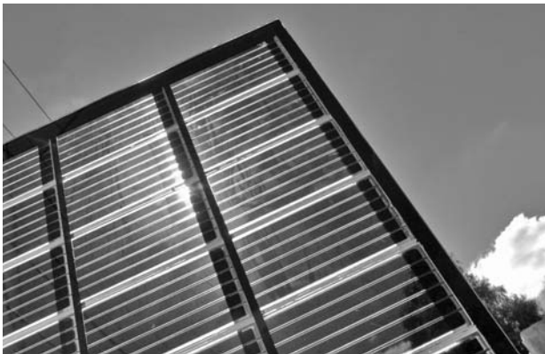
Figure 3-3a: The principles of photosynthesis have been mimicked in dye-sensitized solar cells. These low-cost cells, made from benign materials, can be fashioned into windows, roof tiles, and façade panels, giving the Commonwealth Scientific & Industrial Research Organization (CSIRO) building in Australia the ability to gather its own energy.
