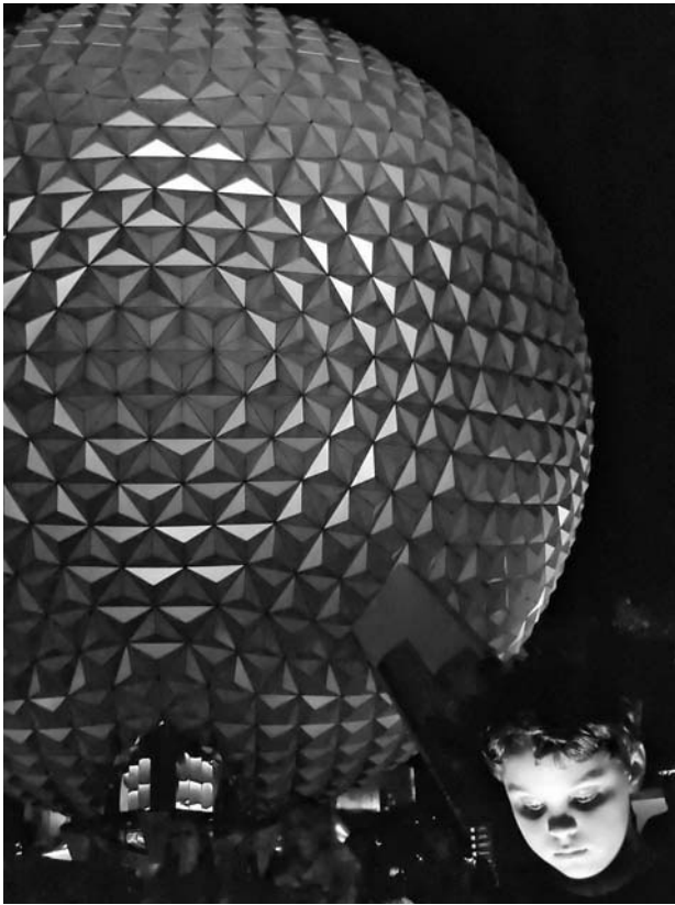
Figures 3-5a and 3-5b: Buckminster Fuller's geodesic domes (like the Epcot Center dome pictured here) incorporate structural principles found in nature at many scales, from the C_{60} molecule to the skeletons of radiolarians.
