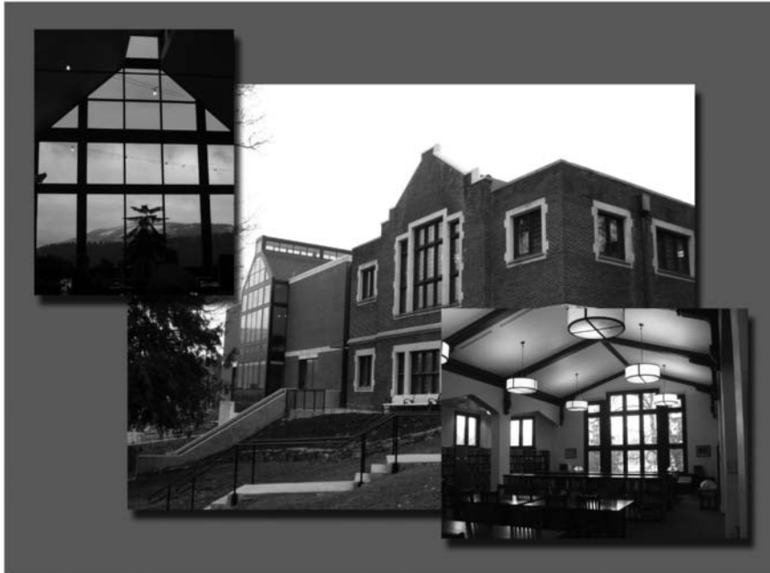
Photo 2.3 The Hood River County Library. The old library is on the right-hand side of the exterior (view taken from the south). Notice the large percentage of window-to-wall area on both buildings. The new addition has high walls set with operable windows that draw air from lower openings, creating a convective flow of outside air through the building when ventilation and cooling are needed. The photo insets capture the interior to exterior view from the old and new spaces (Ken Baker).
