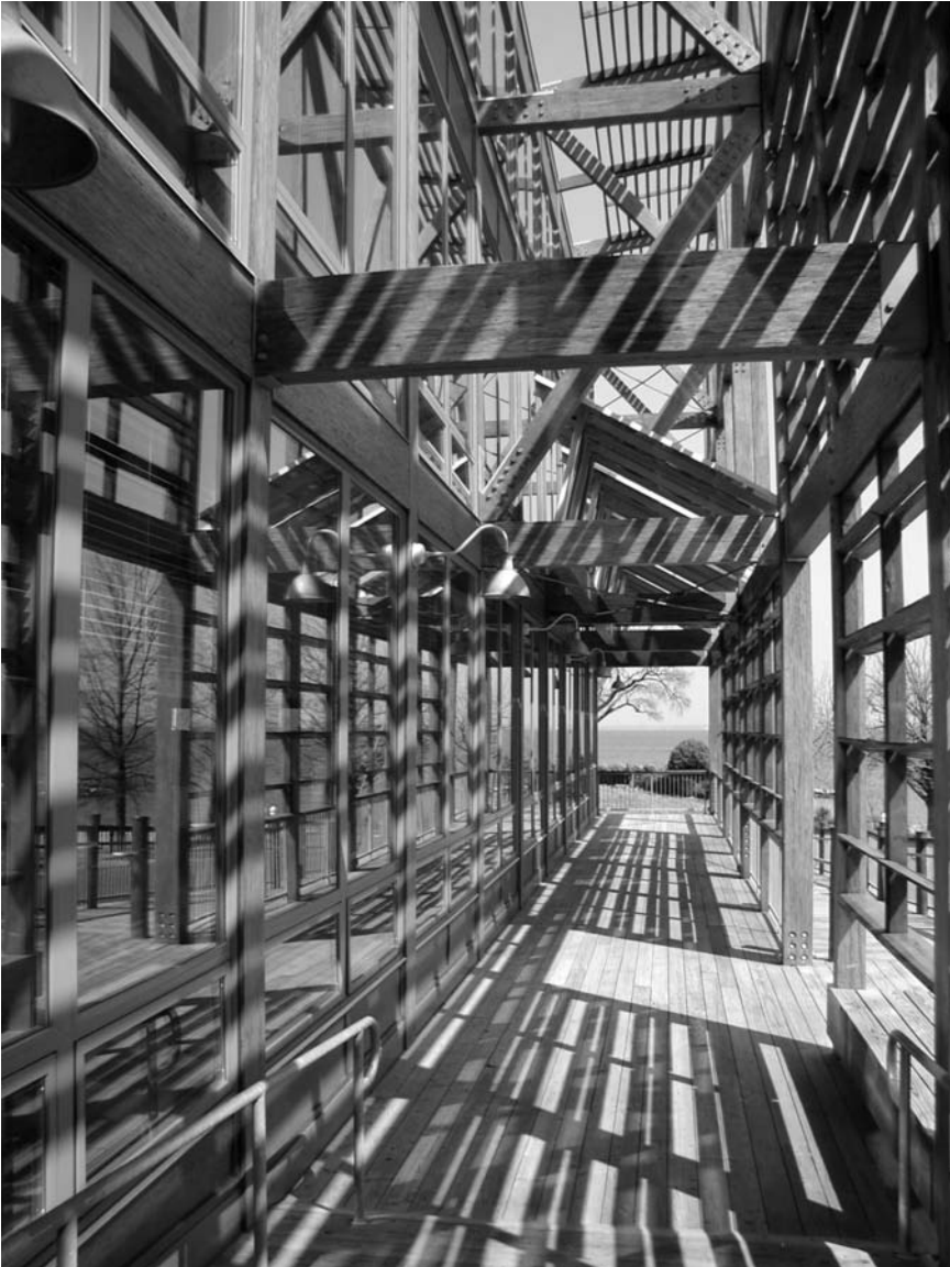
Photo 6.2 Philip Merrill building, exterior deck. This deck and structure serves several functions. It provides shade for the interior building and for people using the deck, serves as a support structure for photovoltaic panels that supply power to the building, and adds to the architectural and aesthetic interest of the building (Dr. Joel Loveland).
