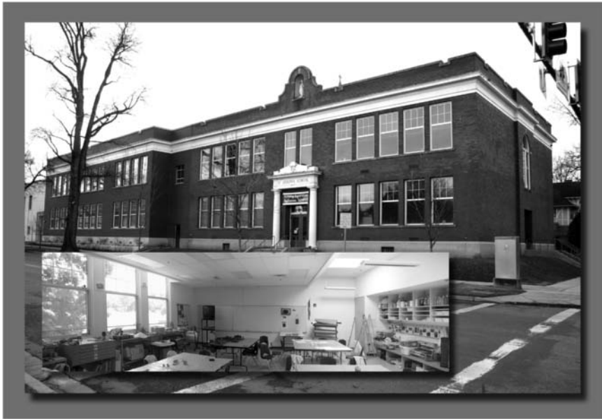
Photo 1.2 Daylighting—blending old and new. St. Joseph's Elementary school in Boise, Idaho, is an example of an early 1900s building with windows restored to full daylighting benefit. In contrast to the school shown in Photo 1.1, these windows are being used per original design, for bringing natural light into the classroom. Note the photo of the interior classroom space and the addition of a set of skylights to the back of the classroom. This is a recently added feature (designed by InSight Architecture, Boise, Idaho) and shows how modern and old design can integrate with great compatibility and purpose (Ken Baker).
