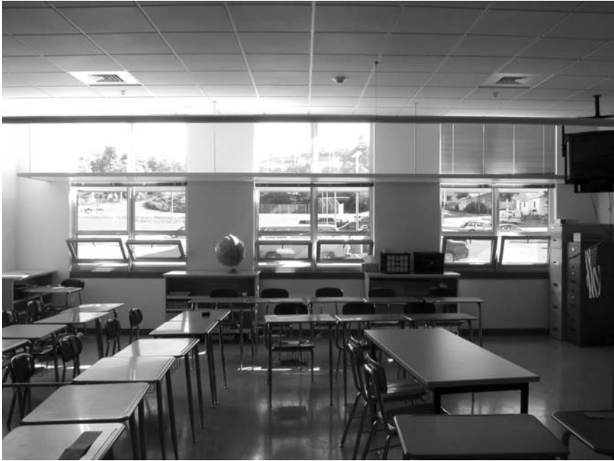
Photo 2.1 Daylight harvesting strategies, Dalles Middle School, Dalles, Oregon, Boora Architects. An interior light shelf in the classroom shown here has two main functions: First, it eliminates glare by reflecting light from the upper window onto the ceiling, spreading the luminance over a larger area of the room and thus diminishing the contrast in light levels between the interior space and the window wall. Second, it brings natural light deeper into the building space, providing more occupants with natural light and reducing the need for electric lighting (Kevin Van Den Wymelenberg).
