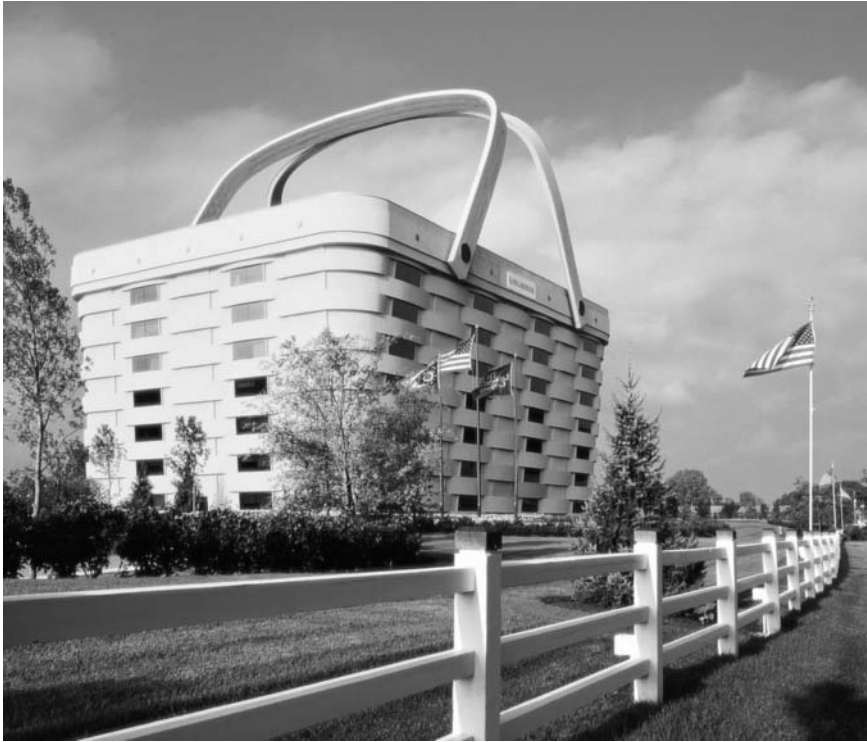
Photo 3.1 The Longaberger Home Office is a seven-story building that replicates the company's trademarked Longaberger Basket (The Longaberger Company).
