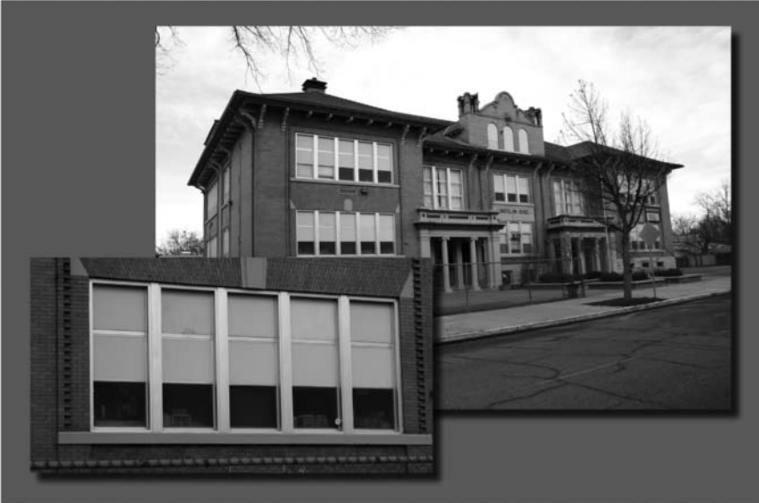
Photo 1.1 Window energy efficiency measures (Ken Baker).
