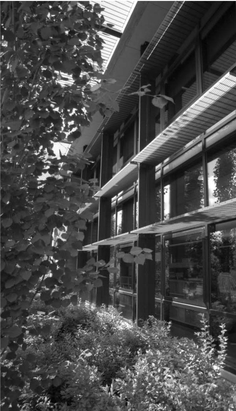
Photo 2.2 Exterior building shading strategies, Pierce County, Washington, Public Safety building, Miller Hull Architects. Depending on a building's orientation and size and location of windows in the exterior building wall, good exterior shading devices (or overhangs) like the one shown here can help to eliminate unwanted solar gain and glare. Notice also that exterior vegetation provides natural shading (Kevin Van Den Wymelenberg).
