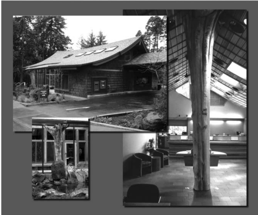
Photo 2.5 The Bank of Astoria, Manzanita, Oregon, Tom Bender, architect. The exterior views are taken from the west. In the background photo, note the slope of the roof's ridge. Natural roofing material is designed to grow moss. The bottom left inset highlights the columnar tree trunk that supports the roof's drainage pan. The interior photo captures the beauty of form and textures highlighted by natural daylighting. Windows provide a close view of trees and the street. The changing light conditions by day create connections for people to the outdoors (Tom Bender and Ken Baker).
