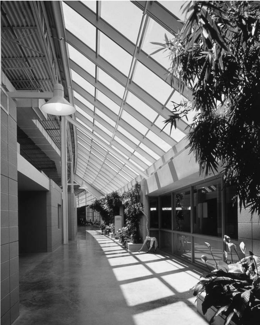
Photo 6.1 Herman Miller Greenhouse, Interior Street, William McDonough + Partners. The interior street became a key design element for increasing workplace satisfaction among occupants. This plant-filled walkway allows employees to access different areas of the factory and provides both natural light and views for the workers, as well as a pleasant space in which to socialize in a summer-like environment during the cold Michigan winters (The Herman Miller Company).
